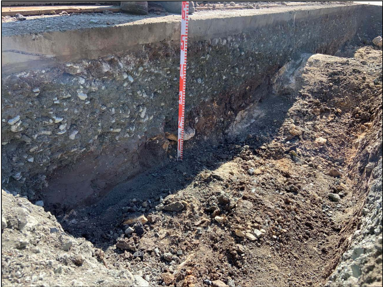
Figure 33. Photograph of T-3 northeast sidewall, view to east
