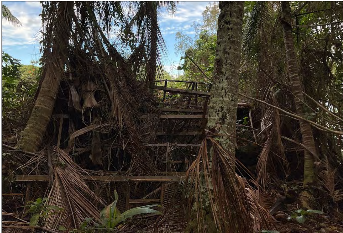
Figure 19. Old metal bleachers along the cliff edge portion of the project area, view to the northwest.
