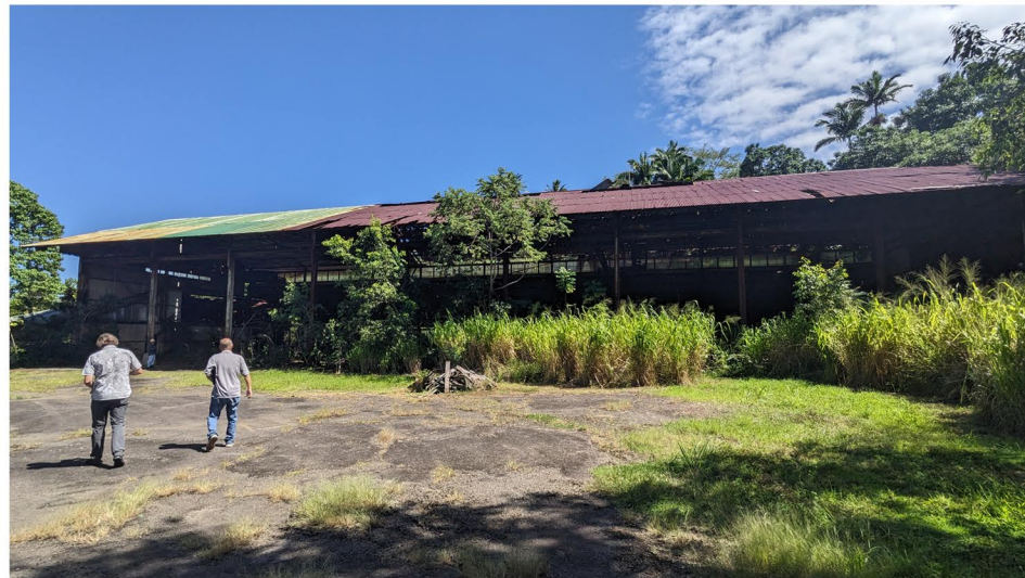
7. Former Laupāhoehoe Shop Building in Lower Park Area
