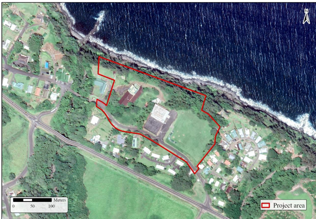
Figure 49. 2021 Google Earth aerial image showing project area, note land use activities in the western portion of the project area.
