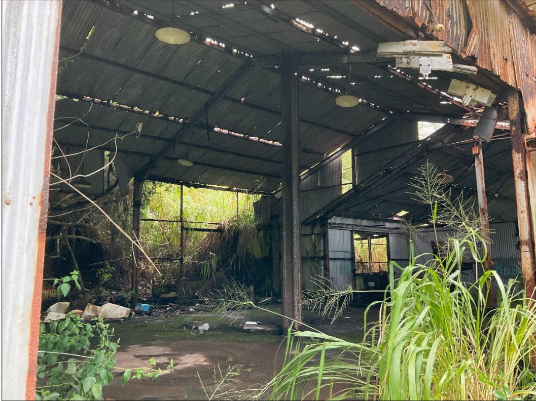
Figure 62. Feature A, interior of large garage, view to the south.
