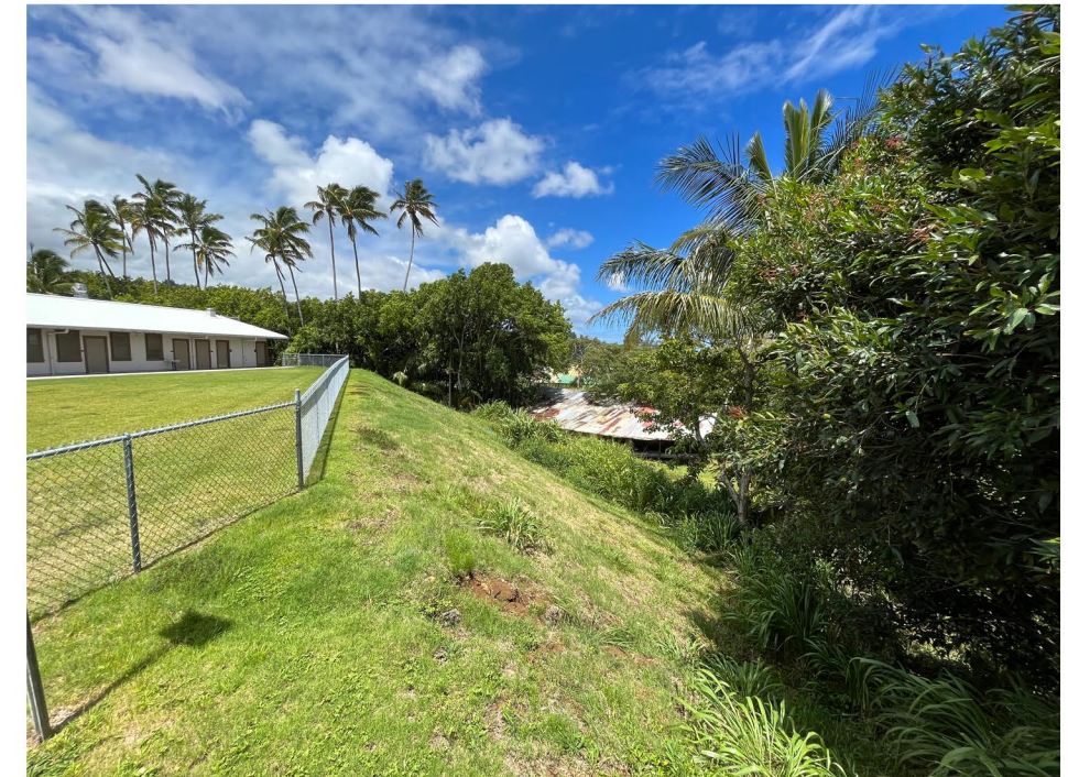
9. Slope Behind Former Gym Site Towards Former Shop Building
