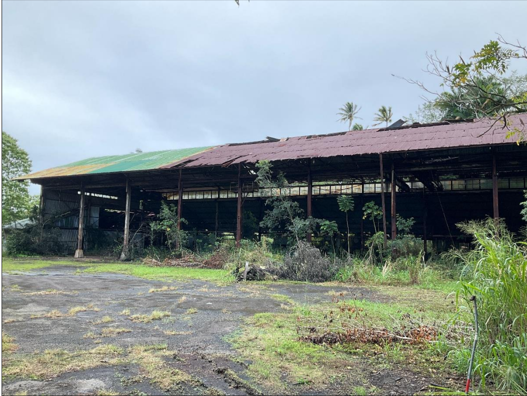
Figure 60. Feature A, large garage, view to the east.
