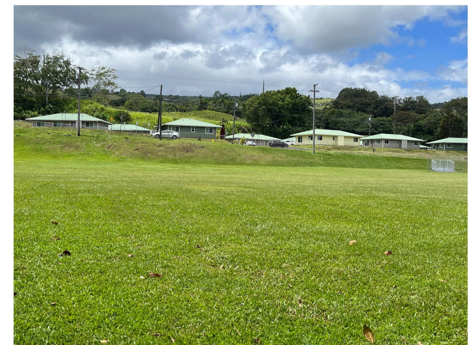
12. View of Embankment Along Skill Camp Road
