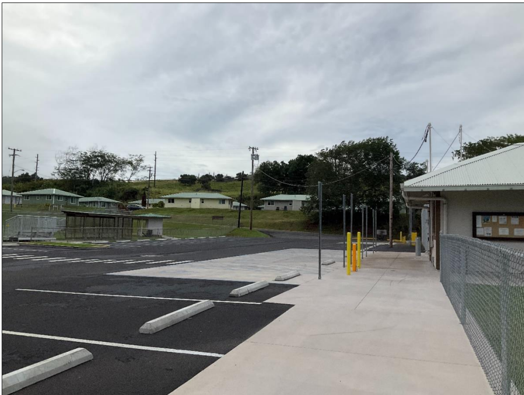
Figure 8. Asphalt paved parking lot located between grassy sports field and annex building and tennis/pickleball courts, view to the southeast.
