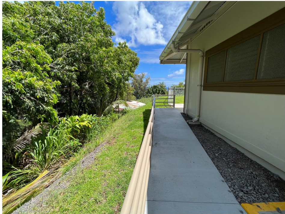
5. Slope Behind Annex Building to Lower Area
