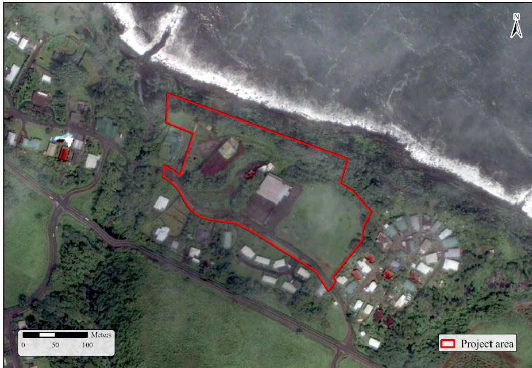
Figure 50. 2014 Google Earth aerial image showing project area, note land use activities in the western portion of the project area.
