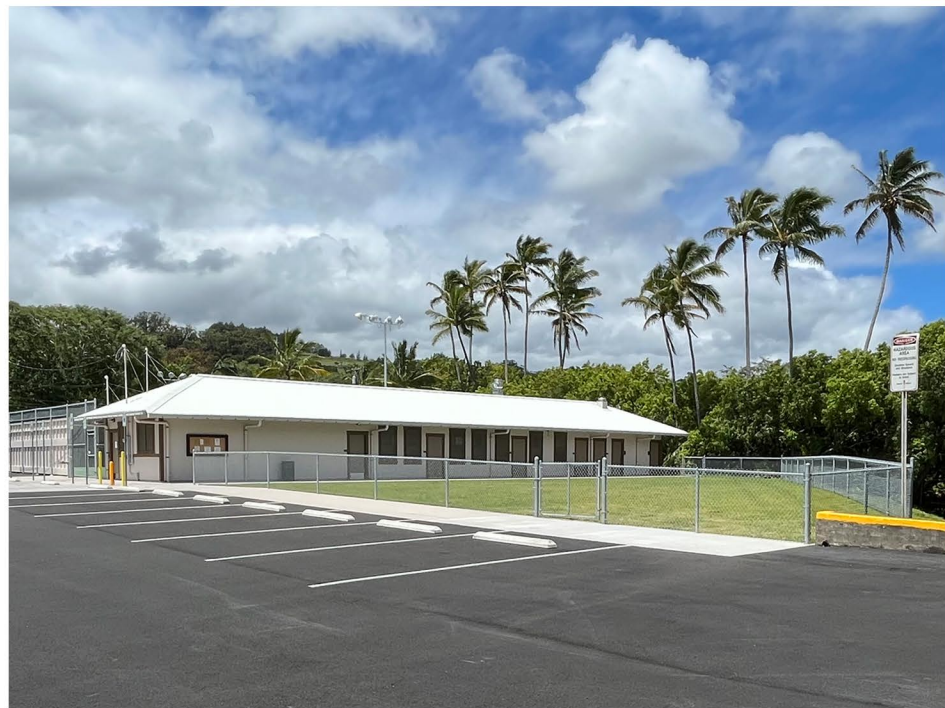
10. Annex Building from Northeastern End of Parking Lot
