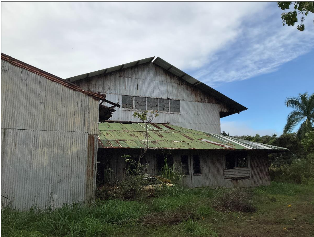
Figure 61. Feature A, large garage, view to the southwest.
