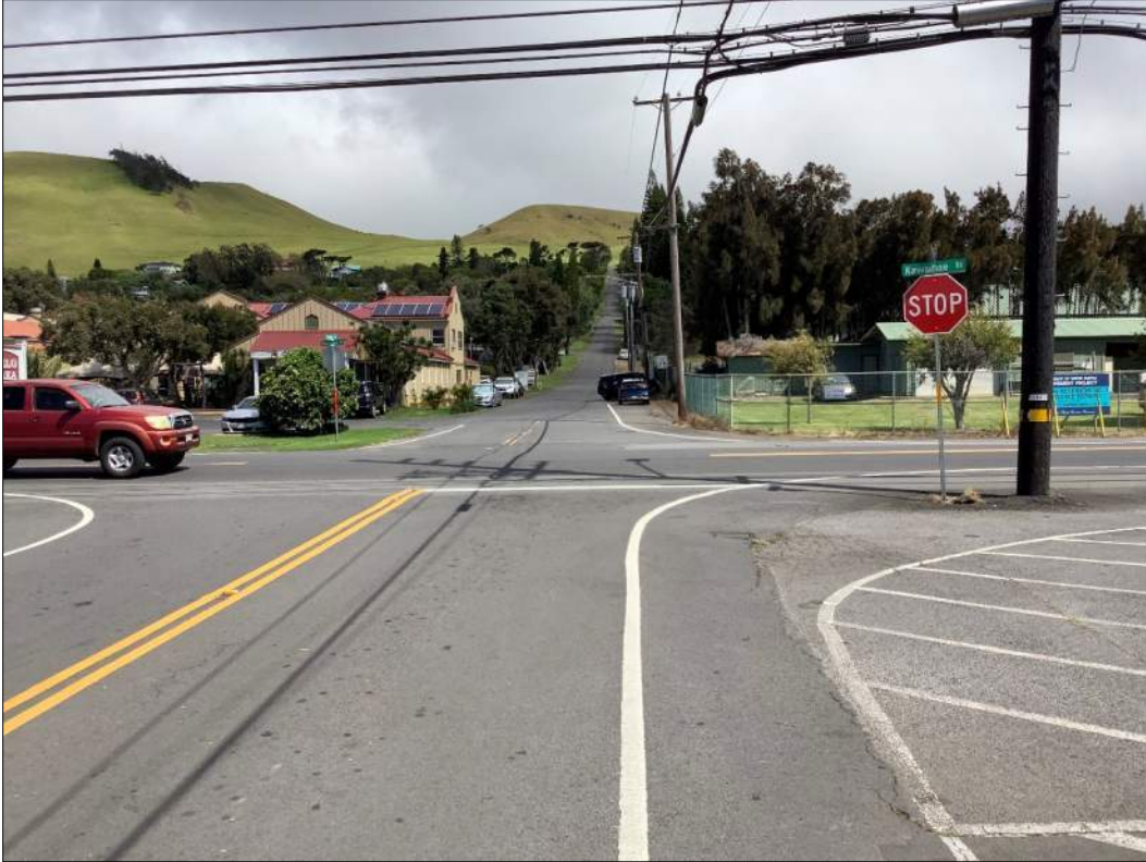
Figure 16. Kawaihae Road-Opelo Road intersection, view to the north.
