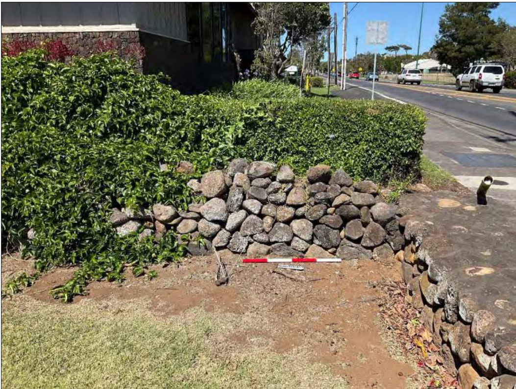
Figure 58. Site 31347 rock wall on western parcel boundary, view to the west.
