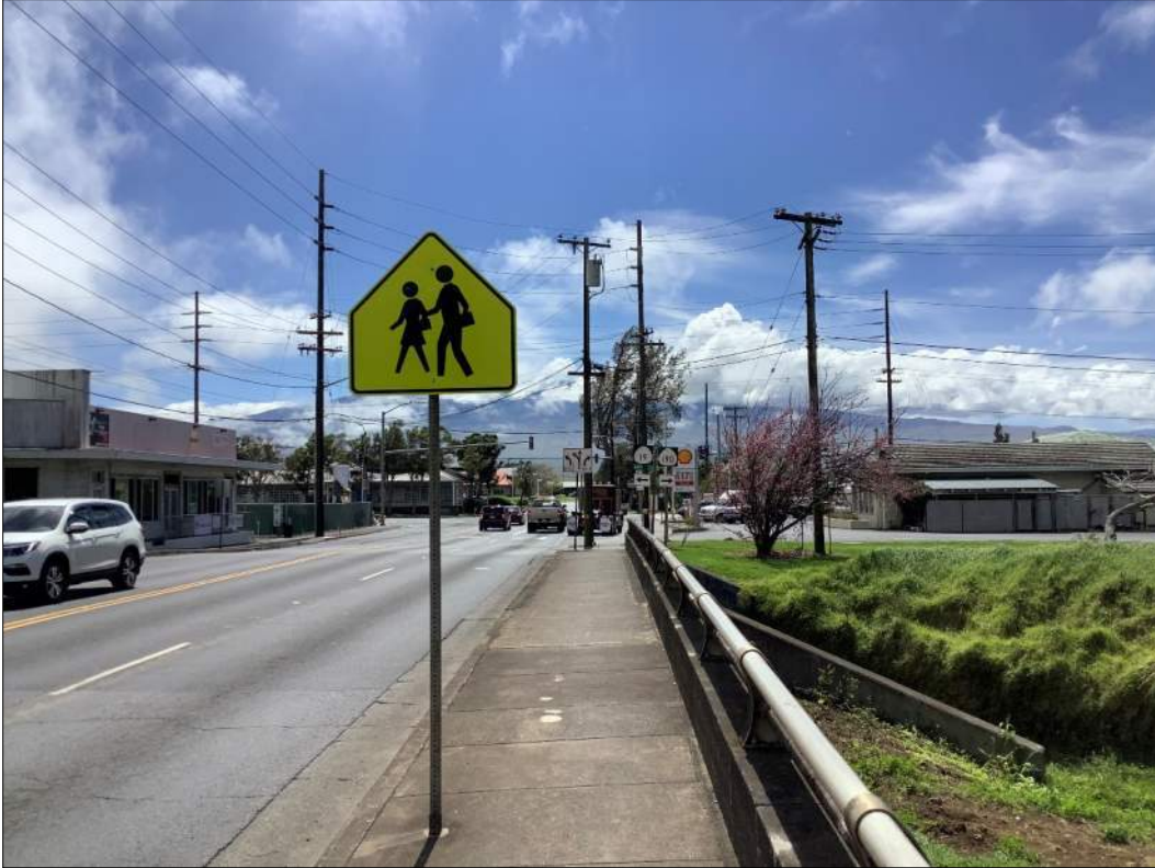
Figure 12. Lindsey Road at the Waikōloa Stream bridge with Lindsey Road-Māmalahoa Highway intersection in the background, view to the southeast.
