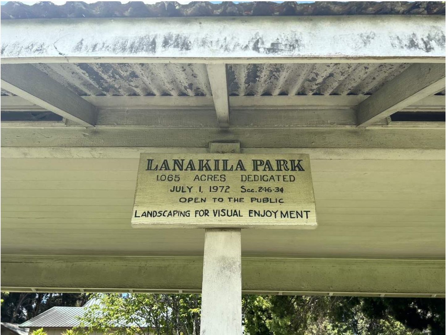
Photo 9: Lanakila Park sign, located under roof eave on southeast elevation.
