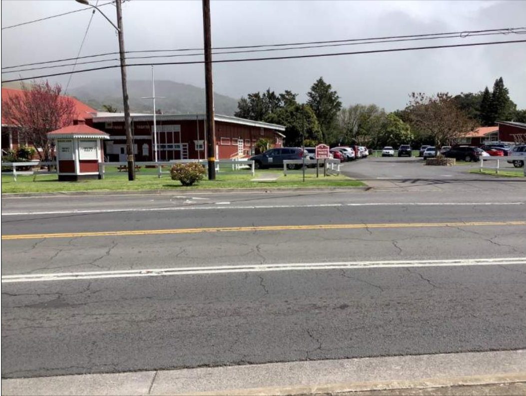
Figure 13. Lindsey Road, view northeast toward Parker School.
