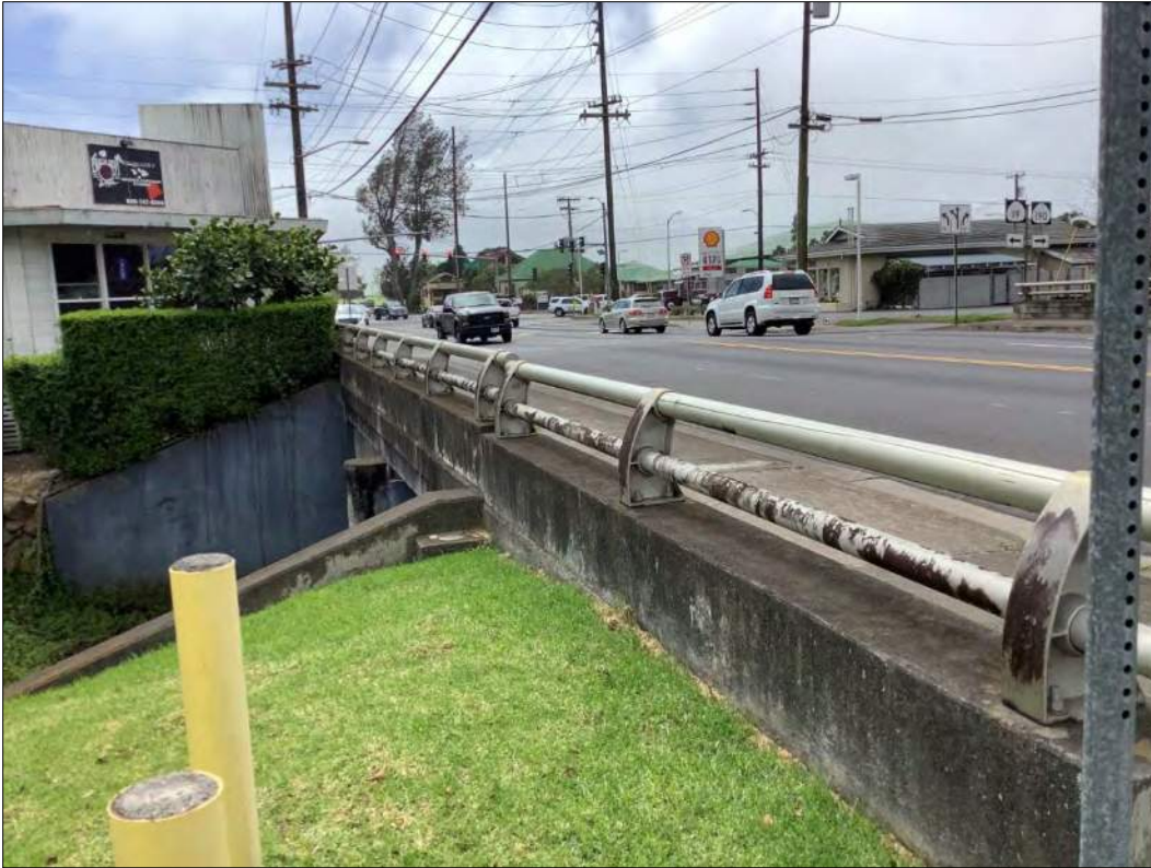
Figure 23. Waikoloa Bridge, view to the south.
