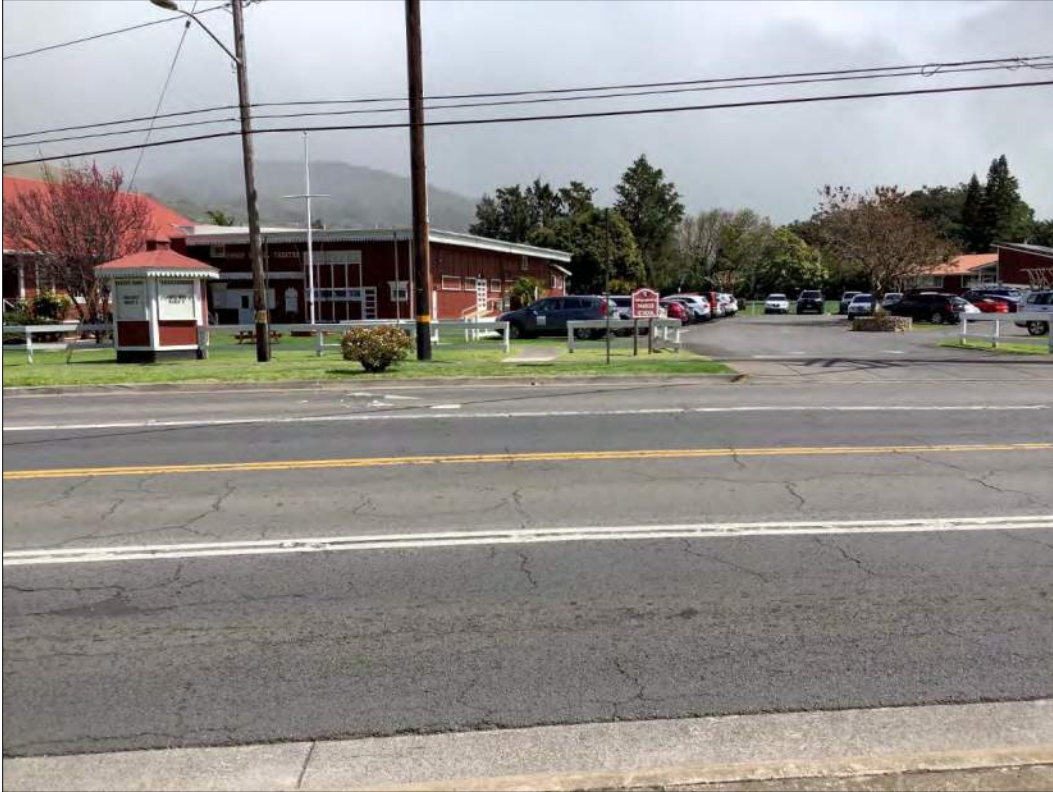
Figure 13. Lindsey Road, view northeast toward Parker School.
