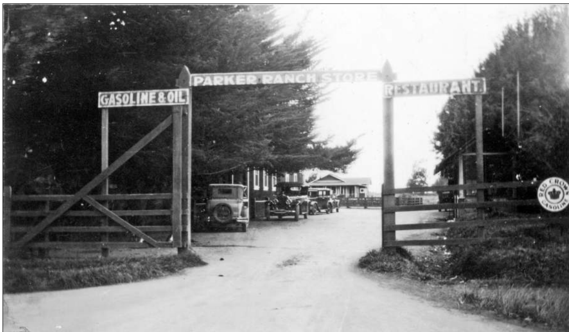
Figure 29. Entrance to the former Parker Ranch store and restaurant ca. the 1930s (photo courtesy of the Kō Education Center, Honoka'a).
