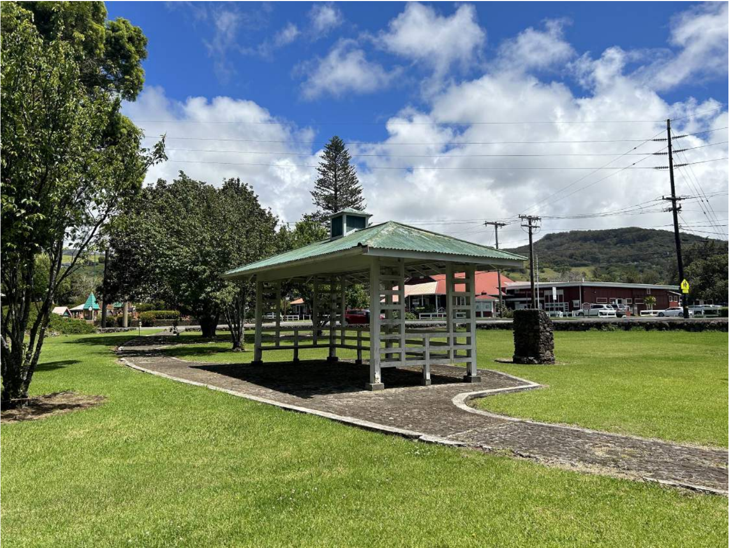
Photo 6: Corner of rear (southwest) elevation and southeast elevation of gazebo.
