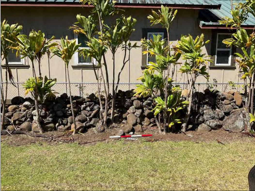
Figure 57. Site 31347 rock wall on western parcel boundary, view to the west.
