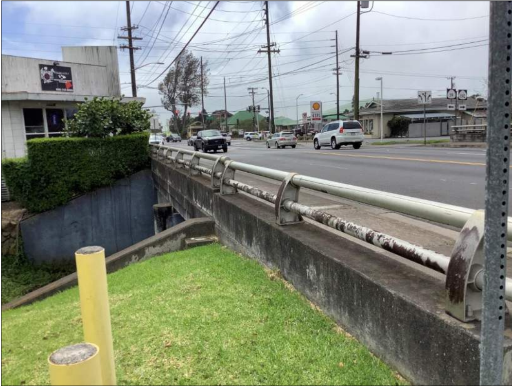
Figure 23. Waikoloa Bridge, view to the south.
