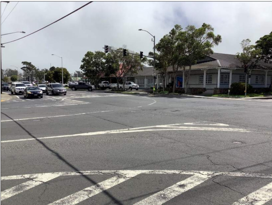
Figure 13. Lindsey Road-Māmalahoa Highway intersection, view to the east.
