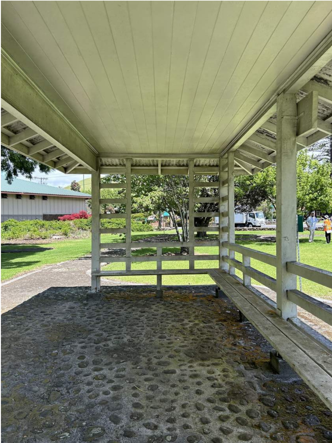
Photo 8: Interior of gazebo, looking toward northwest interior elevation.
