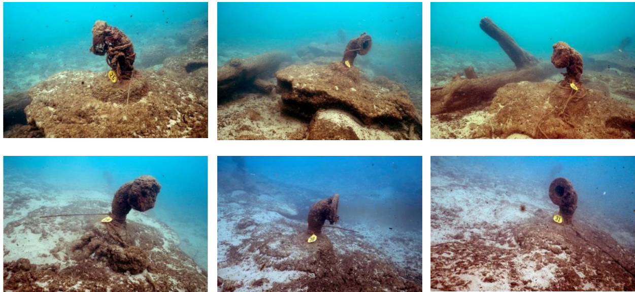
Figure 2-5: Existing Wailua WWTP Ocean Outfall Diffusers
