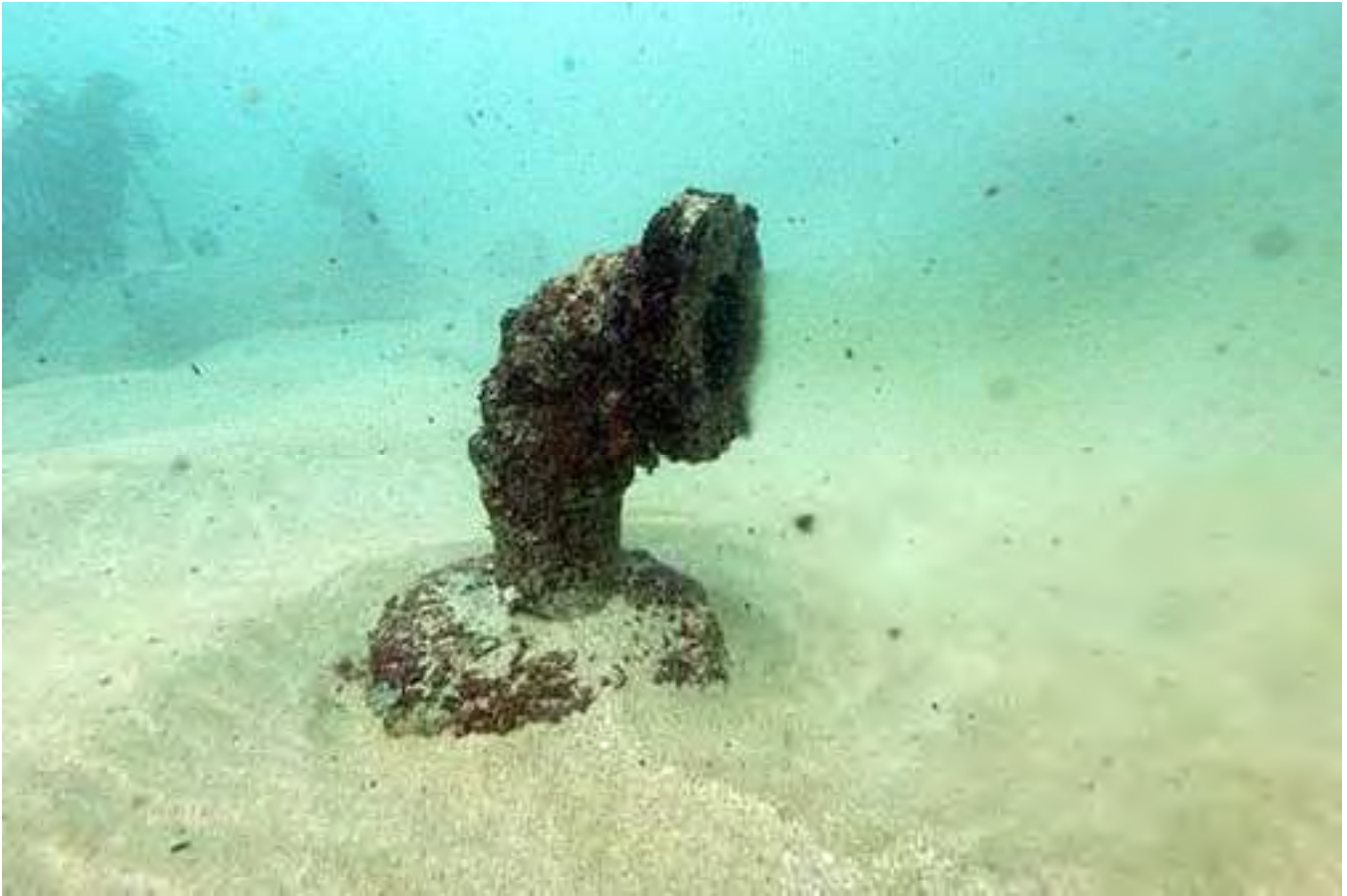
FIGURE 2. Photographs of two Wailua Wastewater Treatment Plant ocean diffuser ports discharging effluent taken on December 23, 2016. Second port can be seen faintly in the background. Note difference in sand cover around ports between Figures 4 (2012) and 3-4 (2016).
