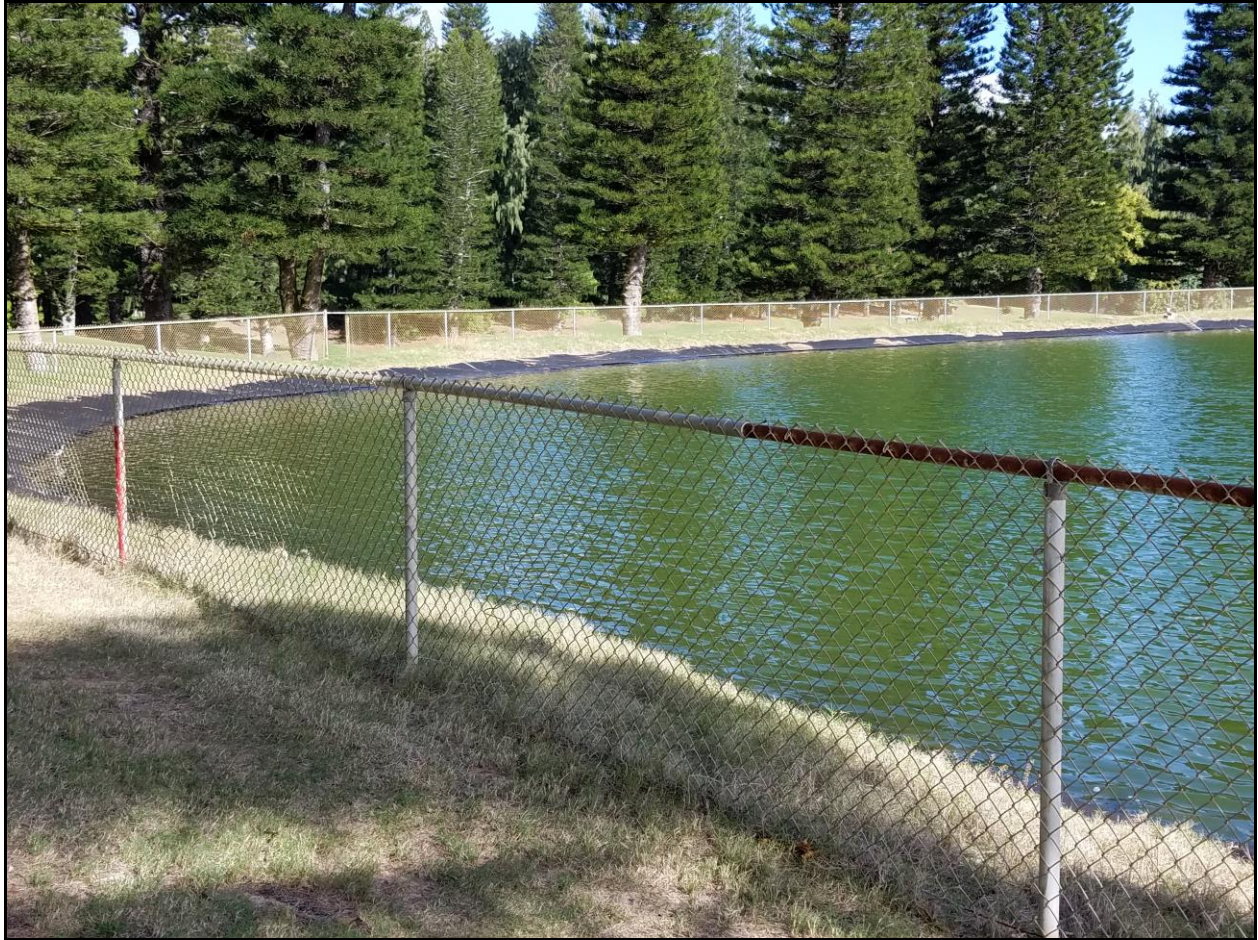
Figure 3-1: Irrigation Holding Pond
