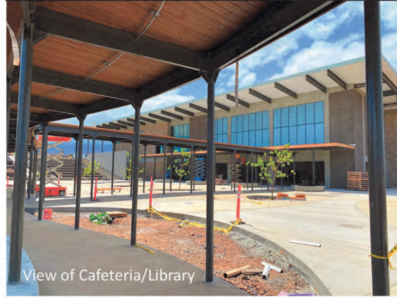
Photo Credit: Nordic PCL Construction
