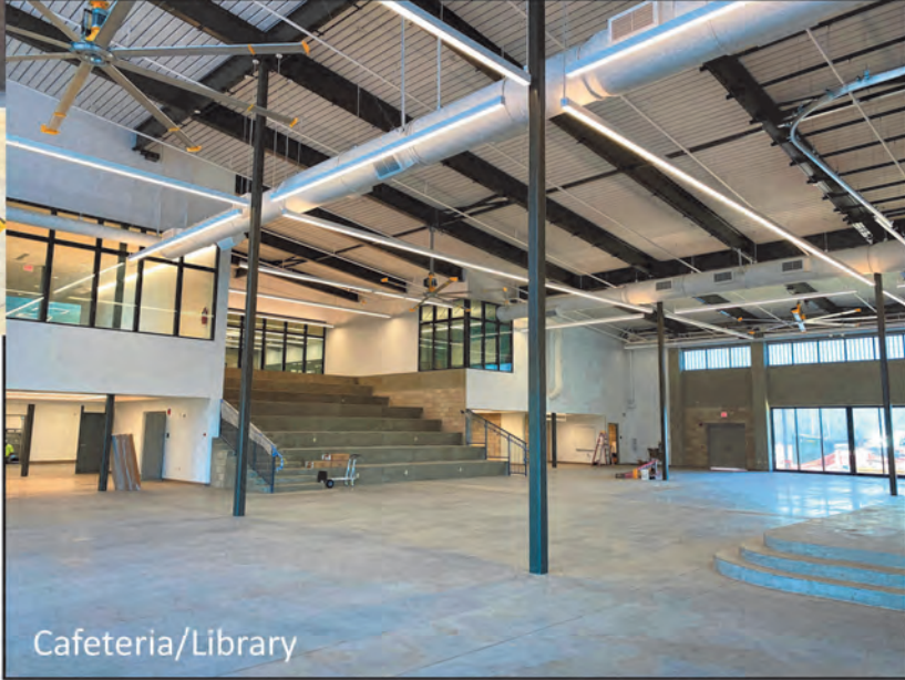
Photo Credit: Nordic PCL Construction
