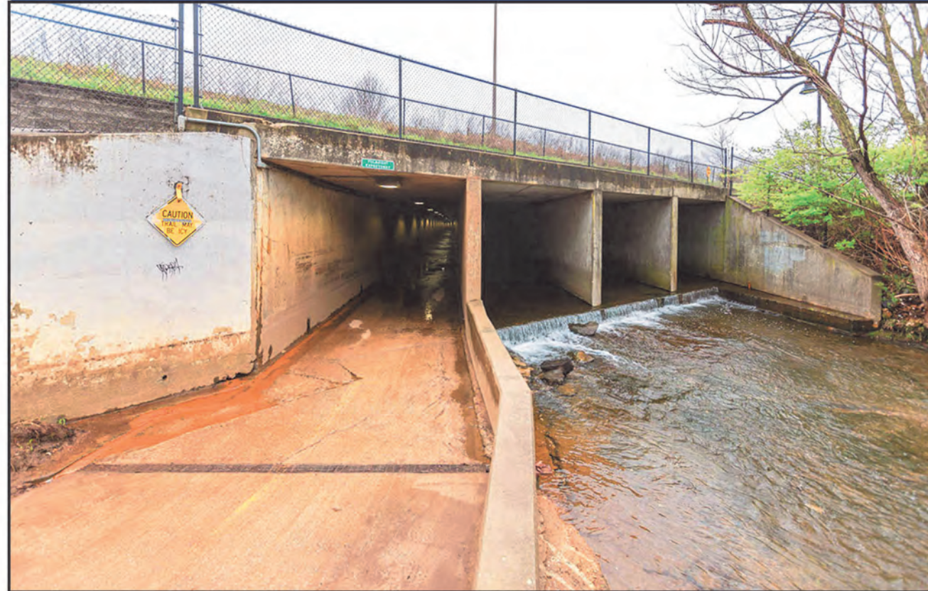
Tunnel under Existing Bridge Example
