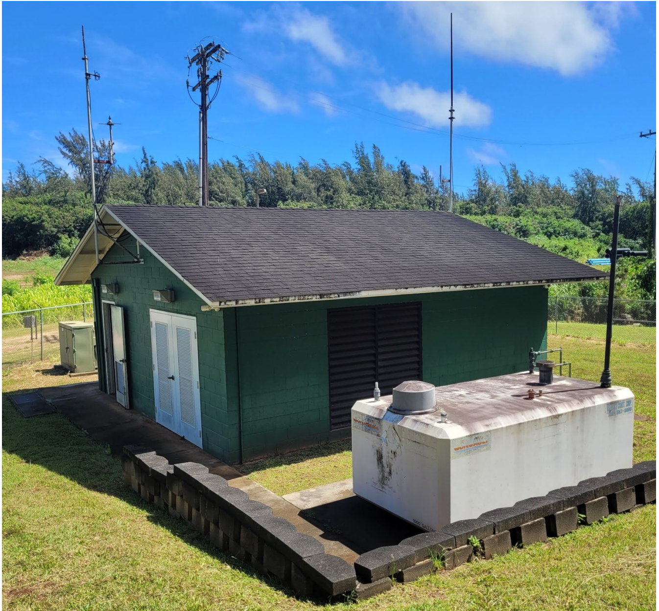
Figure 2-8: Example of Pump Control and Chlorination Building
