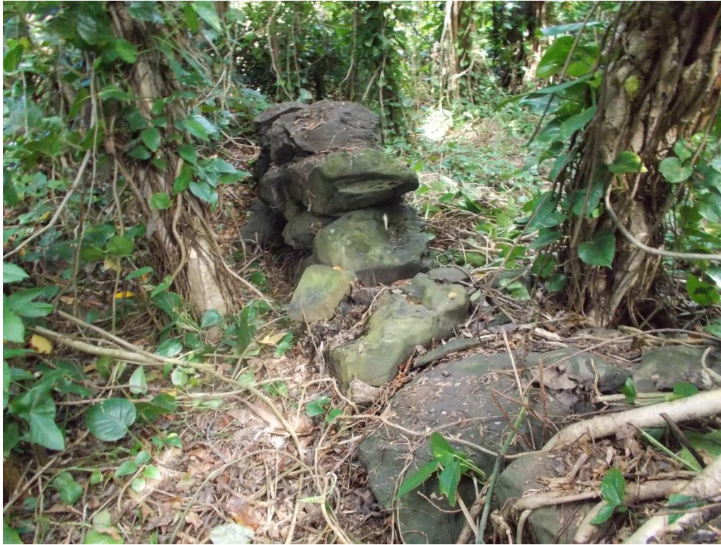
Figure 9. Dry stack rock wall. View facing north.
