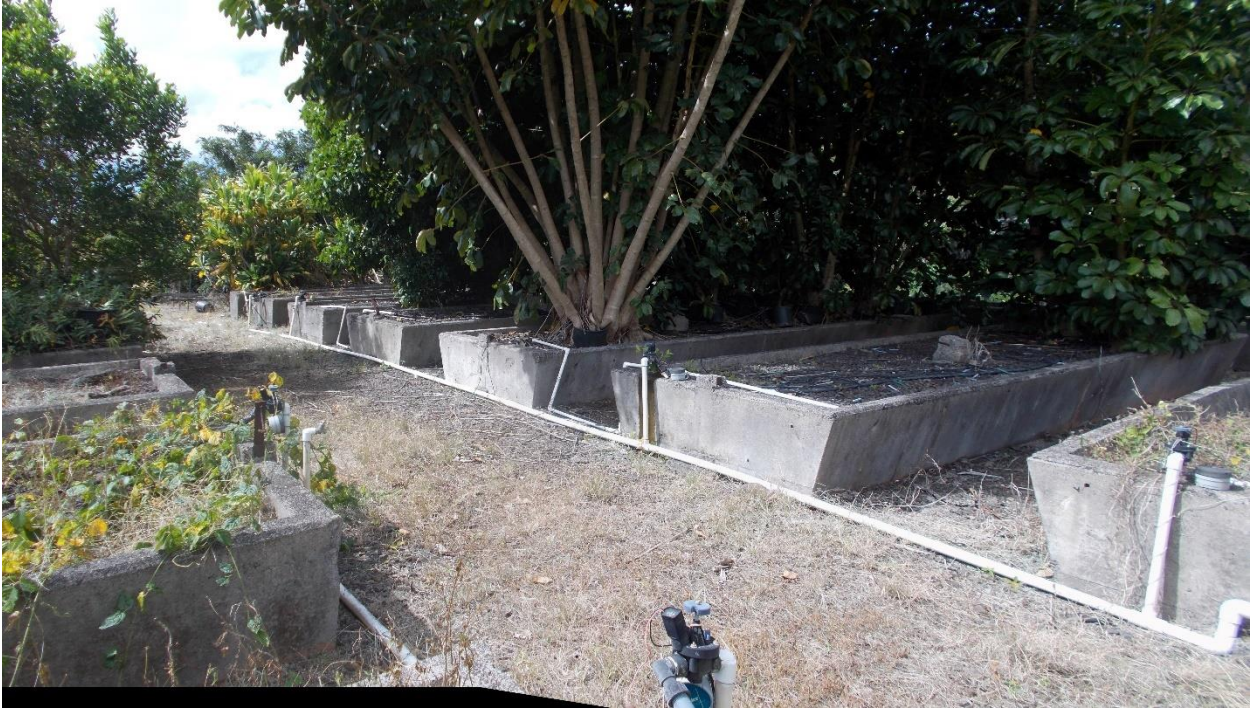
Figure 11. Concrete planters showing aisle between the rows of planters. View facing west.
