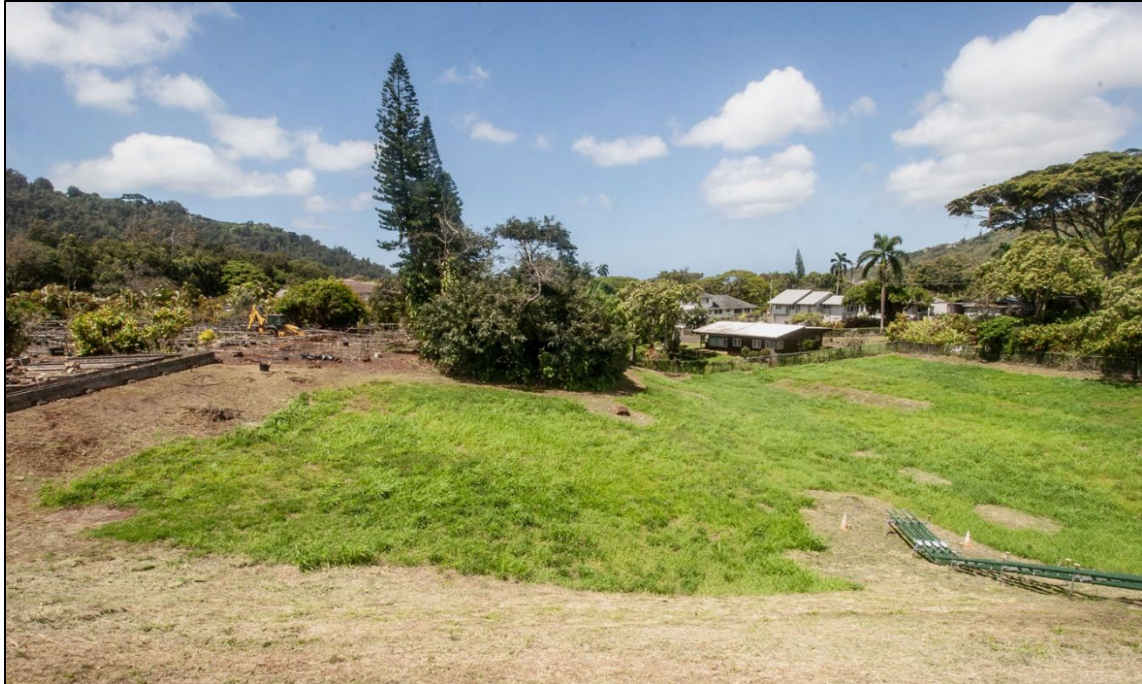
Figure 2. Maintained grassy swale downslope of Nuuanu Reservoir No. 1 showing portion of BWS nursery area on the left. Foreground is downslope face of berm.
