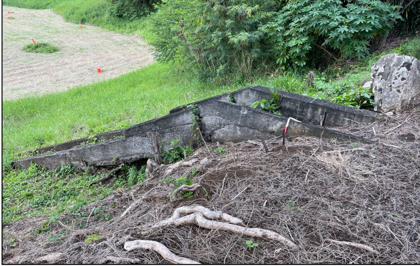
Figure 25. Feature 11 sluice, with Nu‘uanu Reservoir No. 1 below, facing northeast.
