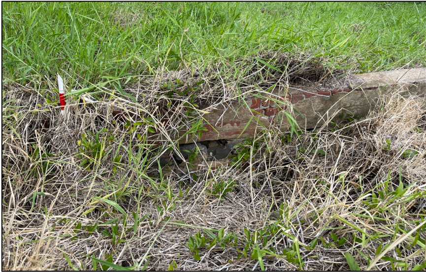
Figure 24. Feature 10 sluice, detail of brick and mortar construction, facing east.
