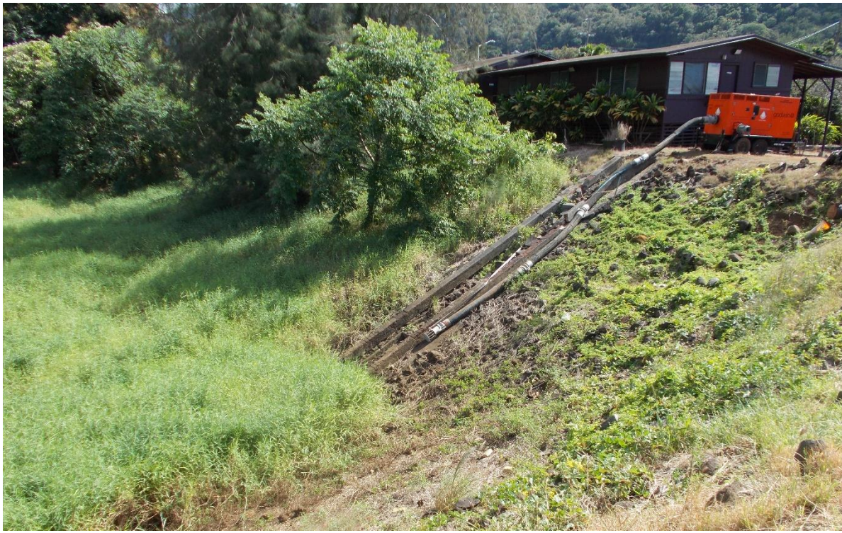
Figure 14. The brick sluice extending down the southeast side of the reservoir. The concrete sluice is out of view in the underbrush to the left. View facing east.
