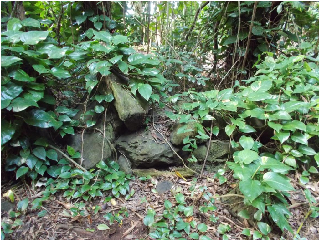
Figure 10. Dry stack rock wall. View facing southwest.
