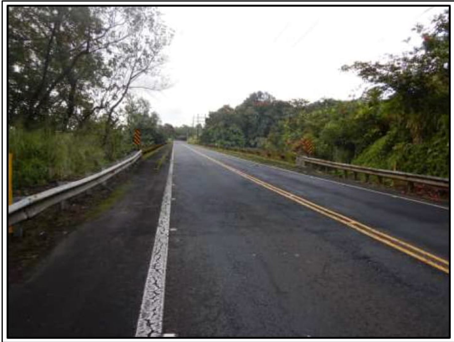
Figure 1-2. View of the Existing Nanue Stream Bridge North Approach (Looking South)
