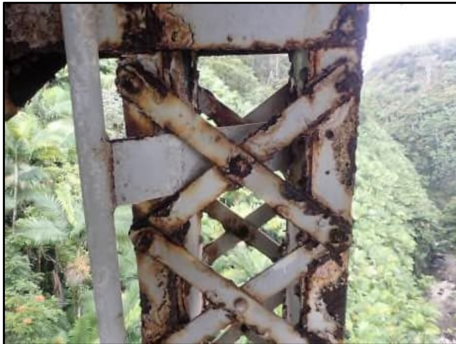
Photograph 44. Bent 3 Level 1, Column D Vertical near top - Corrosion, typical laminar at upper levels (CS 3)
