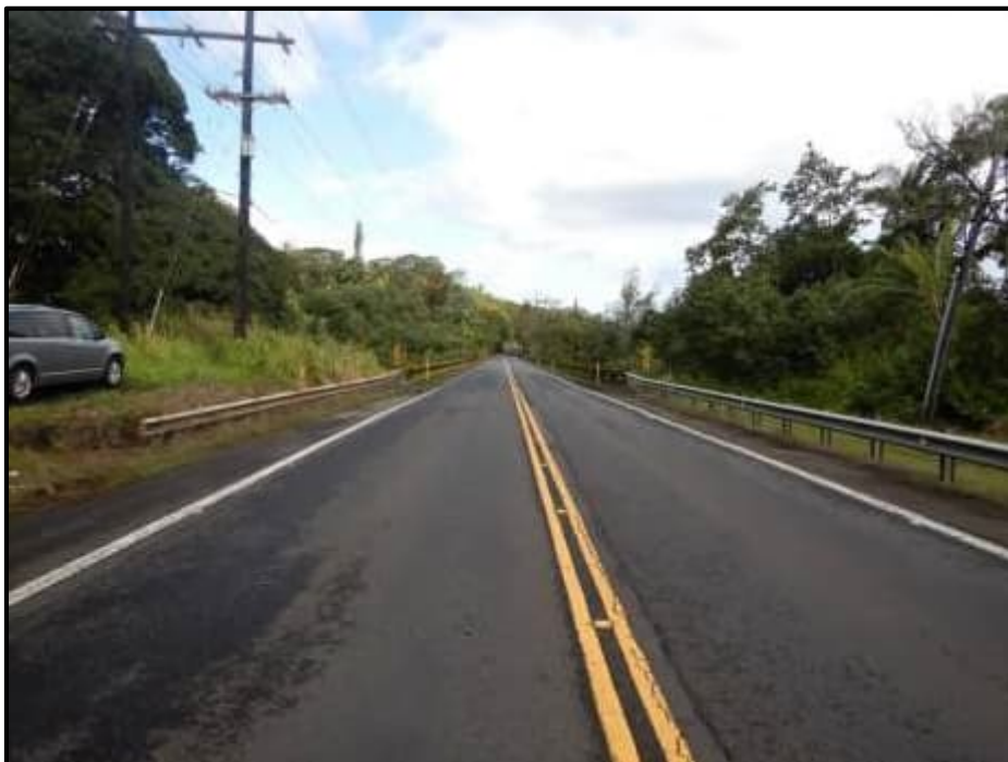
Photograph 4. South Approach (Looking North)
