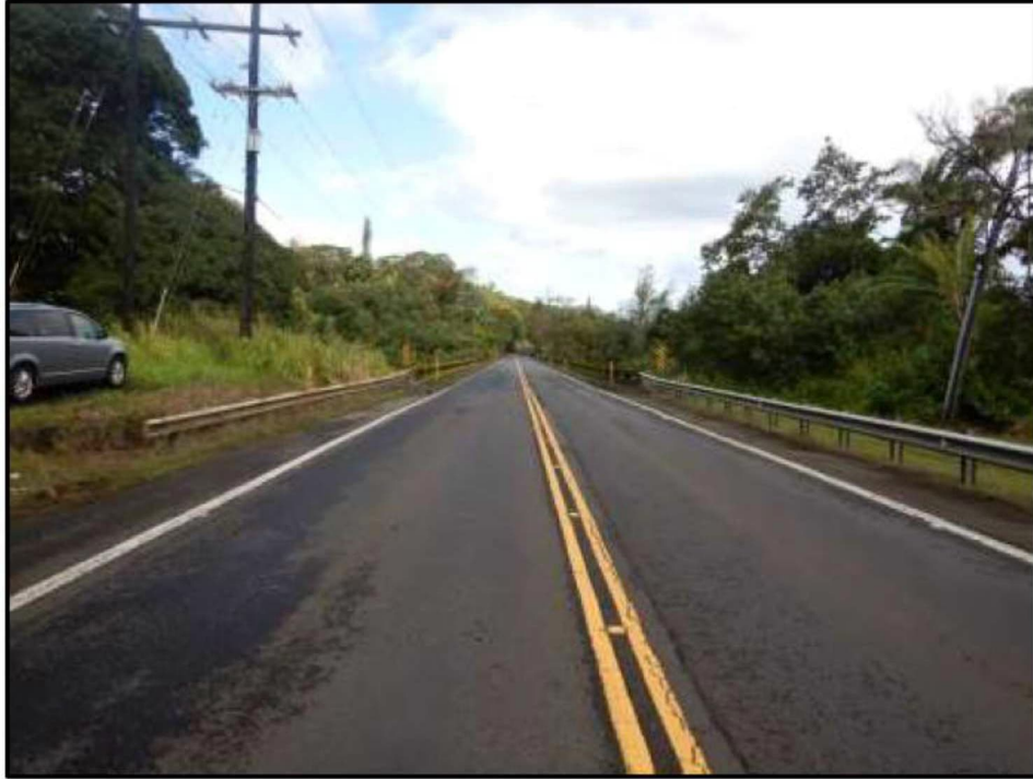
Figure 2c. South Approach (Looking North)
