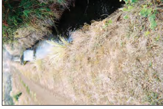
Figure 11: Waihee Ditch (50-50-04-5197) paralleling Old Waikapu Road (50-50-04-5730). View to South.
