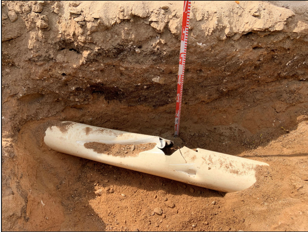
Figure 53. Photograph of T-11 south sidewall, view to south
