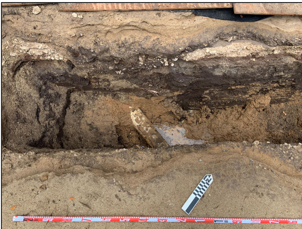
Figure 60. Southwest end of T-13 showing broken PVC fire sprinkler line at 1.13 mbs
