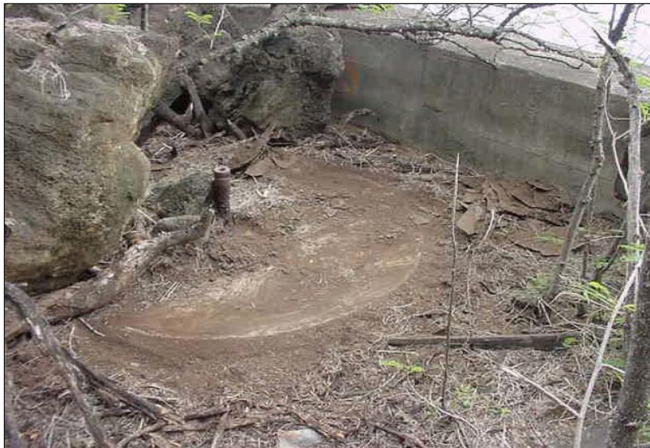
Figure 26. Military coastal gun emplacement (Feature 2) at Site -5929, from Zulick and Cox (2001b:158).
