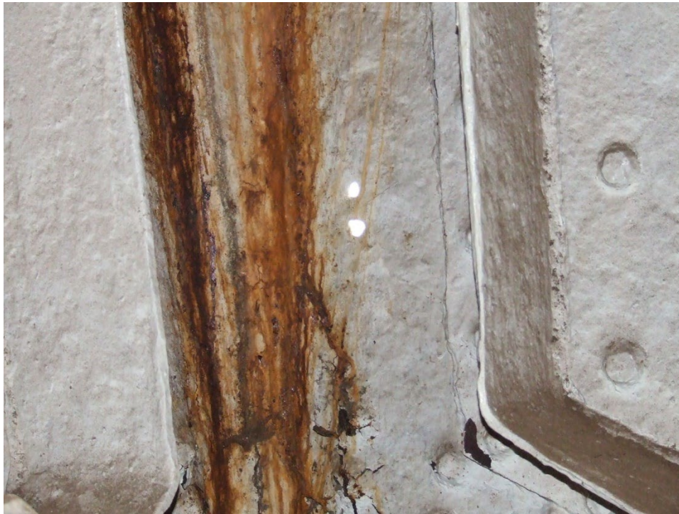
Holed and severely wasted shell plating at stem.
