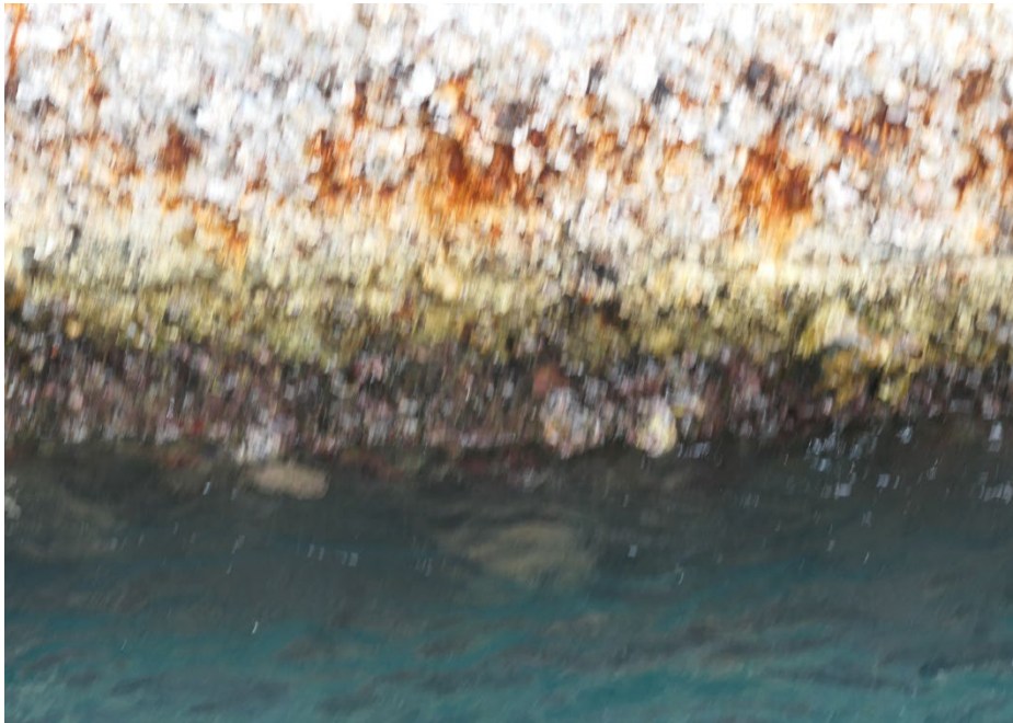
Rusticles formed at the waterline of FOC. Endemic to the entire hull bottom of FALLS OF CLYDE.
