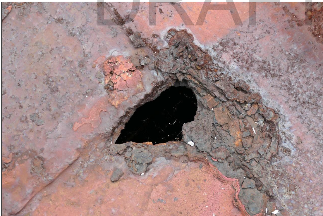
Figure 6: Corrosion has resulted in a loss of structural integrity in a number of areas in the hull and decks (Joseph Lombardi), source: Delgado, “The Four-Masted Ship Falls of Clyde.”
