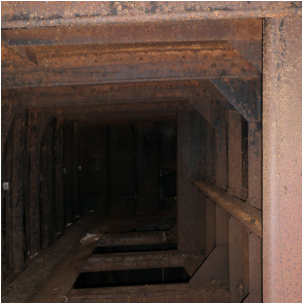
Tank #1, upper flat, looking forward.
