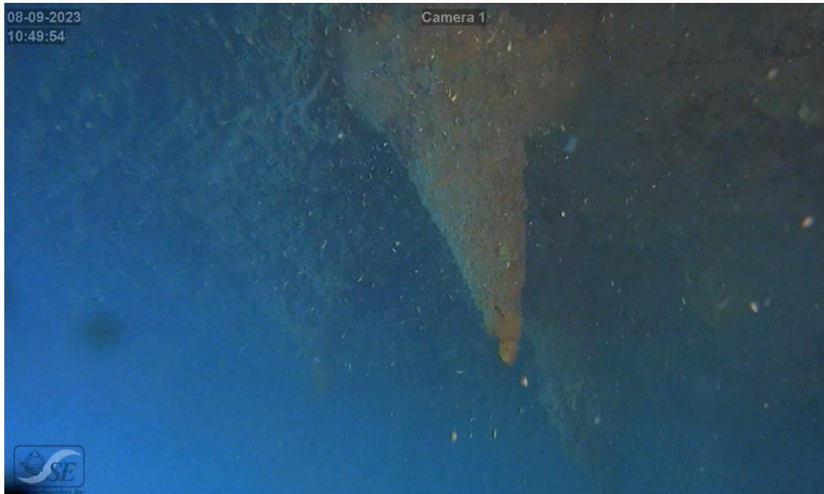
Figure 1: Typical cone shaped corrosion protrusion, appears throughout vessel. Protrusions appeared more frequent towards bottom of hull.
