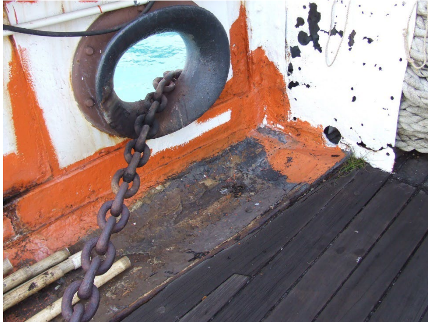
Concrete in waterways causing degradation to substrate. Notice wasted plating in right portion of photo.
