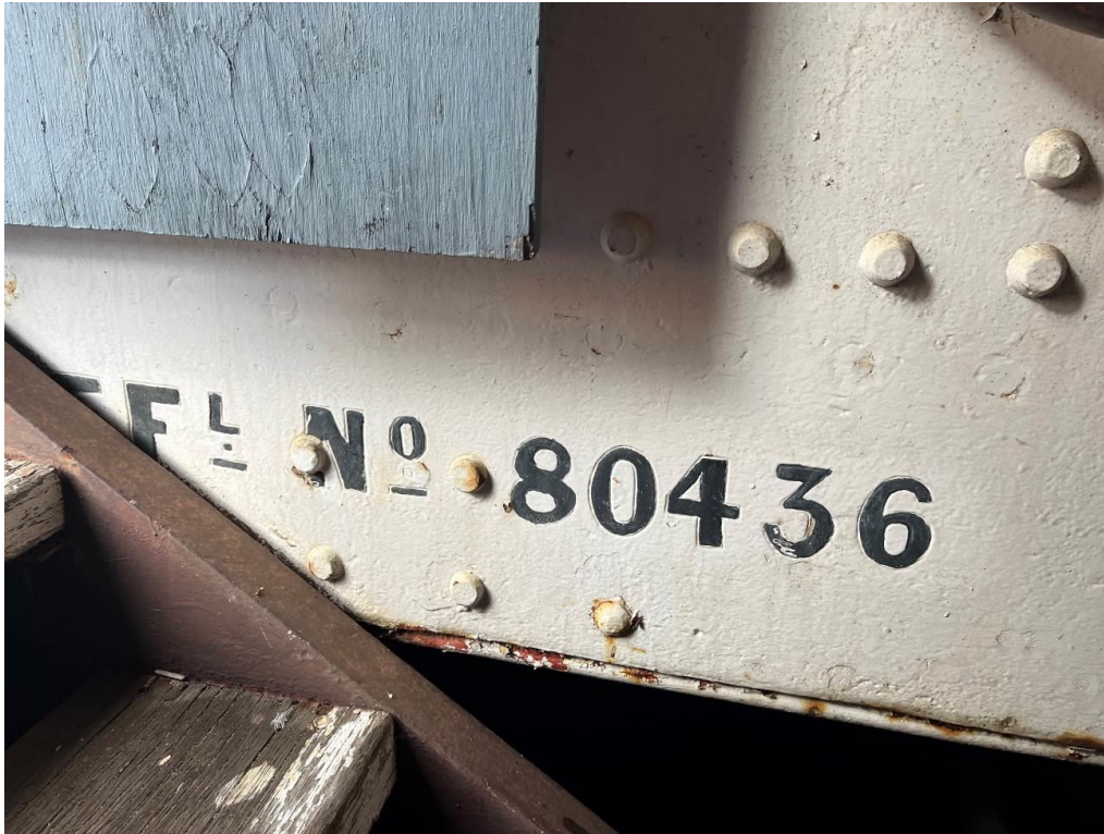
Figure 1: The main hatch coaming has the ship's Official Number from its registration as a British vessel in 1878. If the vessel were to be scrapped, retention of this coaming, if possible, would make it a significant relic of the vessel.
