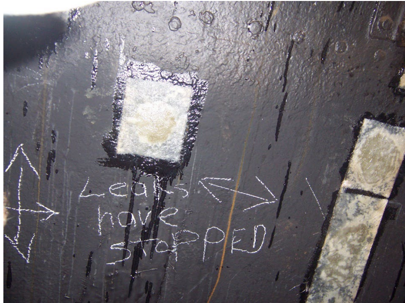
Re-patched holes in bulkheads in Tank #4 port.
