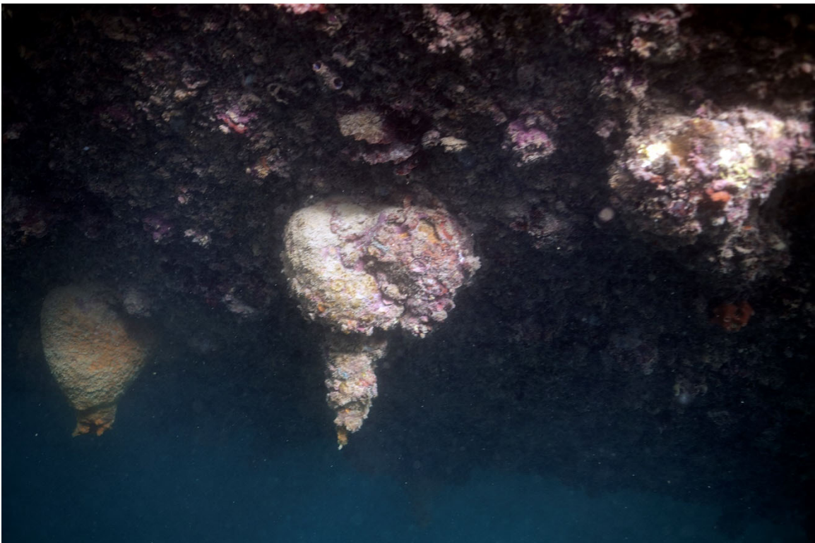
Figure 5 Funnel-Shaped Protrusion Consisting of Rust on the Hull of the Falls of Clyde.
