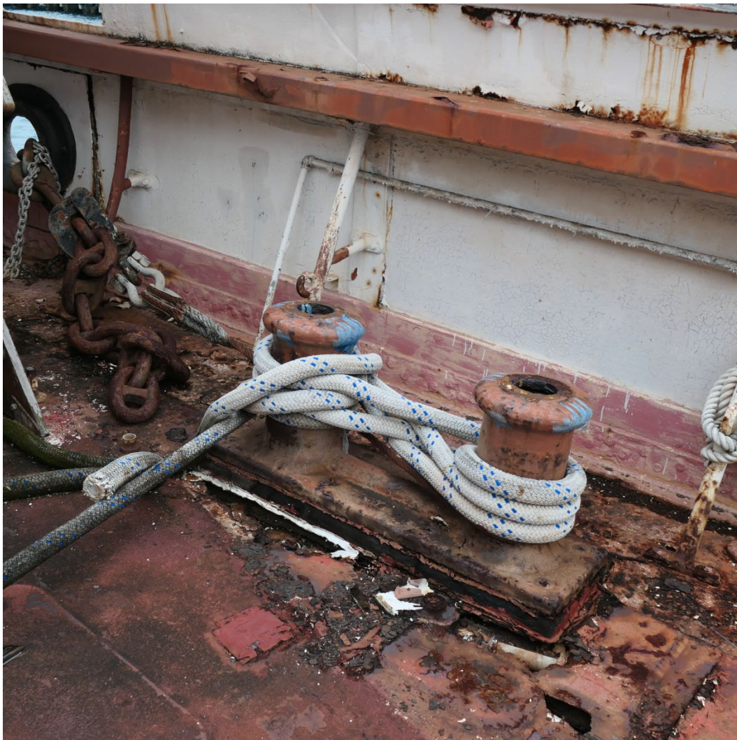
Double bitts made up with line and chain. Load of chain pulling bulwark in around chock. Double bitts pinned to rotted laid deck and iron substrate. Absolute junk....
