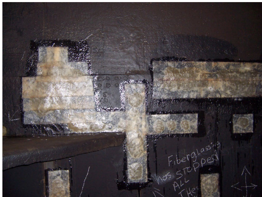
Patched bulkhead in Tank #3.
