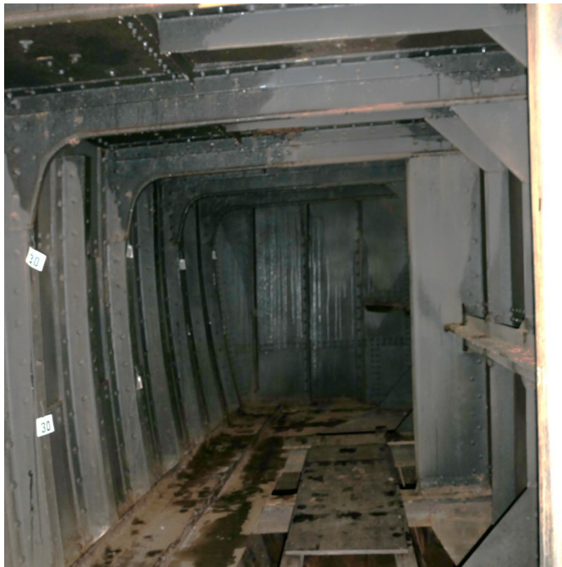
Tank #4 Port, looking forward.
