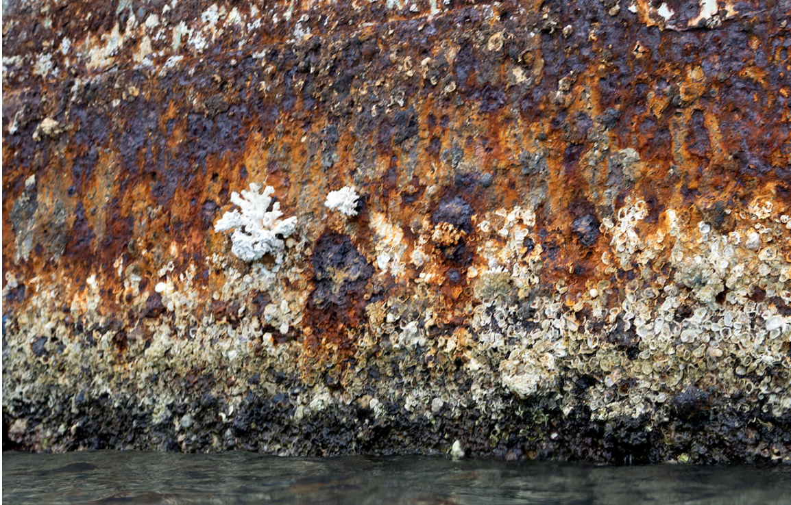
Figure 16 Dead Colonies of P. damicornis (Visible as Pure White Branching Skeleton) Above the Waterline on the Hull of the Falls of Clyde.
