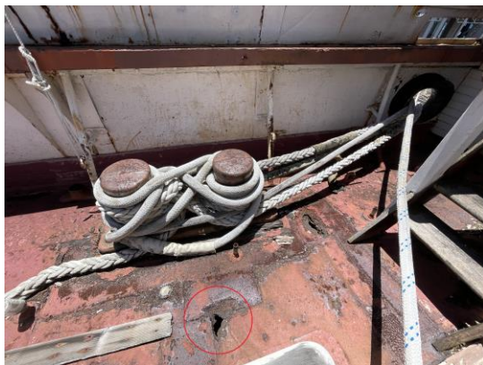
Photo #3, main deck wastage
