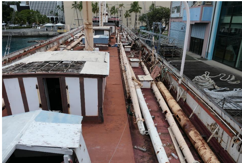
Figure 18: The corroding, dry-rotted and crowded decks of the ship are in danger of collapse and a hazard to anyone who boards the vessel (Joseph Lombardi).
