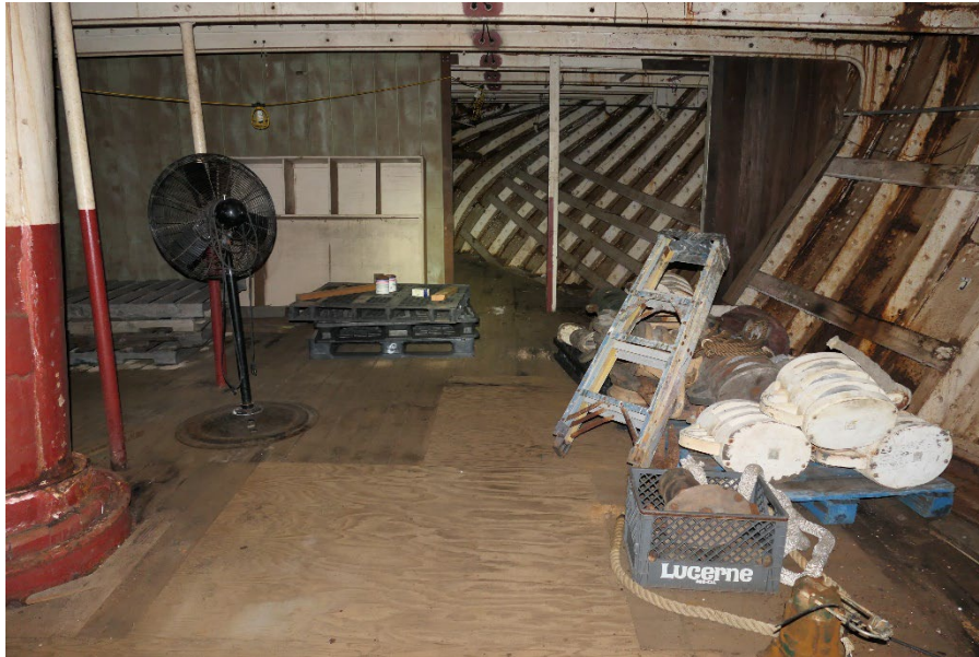
Storeroom, looking aft to port.
