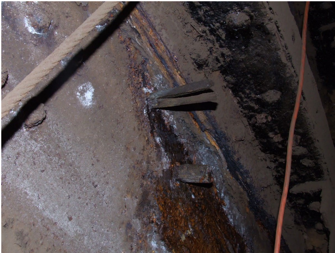
Wooden plugs keeping the ocean out.
