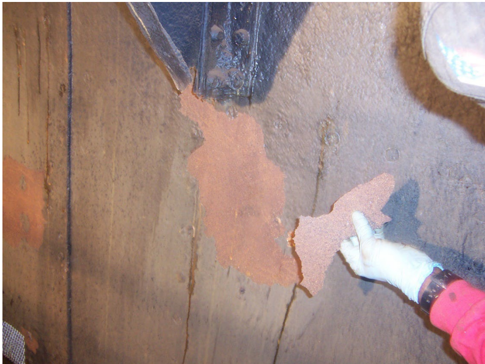
New paint system failure on bulkhead.
