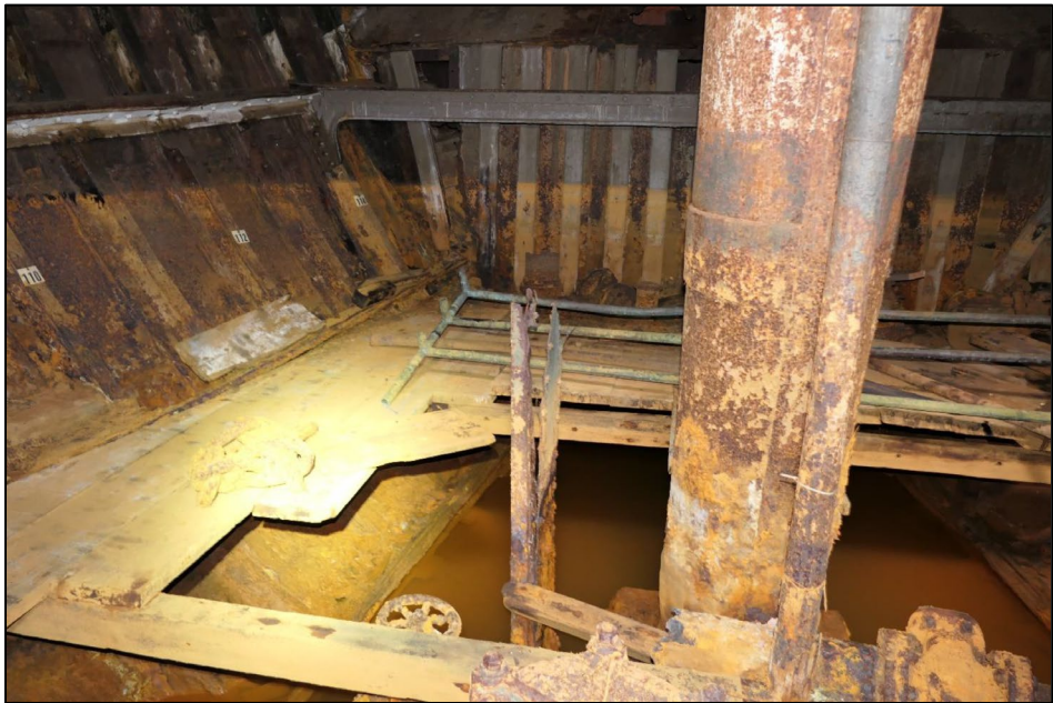
Figure 4: Corroded base of the foremast in the bilge, March 2023 (Joseph Lombardi), source: Delgado, "The Four-Masted Ship Falls of Clyde."
