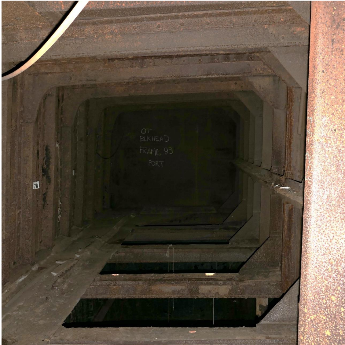
Figure 13: Interior of one of the tanks (Joseph Lombardi).
