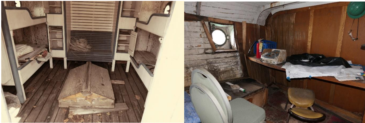
Figure 20: Condition of interior spaces, 2023 (Joseph Lombardi).
