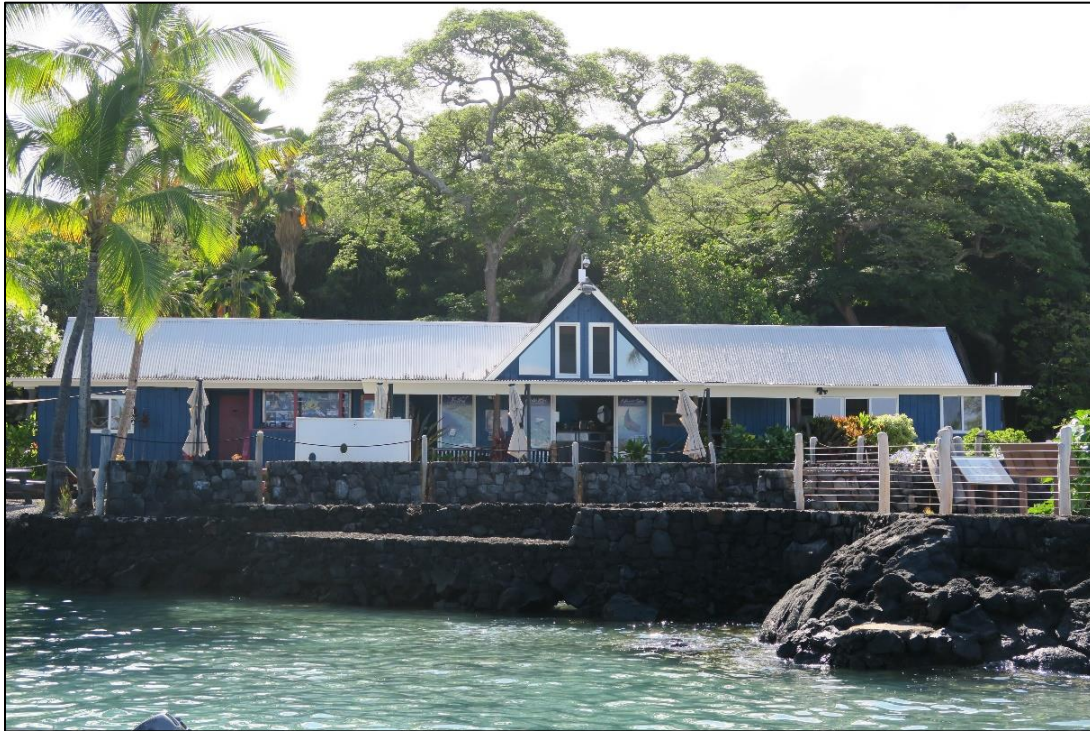
Figure 4-24 Former Machado House Now the Headquarters of Fair Wind Cruises
