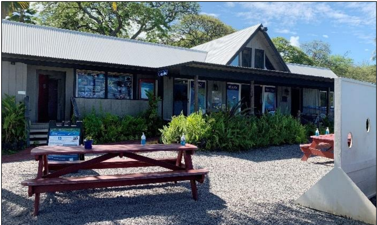
Figure 3-62 Existing Ocean Recreation Commercial Building Entrance
