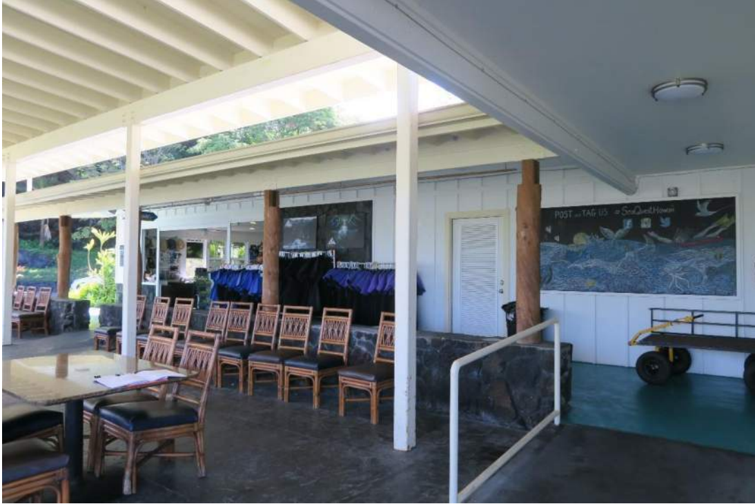
5. Covered Lanai with Original Lava Rock Pony Wall And Ohia Tree Wood Posts
