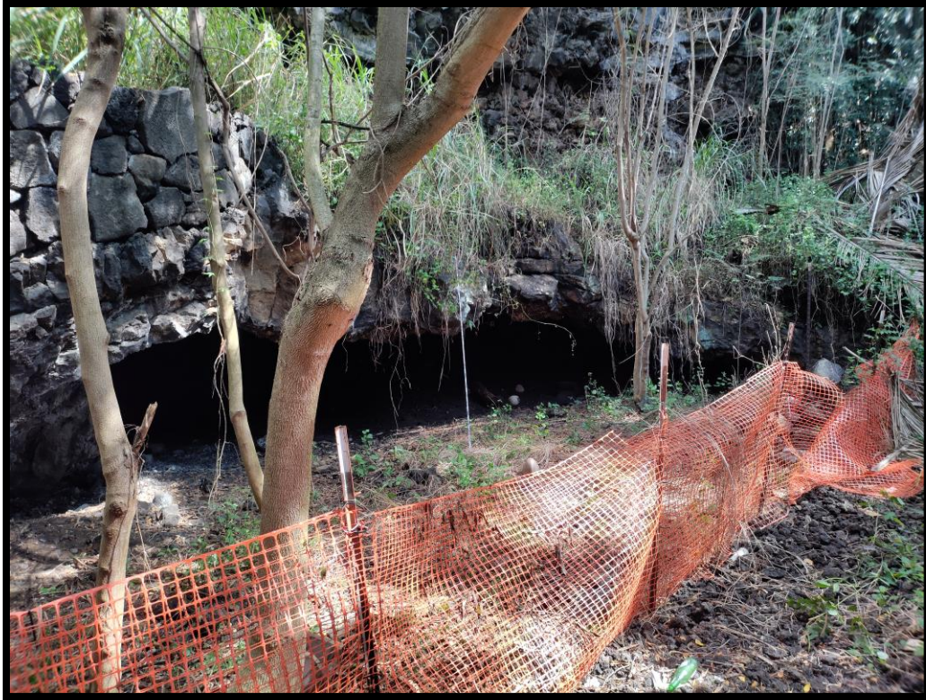
Figure 41. Current condition of entrance to Site 24264 Mo'ikeha Cave (view to southeast).
