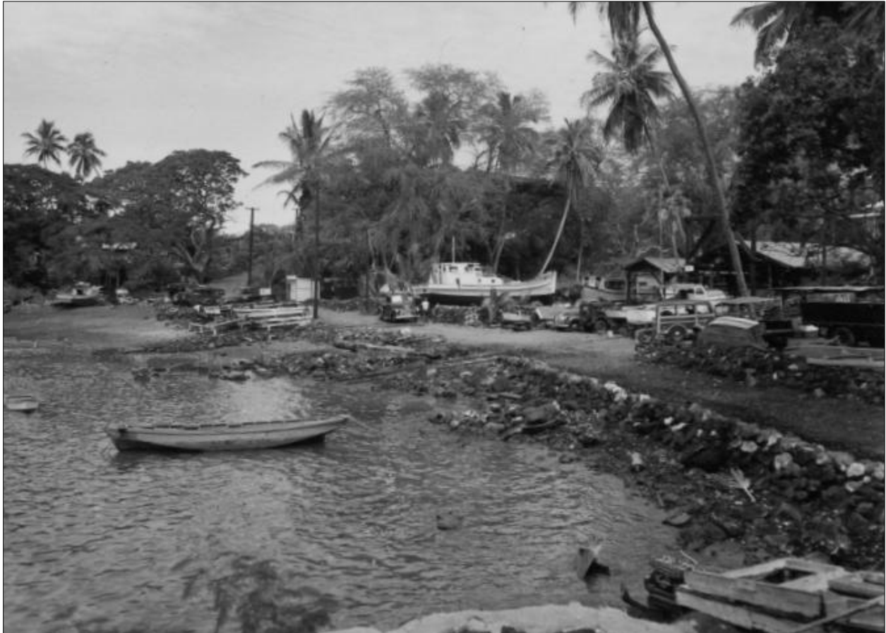
Figure 45. Keauhou Bay in February 1950 showing absence of pier and the Machado dry-dock where the boat and vehicles are parked (Hawai'i State Archives PP-29-11-003).
