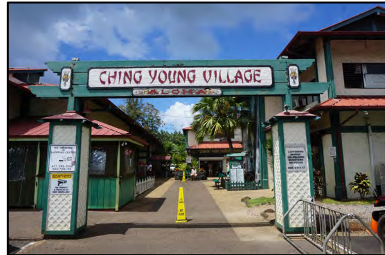
Photo 20: Shopping center entrance between Building A (left) and Building D (Right) Facing North.
