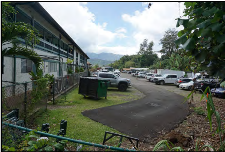
Photo 17: Area view of north border of the Property facing west from east parking lot.
