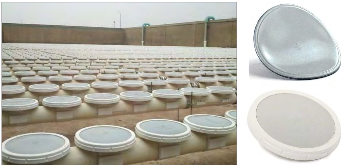
Figure 4: Example ECD Diffusers with PTFE Membranes
