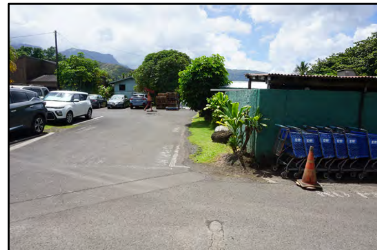
Photo 8: View of existing WWTP enclosure (right side of photo). Facing West.
