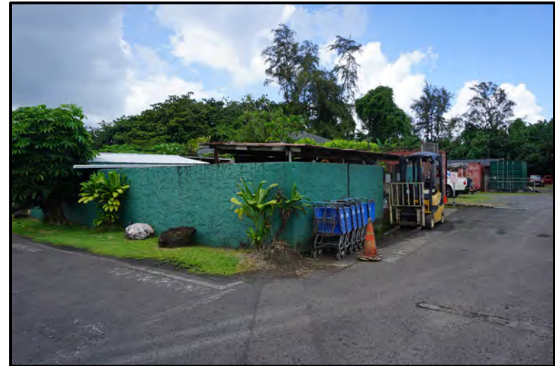
Photo 2: View of existing WWTP enclosure. Facing northwest.
