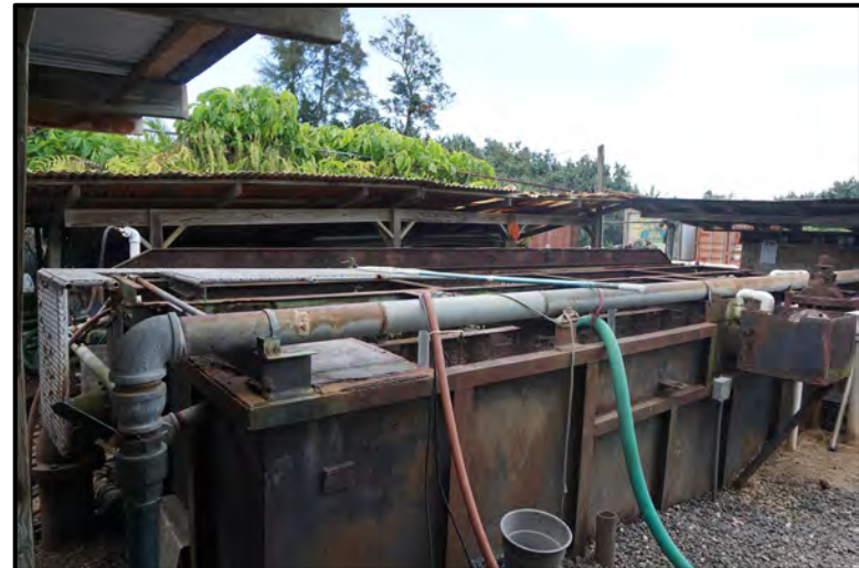
Photo 11: Interior view of existing WWTP enclosure. Facing northeast.
