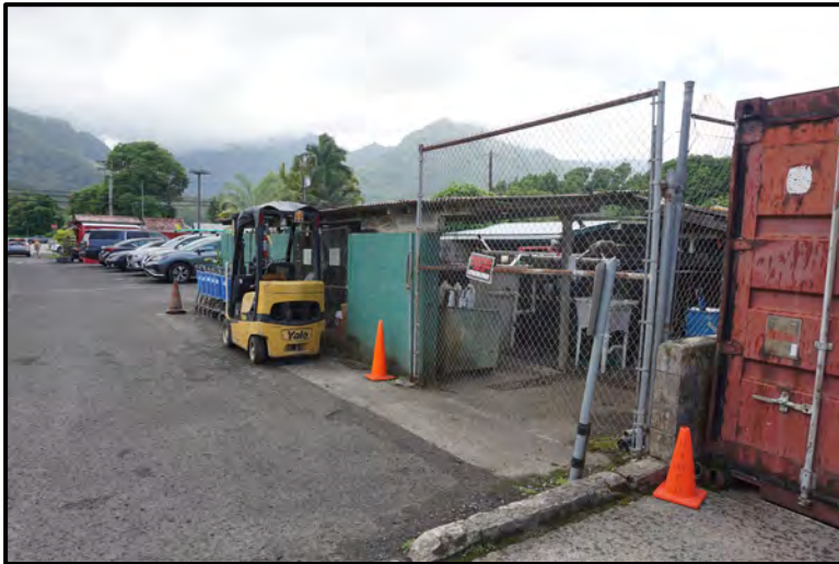
Photo 1: View of existing WWTP enclosure. Facing South. Property line ends at short concrete wall in lower right.
