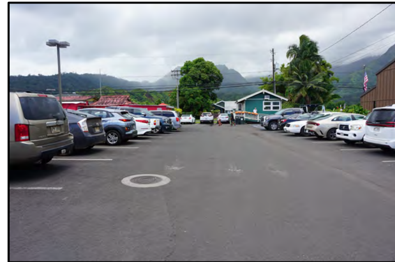
Photo 6: Western portion of West parking lot. Facing south. General location of existing primary injection wells.
