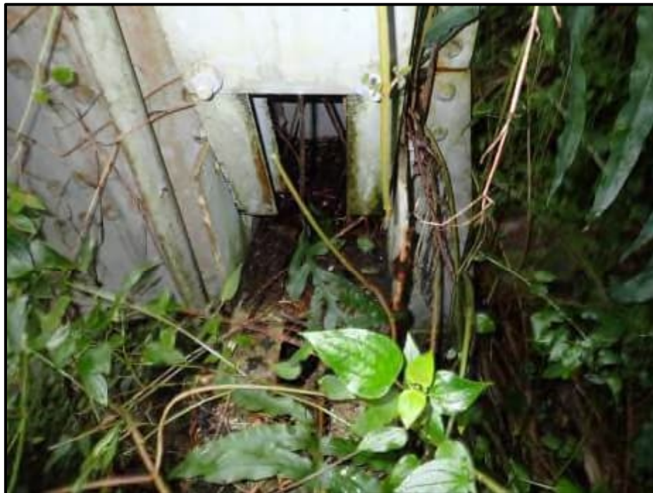
Photograph 43. Bent 3 Level 5, Column A just above bearing, gusset plates - Damage, plates are bowed to the South up to 1/8" for the horizontal bracing member (CS 4)
