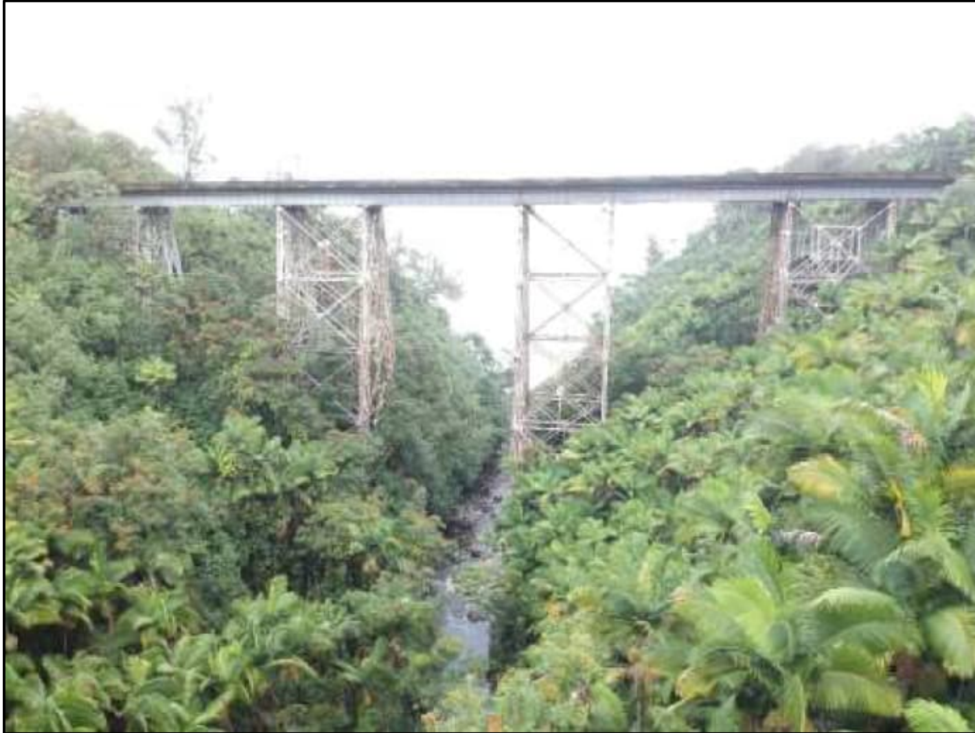
Source: Routine Bridge Inspection Report, Nanue Stream Bridge, March 19, 2021
