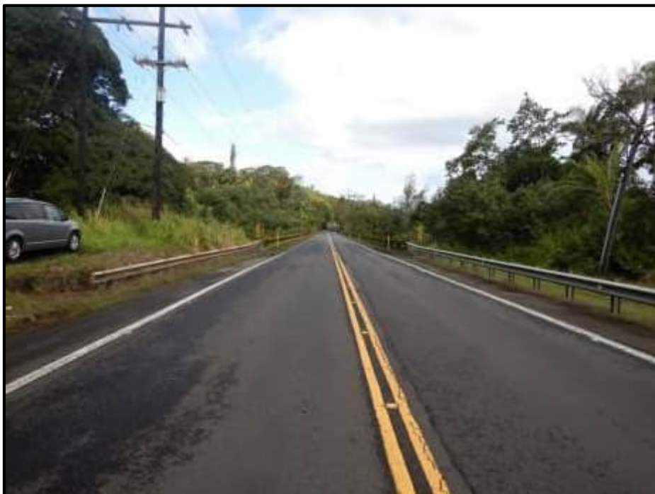
Photograph 4. South Approach (Looking North)
