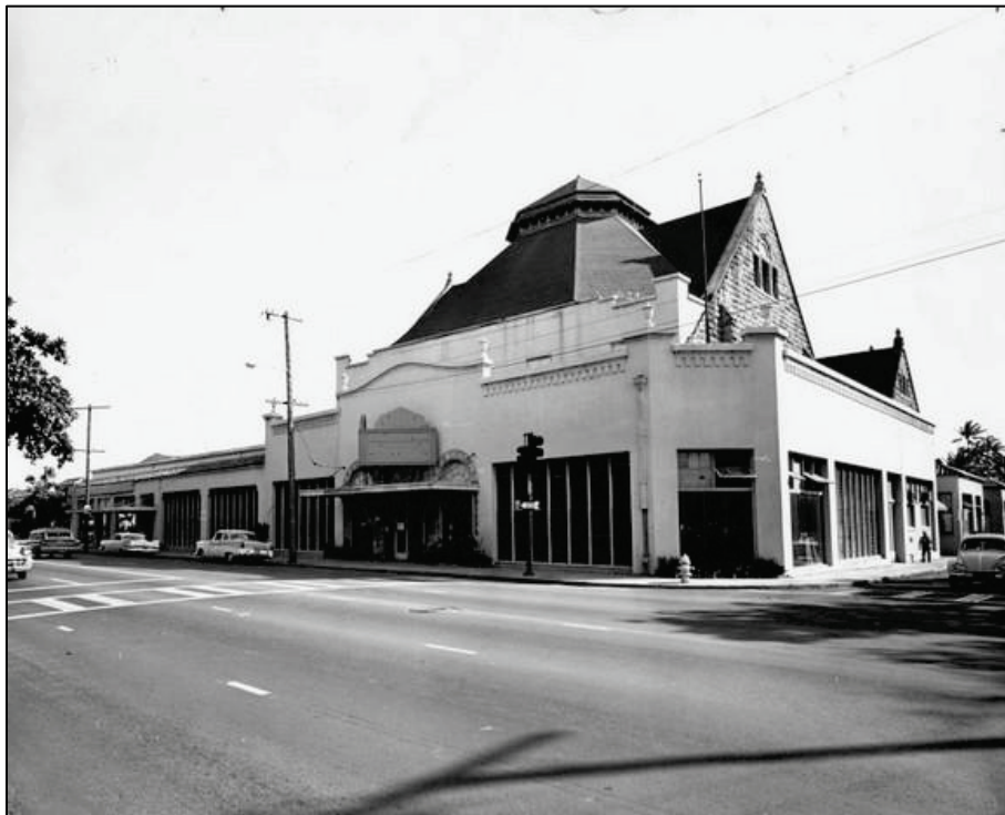
FIGURE 3-5 SCHUMAN CARRIAGE BUILDING PRIOR TO ITS DEMOLITION FOR THE CONSTRUCTION OF THE STATE CAPITOL BUILDING LOOKING TO THE SOUTH FROM THE INTERSECTION OF SOUTH BERETANIA AND RICHARDS STREETS. CIRCA 1950.
