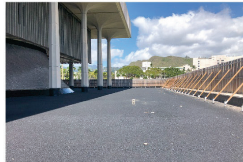
Photo 7: Existing condition of the Diamond Head Capitol pool, looking mauka. Repairs to basin surface completed. (HHF Planners, 2024)
