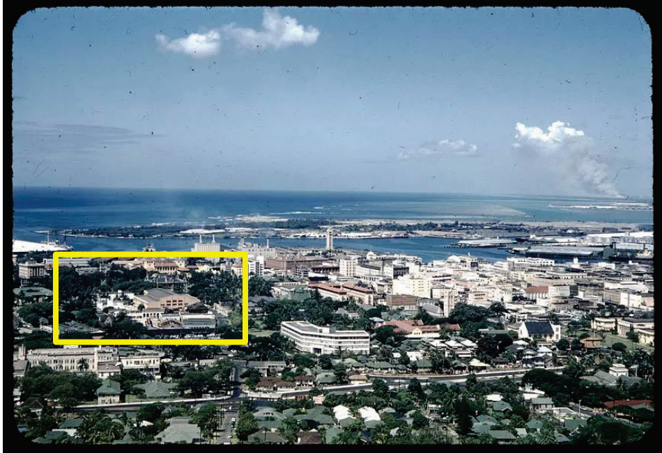
FIGURE 3-4 OBLIQUE VIEW OF DOWNTOWN HONOLULU, LOOKING MAKAI, AUGMENTED TO CLARIFY LOCATION DISCUSSED. CIRCA 1956.
