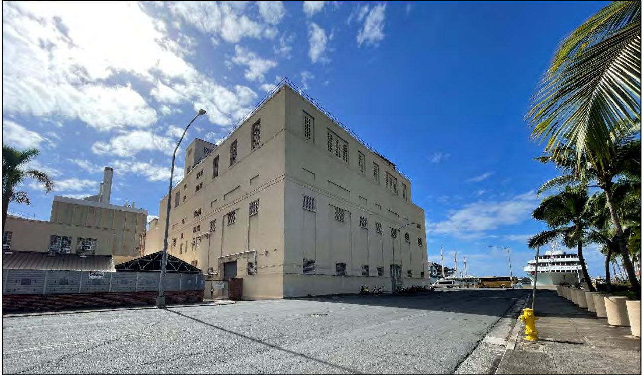
Figure 40. Northeast and northwest facades of HECO Honolulu Power Plant, Unit 7 (background) and Unit 5 (foreground), camera facing south (MASON, 2024).
