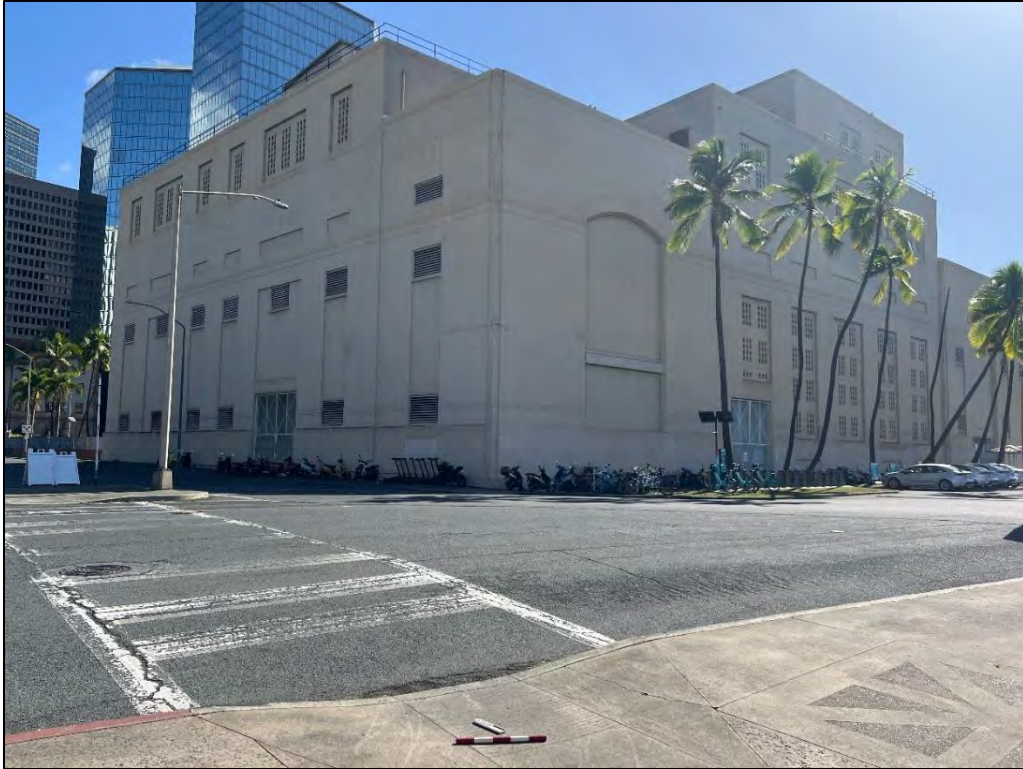
Figure 42. Photo of the Honolulu Power Plant at the corner of Aloha Tower Dr. (foreground) and Bishop St. (to the left), view to east
