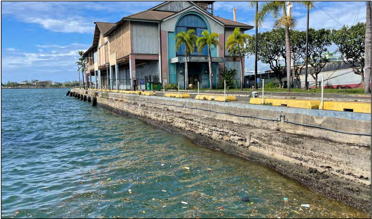
Figure 32. Southeast side of Pier 7, camera facing west (MASON, 2024).
