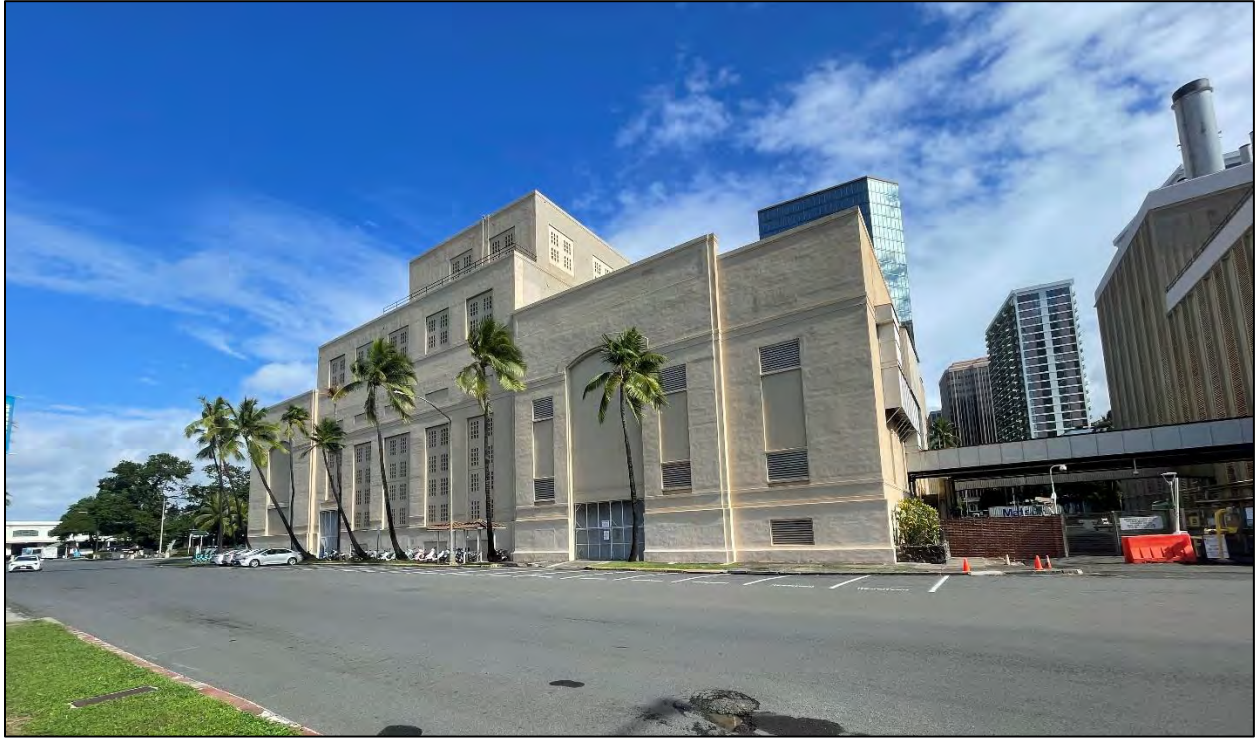
Figure 43. Southwest facades of HECO Honolulu Power Plant, Unit 7 (foreground) and Unit 5 (background), camera facing northeast (MASON, 2024).
