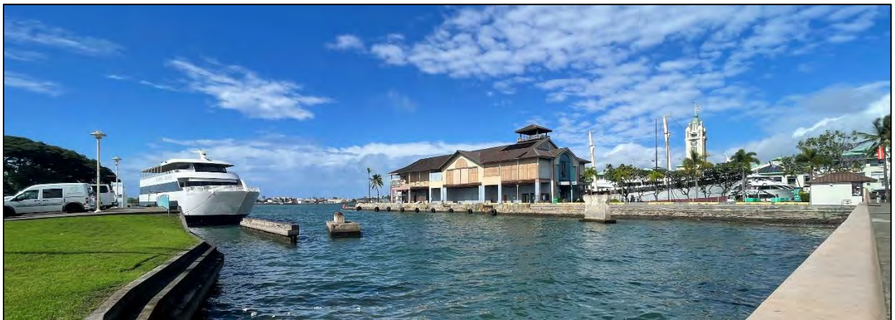
Figure 30. Southeast side of Pier 7, camera facing northwest (MASON, 2024).
