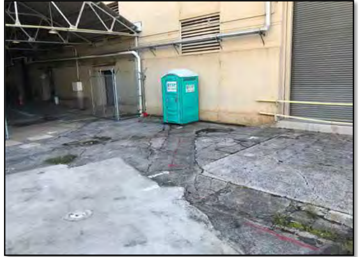
Photo 2: Underground utility marking during utility toning.
