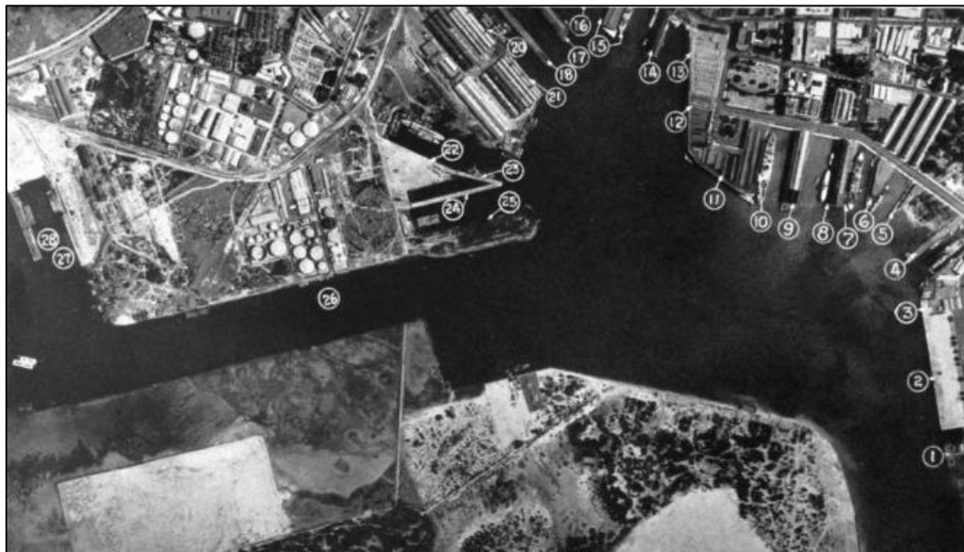
Figure 16. Aerial photo of Honolulu Harbor showing Kalihi Channel, ca. 1935. Source: War Department, Corps of Engineers, Ports of the Territory of Hawaii (Washington: Government Printing Office, 1935), 46.
