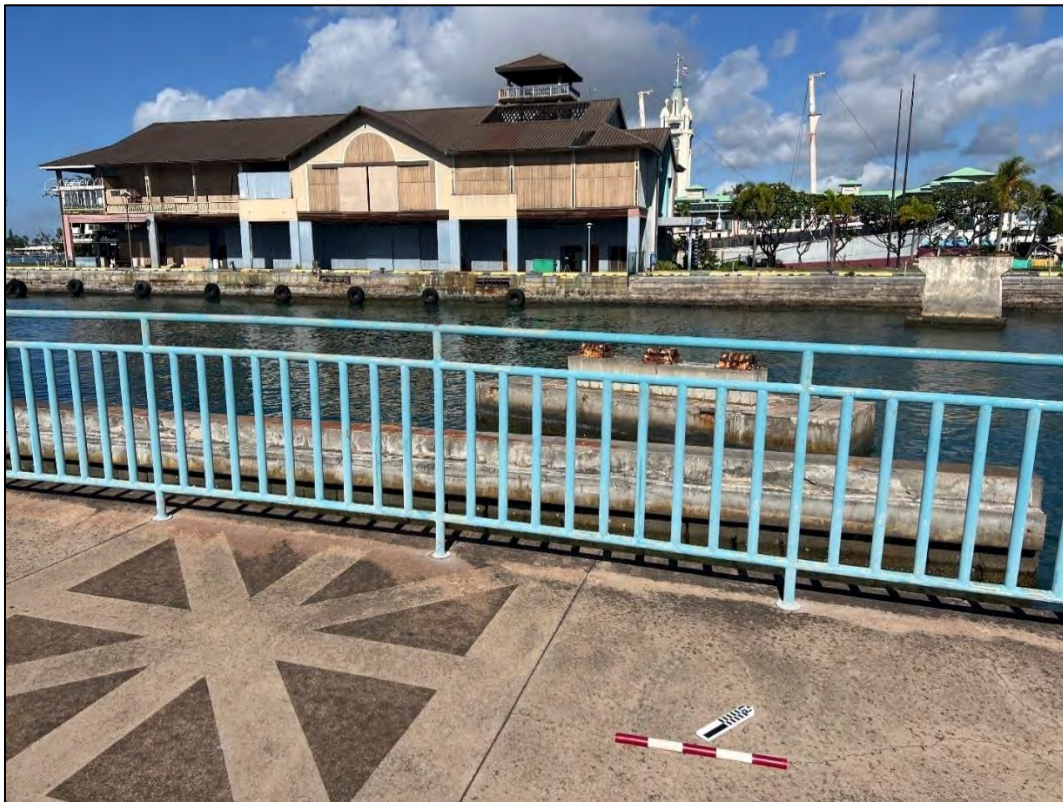
Figure 46. Photo looking towards Pier 7, notice the former Maritime Center upon the dock (also notice the concrete footing in the water slip likely associated with the formerly existing elevated ramp [1964-1980s]), view northwest
