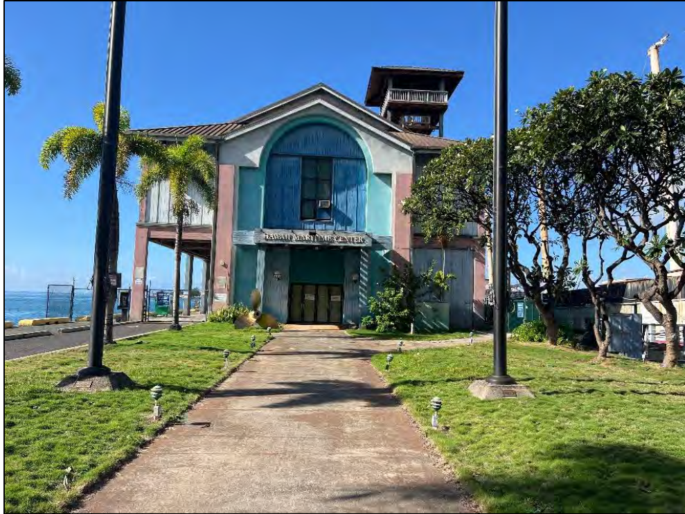
Figure 47. Photo on Pier 7 showing the former Maritime Center (east side), view southwest
