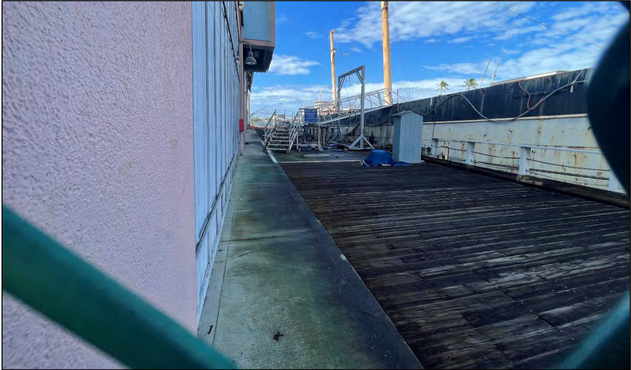
Figure 31. Northwest side of Pier 7, camera facing southwest (MASON, 2024).
