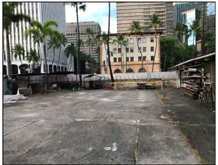
Photo 12: Site conditions at the end of Phase II ESA work.
