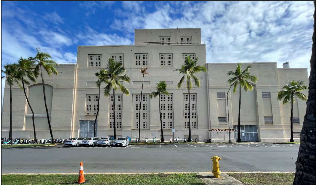
Figure 37. Southwest facades of HECO Honolulu Power Plant, Unit 5 (left) and Unit 7 (right), camera facing northeast (MASON, 2024).
