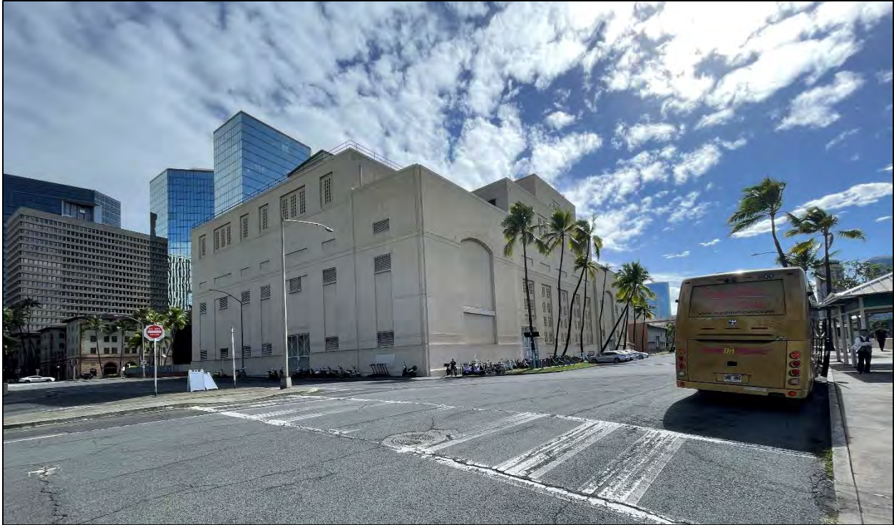
Figure 38. Northwest and southwest facades of HECO Honolulu Power Plant, Unit 5 (foreground) and Unit 7 (background), camera facing southeast (MASON, 2024).
