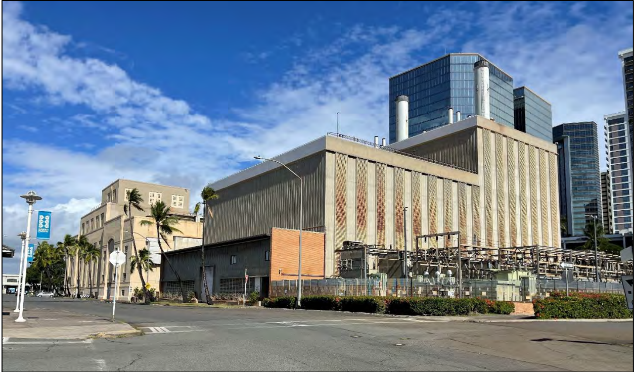
Figure 44. Southeast and southwest facades of Hicks Power Plant (foreground, not part of the project or survey area) and HECO Honolulu Power Plant, Unit 7 (background), camera facing northeast (MASON, 2024).
