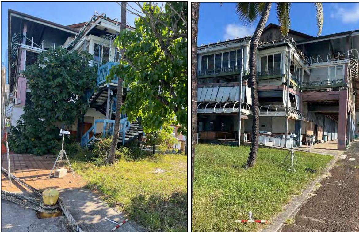
Figure 48. Photos on Pier 7 showing the former Maritime Center (west side), view northeast (left) and north (right)
