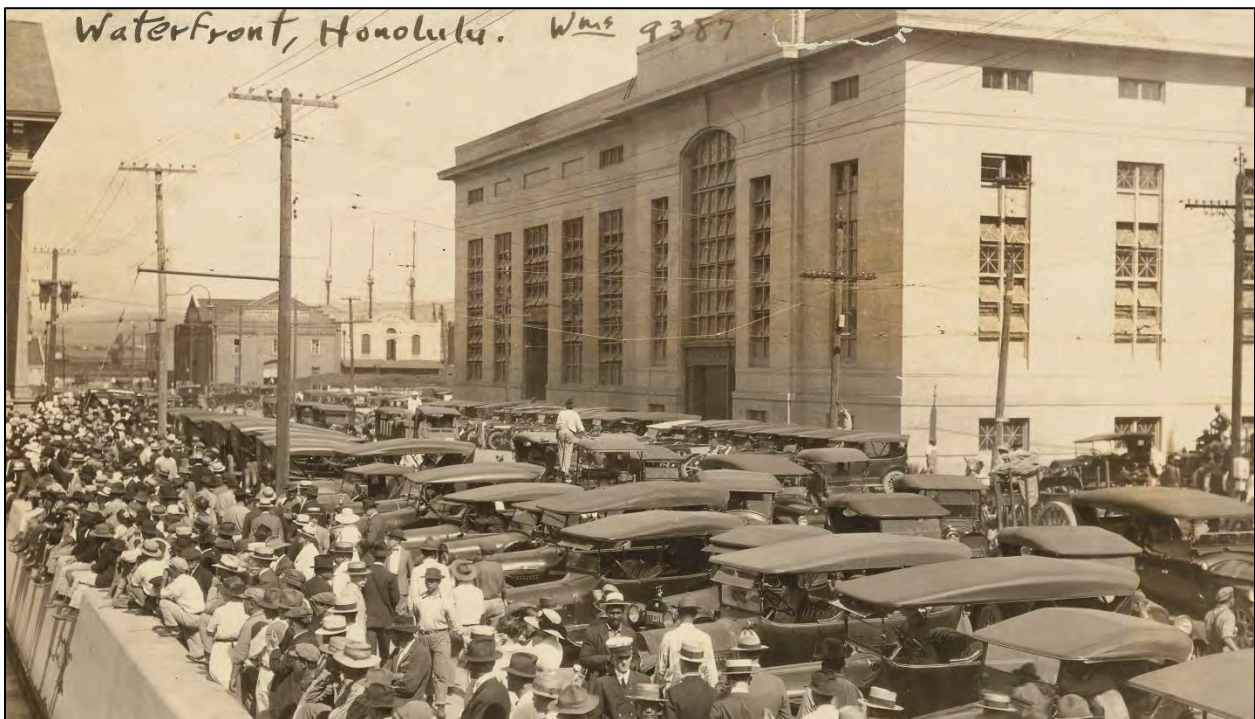
Figure 22. Photo of HECO Honolulu Power Plant, Unit 5, ca. 1920. Source: "Photos: What Honolulu Harbor Looked Like in the 1920s," Local News, KHON, accessed January 18, 2024.
