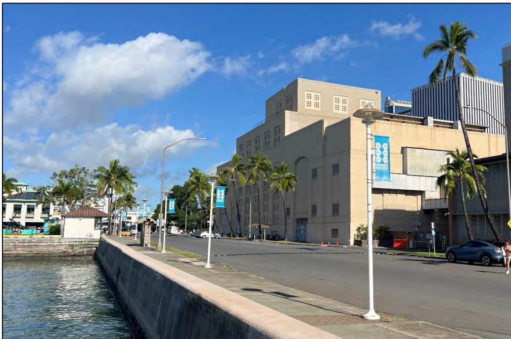
Figure 43. Photo of the south side of the project area showing the Honolulu Power Plant (on right), Aloha Tower Dr. (center), and Pier 7 (on left), view to north
