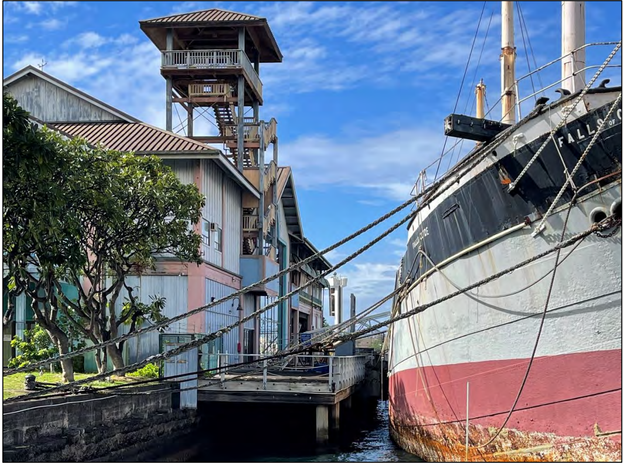
Figure 35. Northwest façade of former Maritime Center, camera facing southwest (MASON, 2024).
