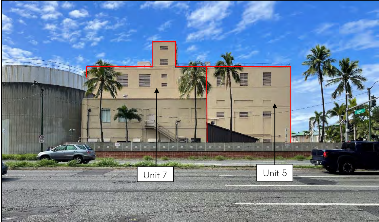
Figure 42. Northeast facades of HECO Honolulu Power Plant, Unit 7 (left) and Unit 5 (right), camera facing southwest (MASON, 2024).
