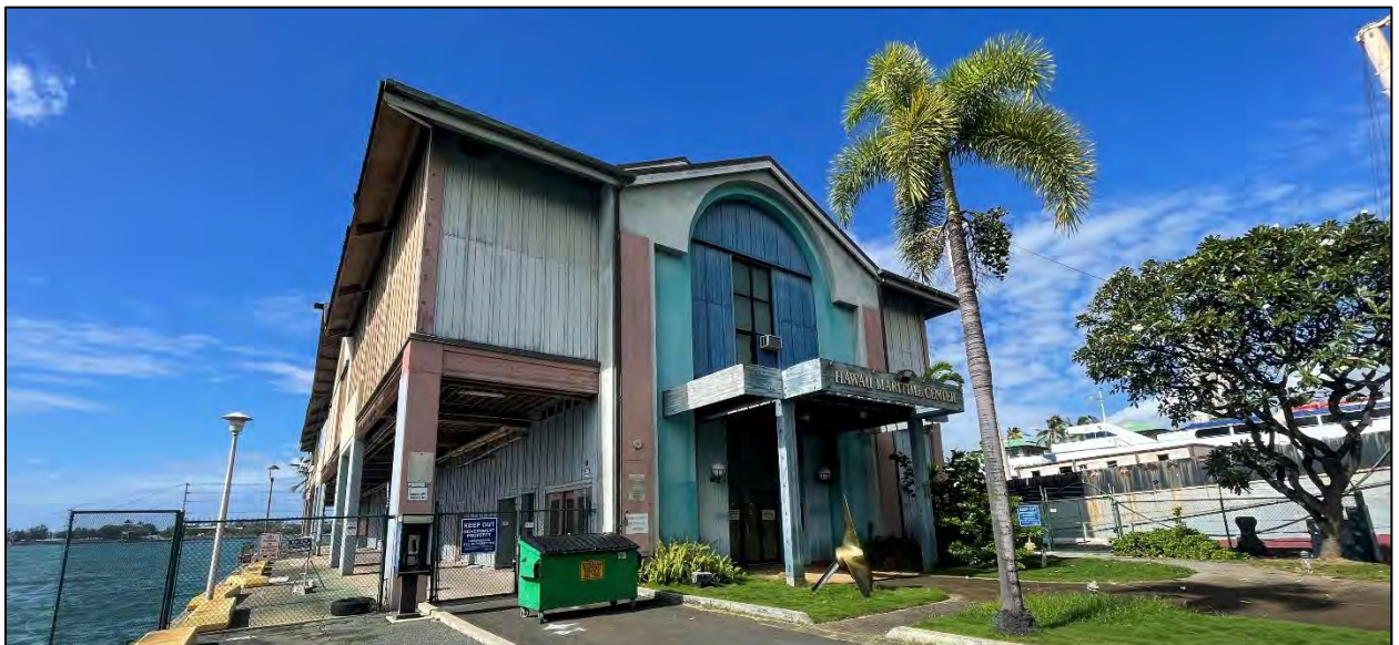
Figure 34. Northeast facade of former Maritime Center, camera facing west (MASON, 2024).
