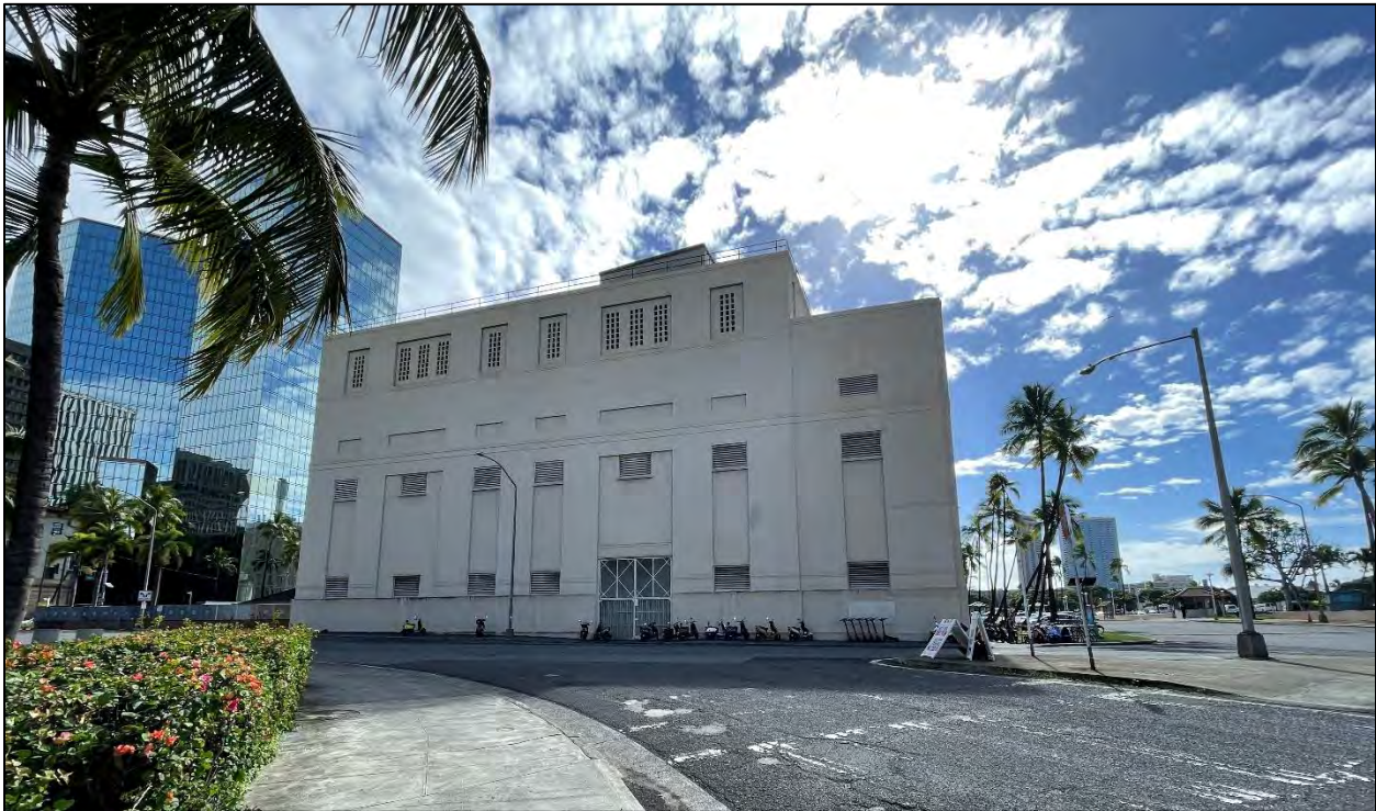
Figure 39. Northwest facades of HECO Honolulu Power Plant, Unit 5, camera facing south southeast (MASON, 2024).
