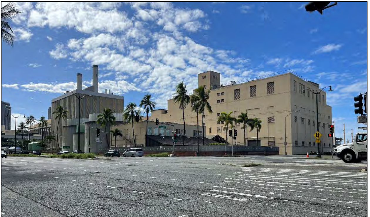
Figure 41. Northeast and northwest facades of HECO Honolulu Power Plant, Unit 7 (left) and Unit 5 (right), camera facing south southwest (MASON, 2024).
