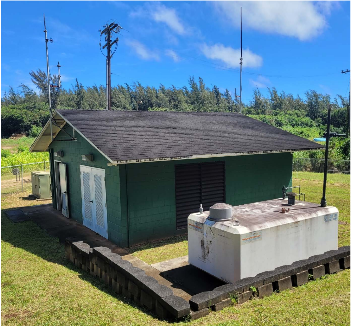
Figure 2-8: Example of Pump Control and Chlorination Building
