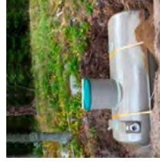
Steel, Horizontal, Cylindrical Tank
