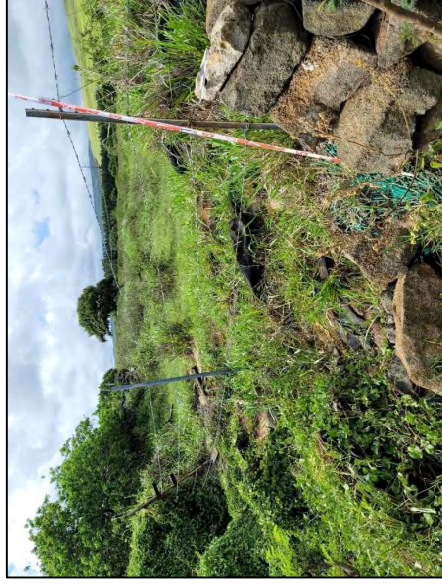
Figure 138. Photograph showing core-filled construction along a section of the SIHP # -30930 rock wall; view to north
