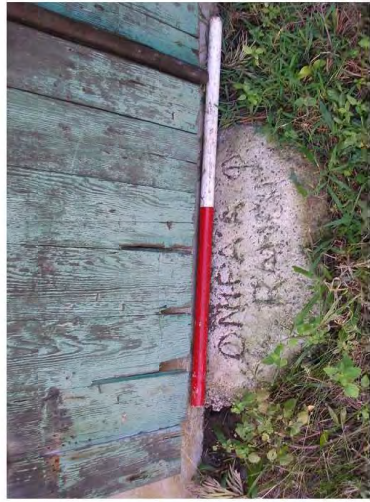
Figure 136. SIFP Site 29507 Feature B, west side of the building, view to the northeast.
