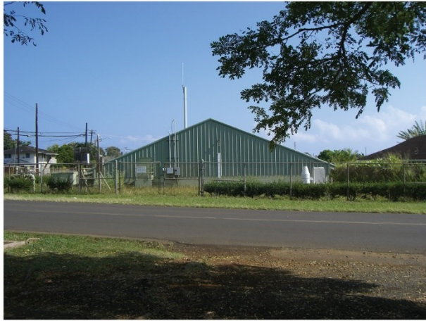
Ornellas Tank Site - Existing tank.
