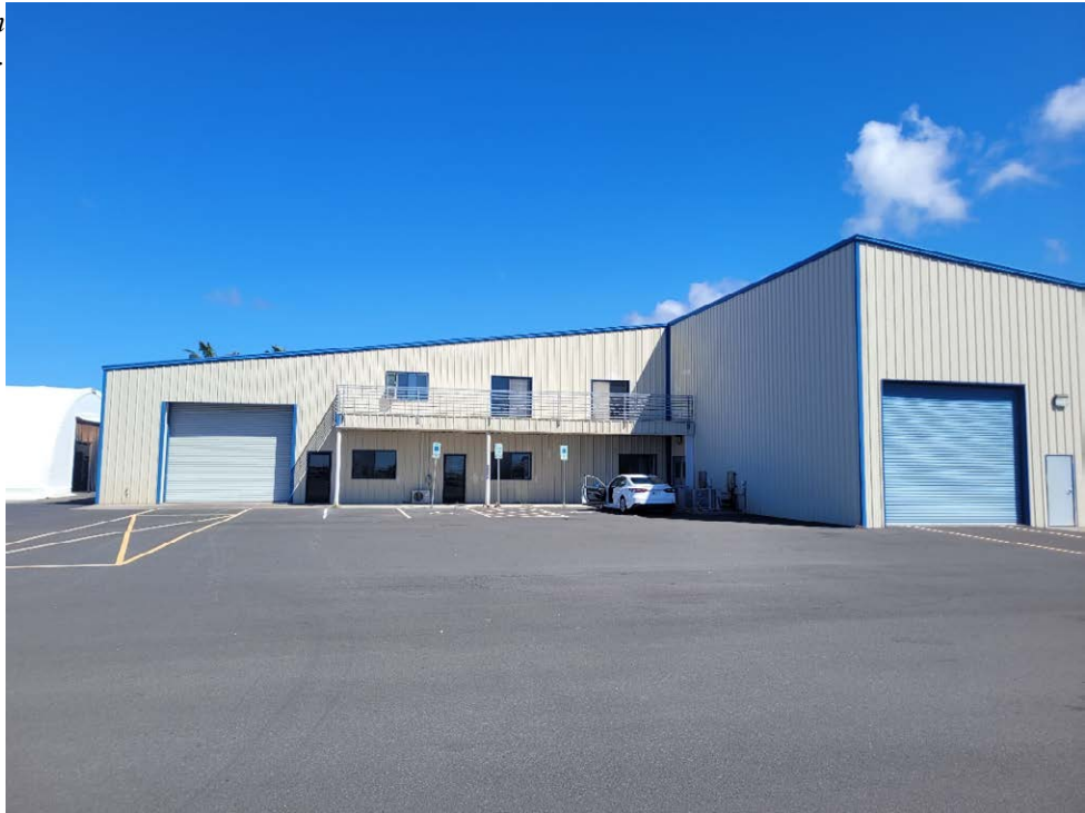
a. Exterior of site (south side).
