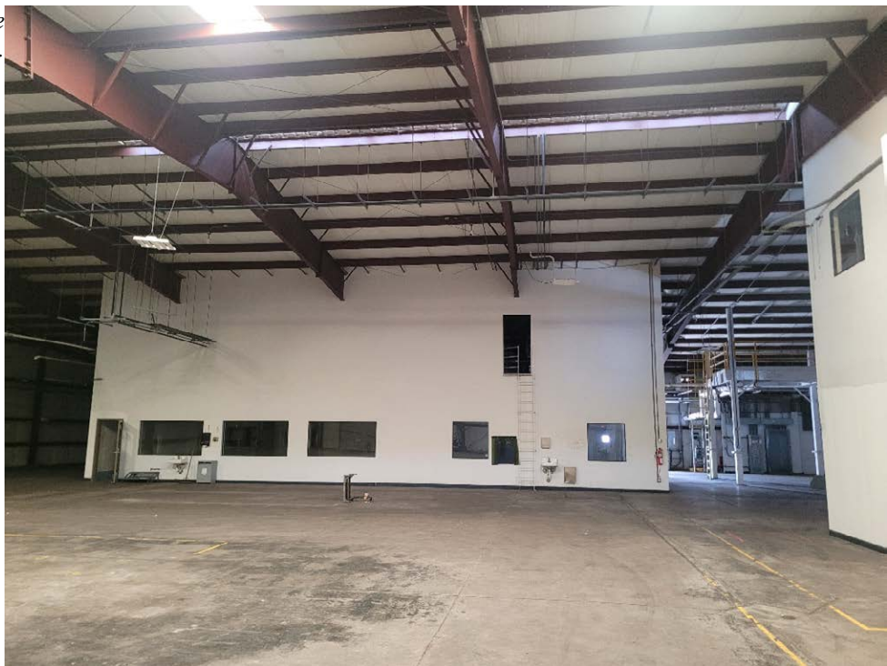
b. View of warehouse interior.
