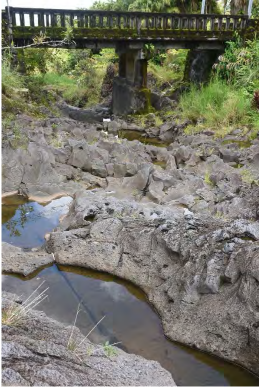
Fig. 27. Ulaino Stream bridge, 645 ft., looking downstream toward span.
