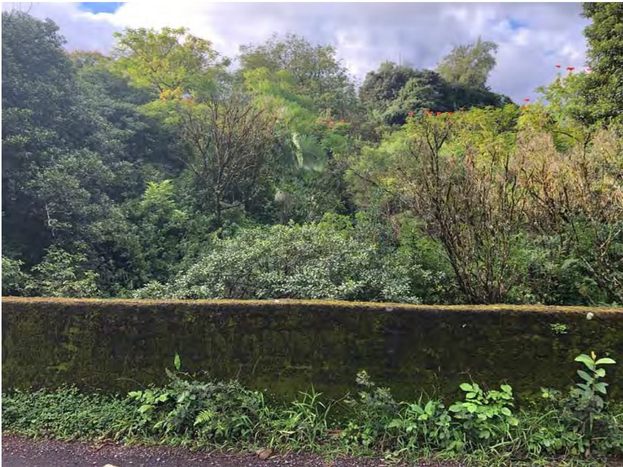
Figure 18. 'Ula'ino Bridge view upstream showing dense forest.
