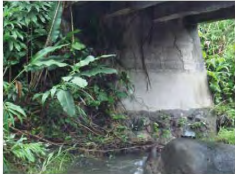
Concrete abutment, Kahului side Courtesy of NOEI
