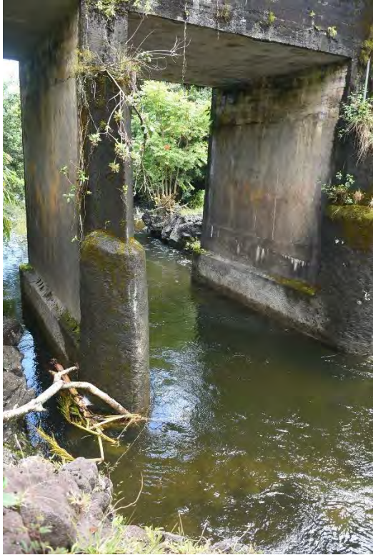
Fig. 35. Mokulehua Stream bridge, 525 ft., downstream beneath span.
