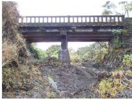
Ulaino Stream Bridge upstream elevation Courtesy of NOEI
