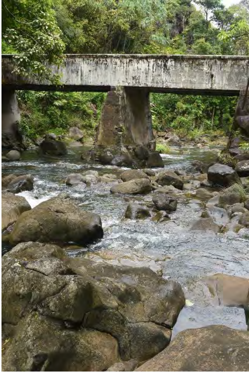
Fig. 15. Puohokamoa Stream bridge, 575 ft., looking downstream toward span.
