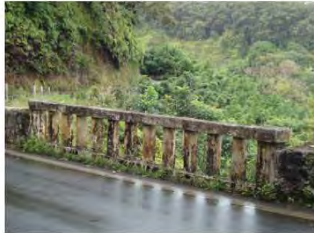
Concrete open vertical railing, downstream side Courtesy of FAI
