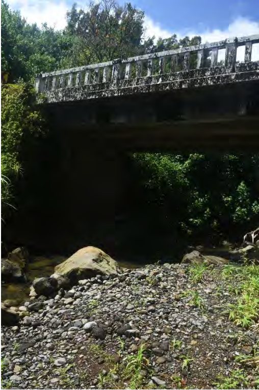
Fig. 7. Kailua Stream bridge, 685 ft., looking upstream at span.
