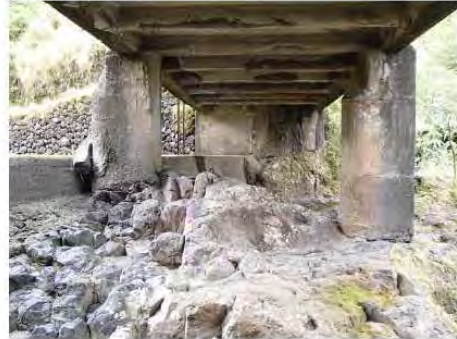
Concrete girders Courtesy of NOEI
