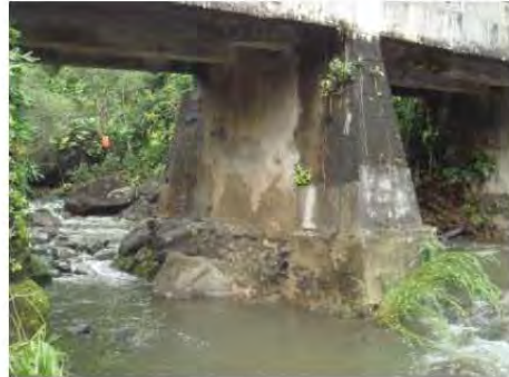
Concrete pier wall with CRM base Courtesy of NOEI
