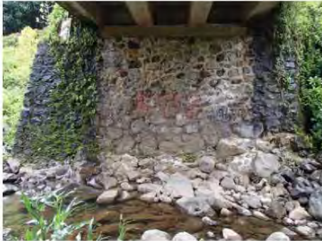
CRM abutment, Hana side Courtesy of NOEI
