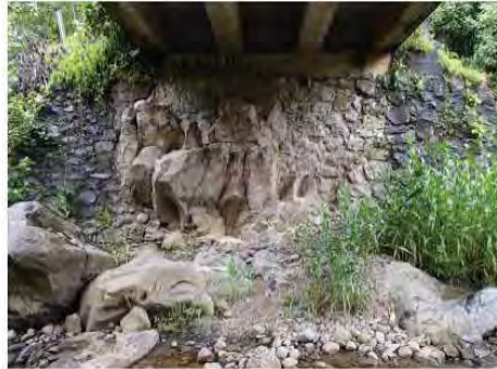
CRM abutment set upon natural rock, Kahului side Courtesy of NOEI
