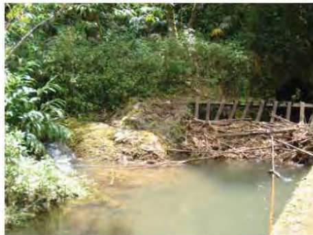
Detail of EMI engineering system Courtesy of FAI
