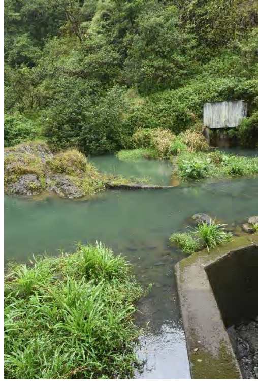
Fig. 20. Kopiliula Stream, 1280 ft, looking west from span across diversion works.
