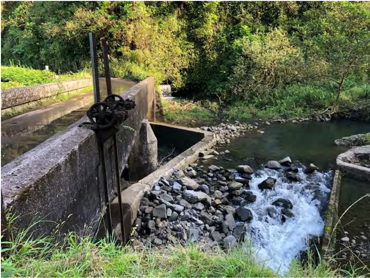
Figure 14. Kōpili'ula Bridge showing a stream diversion.
