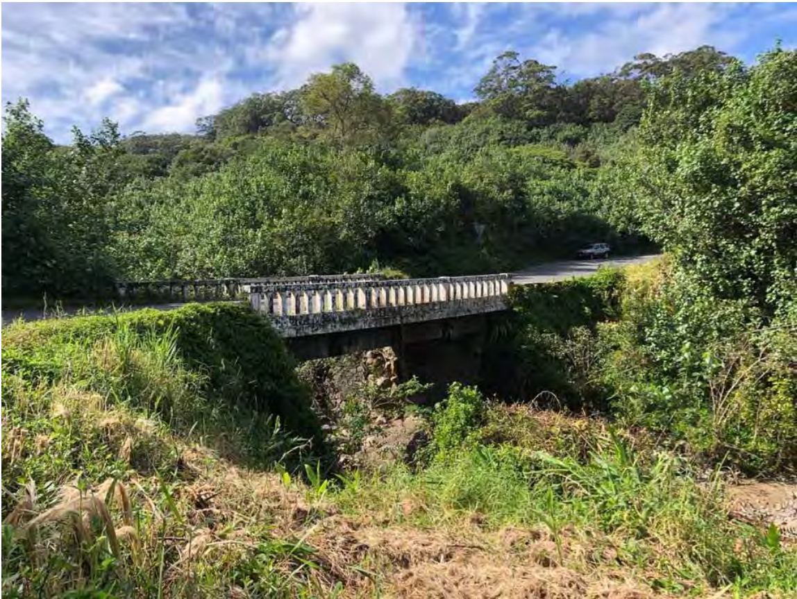
Figure 2. Kailua Bridge showing dense forest growth.
