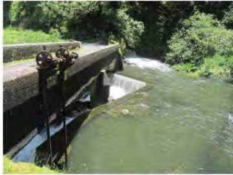
Setting of the Kopiulu Stream Bridge, upstream side Courtesy of FAI
