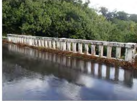
Concrete open vertical railing, downstream side Courtesy of NOEI
