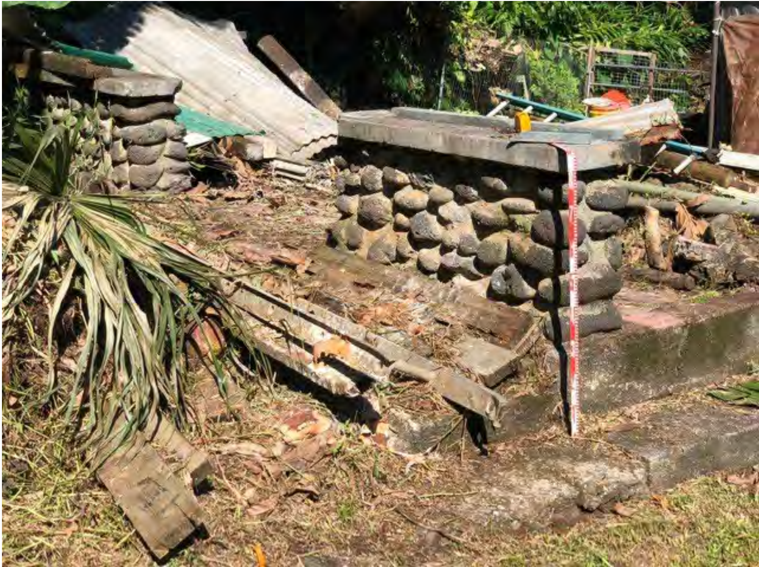
Figure 33: Photograph of Site TS-1. View to Northwest.
