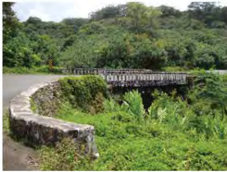
Setting of Kailua Stream Bridge Courtesy of FAI
