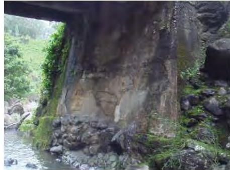
Concrete abutment, Hana side Courtesy of NOEI
