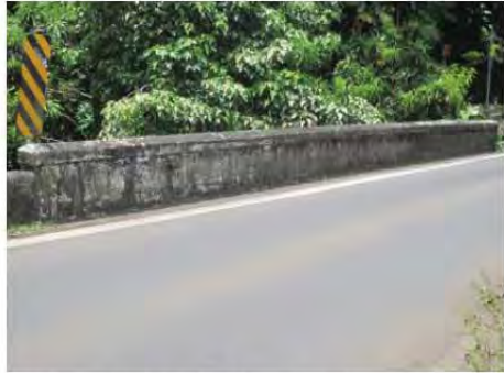
Solid concrete parapet with saddle coping, upstream side Courtesy of NOEI
