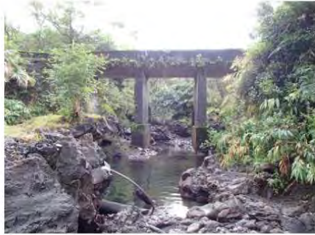
Mokulehua Stream Bridge piers downstream elevation Courtesy of NOEI
