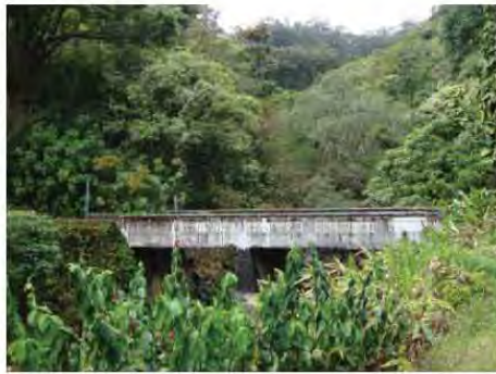
Setting of Puohokamoa Stream Bridge Courtesy of FAI
