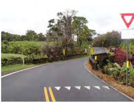
Hana approach to Ulaino Stream Bridge toward Kahului Courtesy of NOEI
