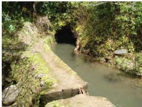
Detail of EMI engineering system, tunnel toward Hana side Courtesy of FAI
