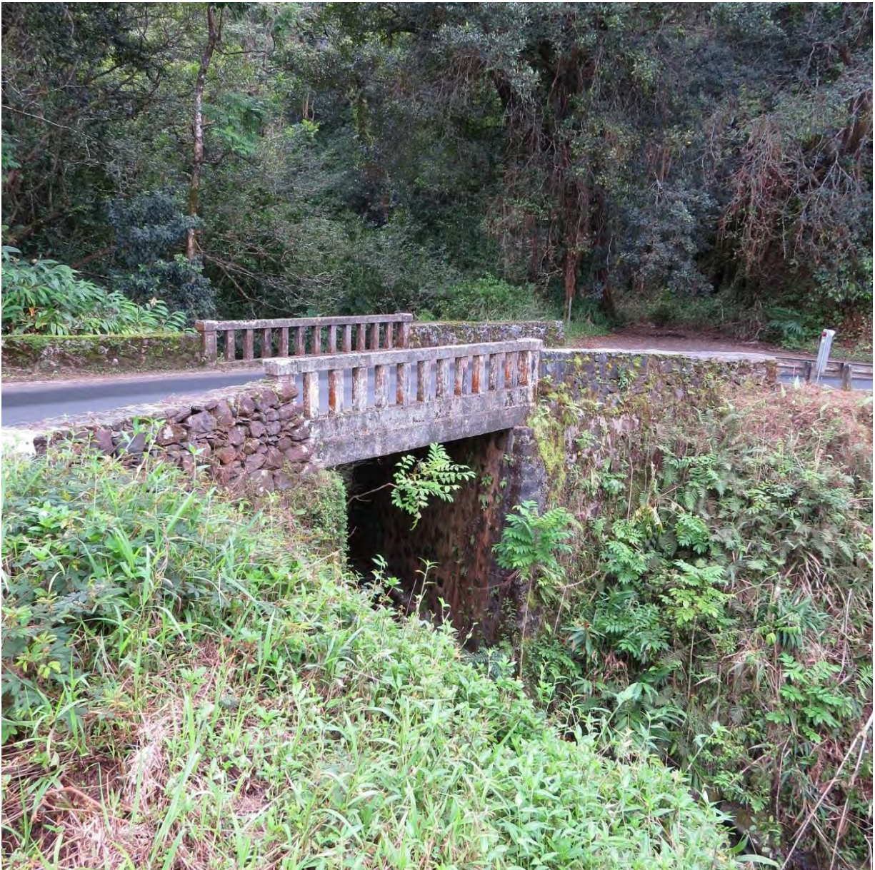
Figure 6. Makanali Bridge showing dense forest and steep terrain.
