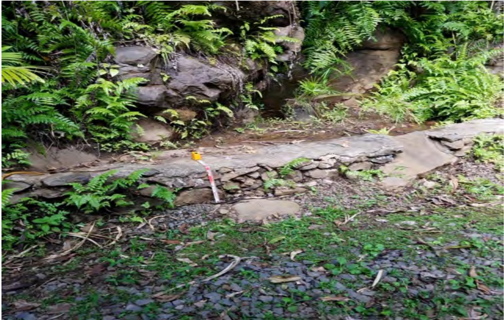
Figure 44: Photograph of Puohokamoa Bridge Site Illustration, Feature 2. View to East.
