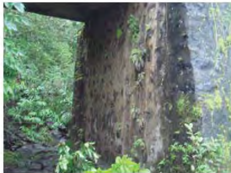
CRM abutment, Kahului side Courtesy of NOEI
