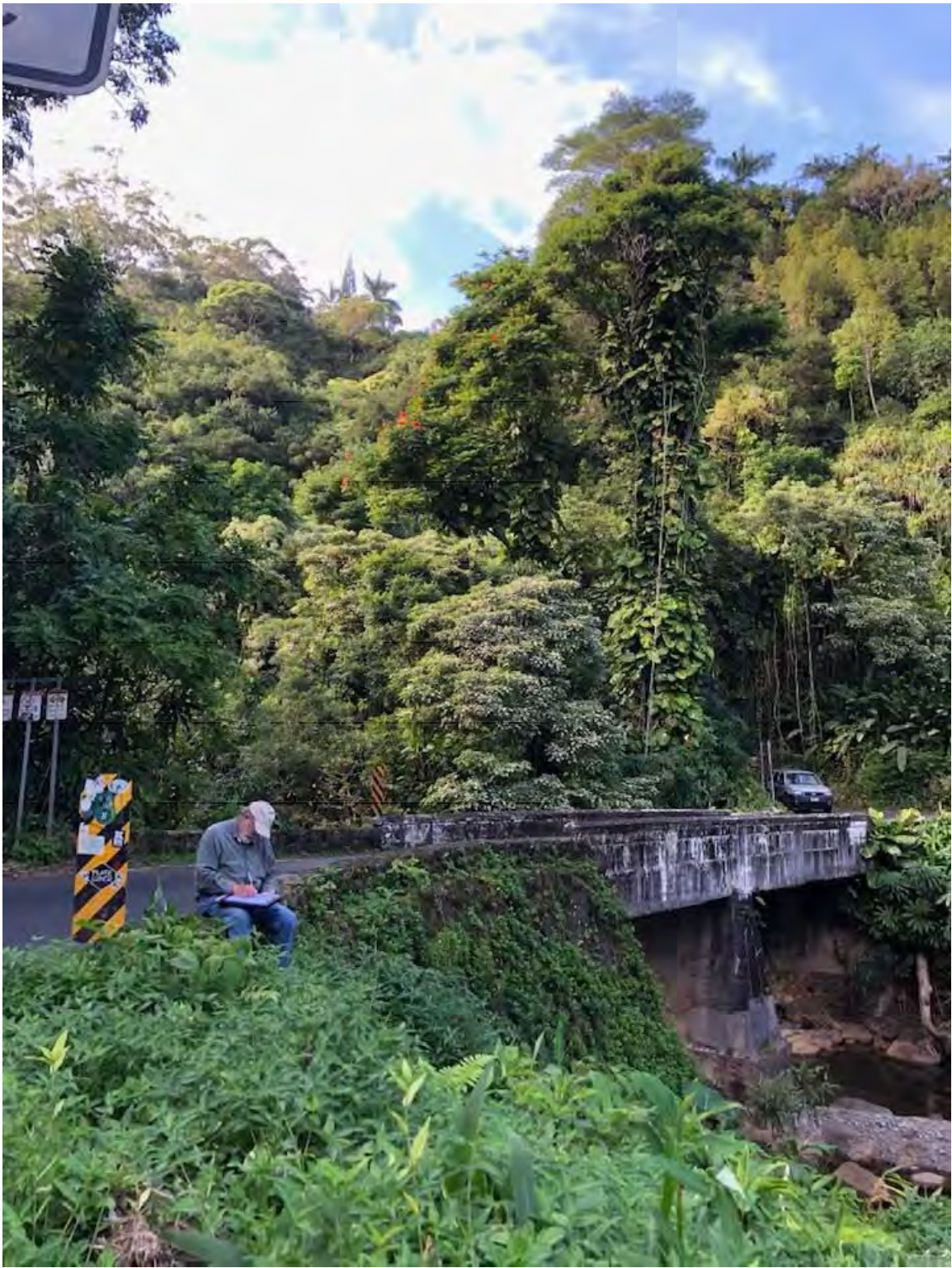
Figure 10. Puohokamo Bridge showing dense forest growth.
