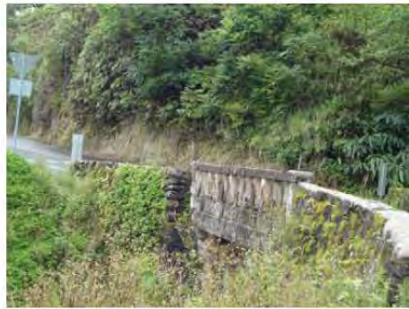
Makanali Stream Bridge downstream elevation Courtesy of FAI
