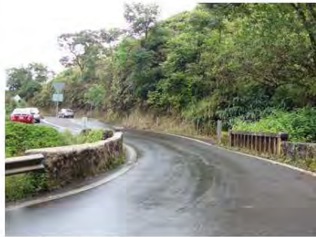
Kahului approach to Makanali Stream Bridge toward Hana Courtesy of FAI
