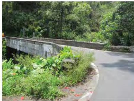
Kahului approach to Puohokamoa Stream Bridge toward Hana Courtesy of NOEI
