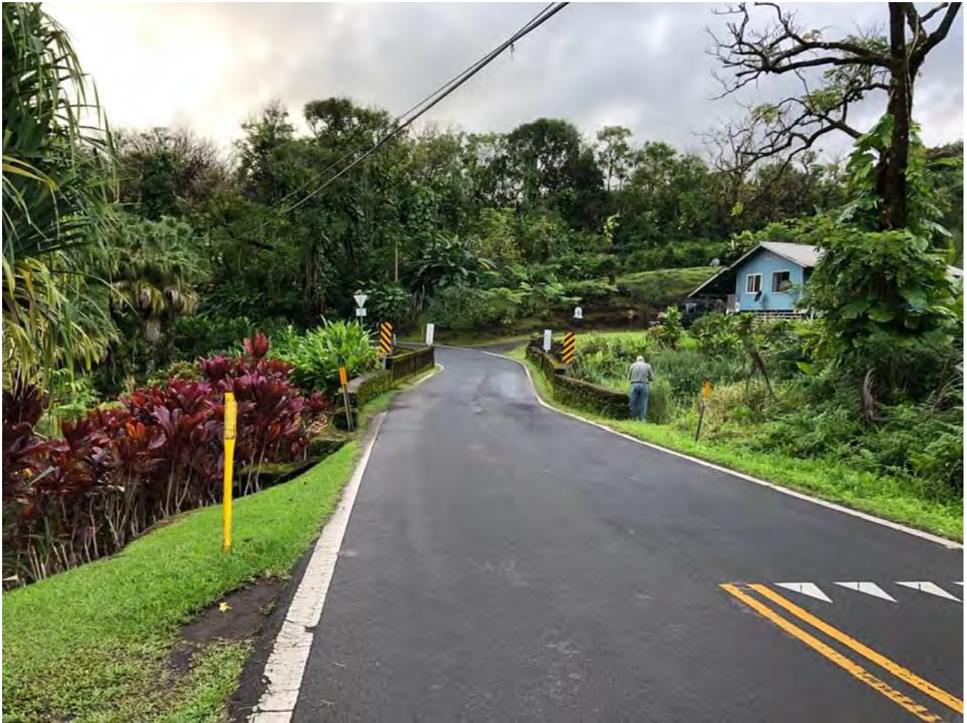
Figure 22. Mokulehua Bridge showing adjacent properties with ornamental vegetation.
