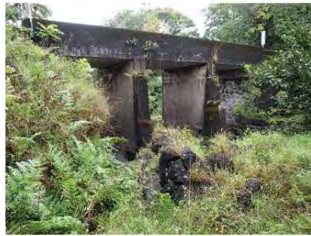
Mokulehua Stream Bridge upstream elevation Courtesy of NOEI
