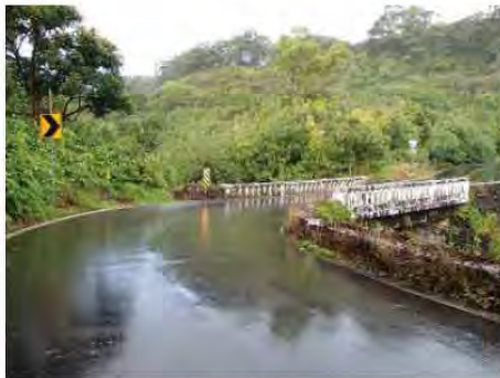
Hana approach to Kailua Stream Bridge toward Kahului Courtesy of NOE1
