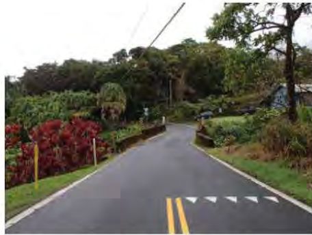
Kahului approach to Ulaino Stream Bridge toward Hana Courtesy of NOEI
