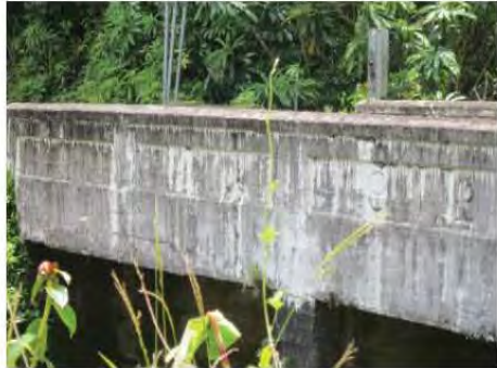
Puohokamaa Stream Bridge downstream elevation with inscription Courtesy of FAI
