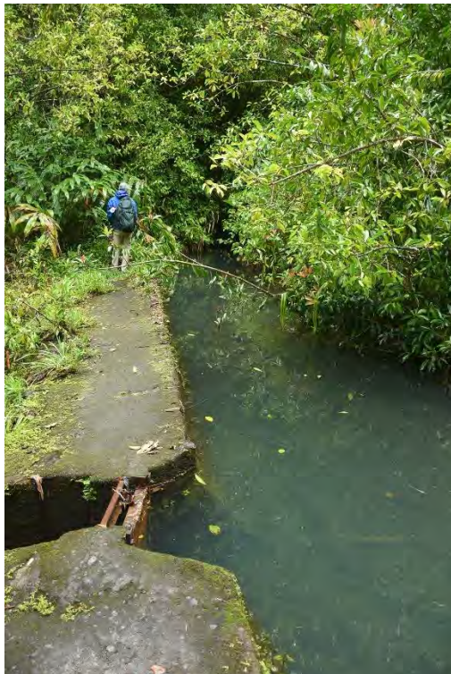
Fig. 13. Makanali Stream, 700ft., diversion wier and pool upstream from bridge.
