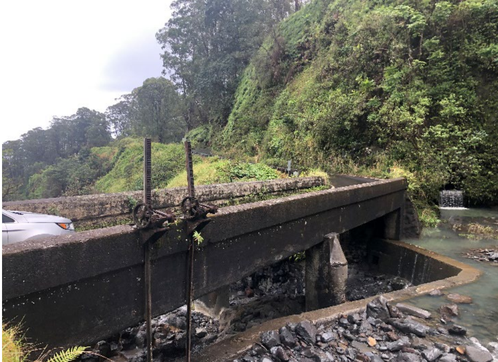
Photo 3-4. Bridge #19—Kopiliula Stream Bridge crossing the Kopiliula Stream (looking downstream from the mauka side of the bridge—Note East Maui Irrigation Co. sluice gate and weir)
