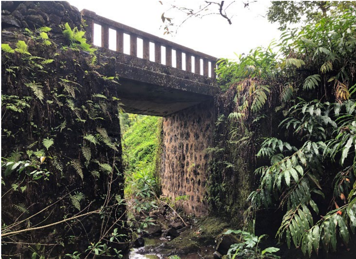
Photo 3-2. Bridge #5—Makanali Stream Bridge crossing the Makanali Stream (looking downstream from the mauka side of the bridge)
