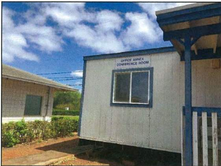
Photograph 6: Front view of Building No. 15 (annex building) located on the south portion of the Subject Property.
