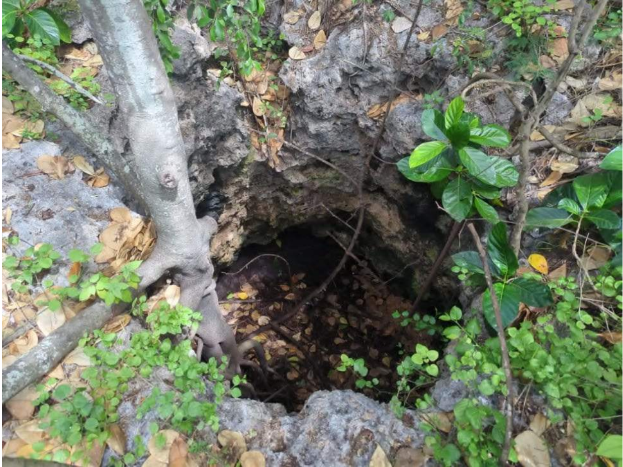
Figure 22. Honua 5, sinkhole (plan view)
