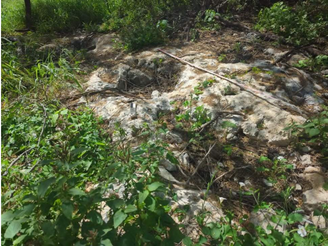
Figure 25. Honua 17, filled sinkholes, facing south
