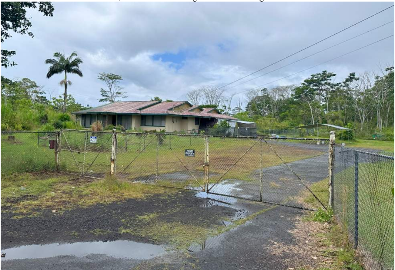
▼ 2h. Alt. 3, home and clearing on Pahoa Village Road
