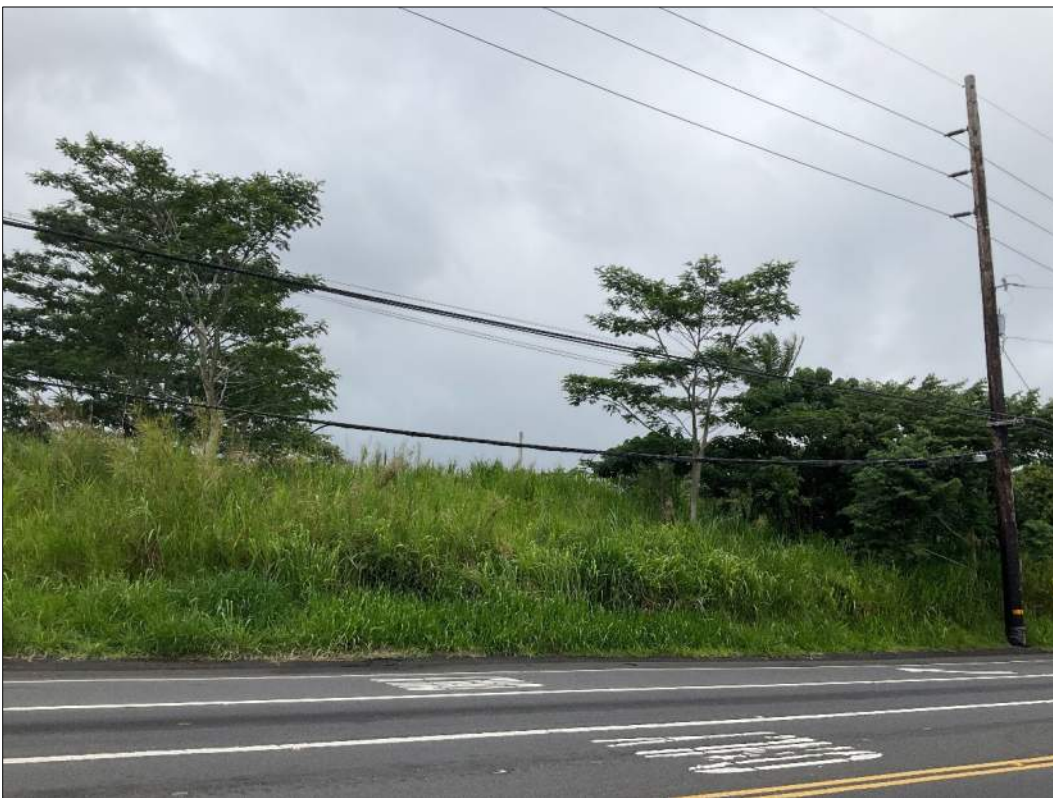
Figure 7. View of the eastern boundary of Alternative 1 with Pāhoa Village Road (foreground), view to the west.
