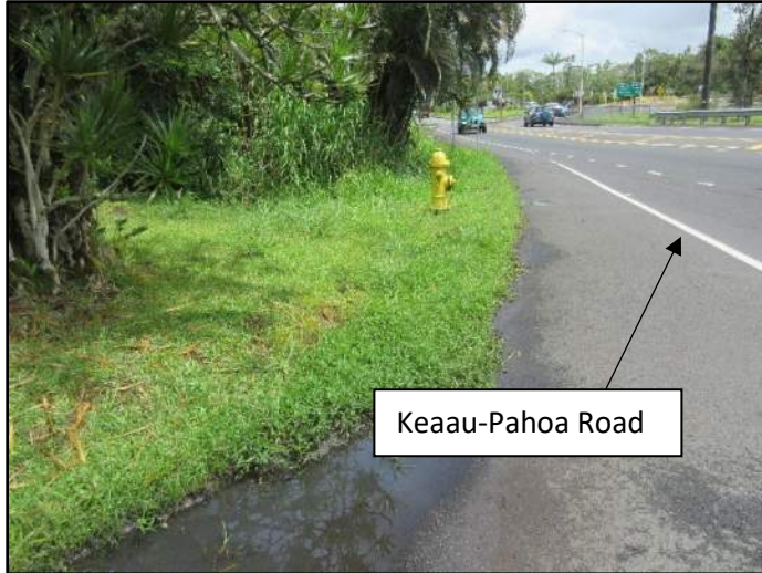
Photograph 16. A view of the fire hydrant located to the east of parcel 007 bordering Keaau-Pahoia Road (31 May 2023).
