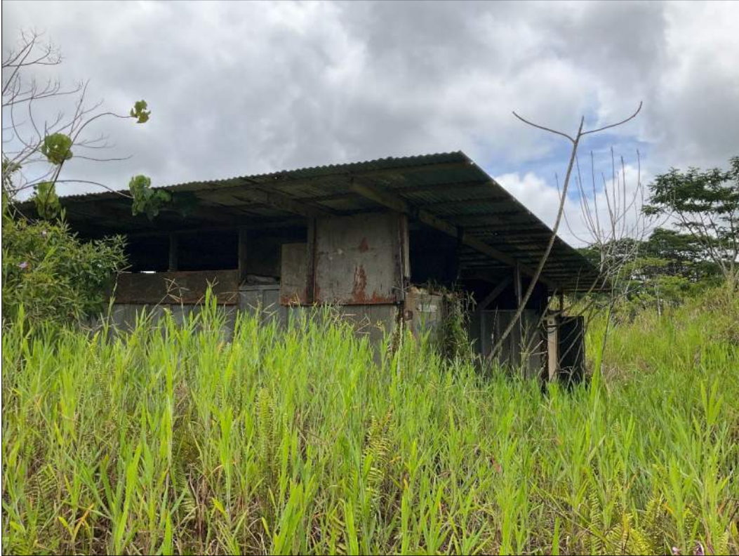
Figure 13. View of wooden shed located on the northwest corner of parcel 004, view to the northeast.
