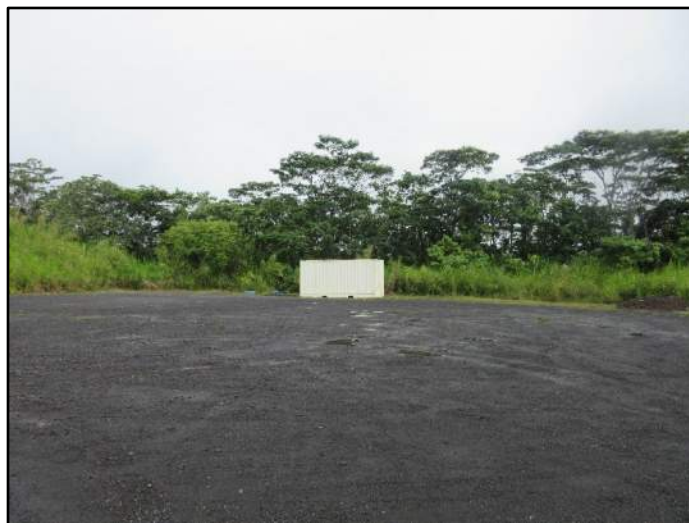
Photograph 3. A view of the metal container located in the parking lot at parcel 007 (31 May 2023).
