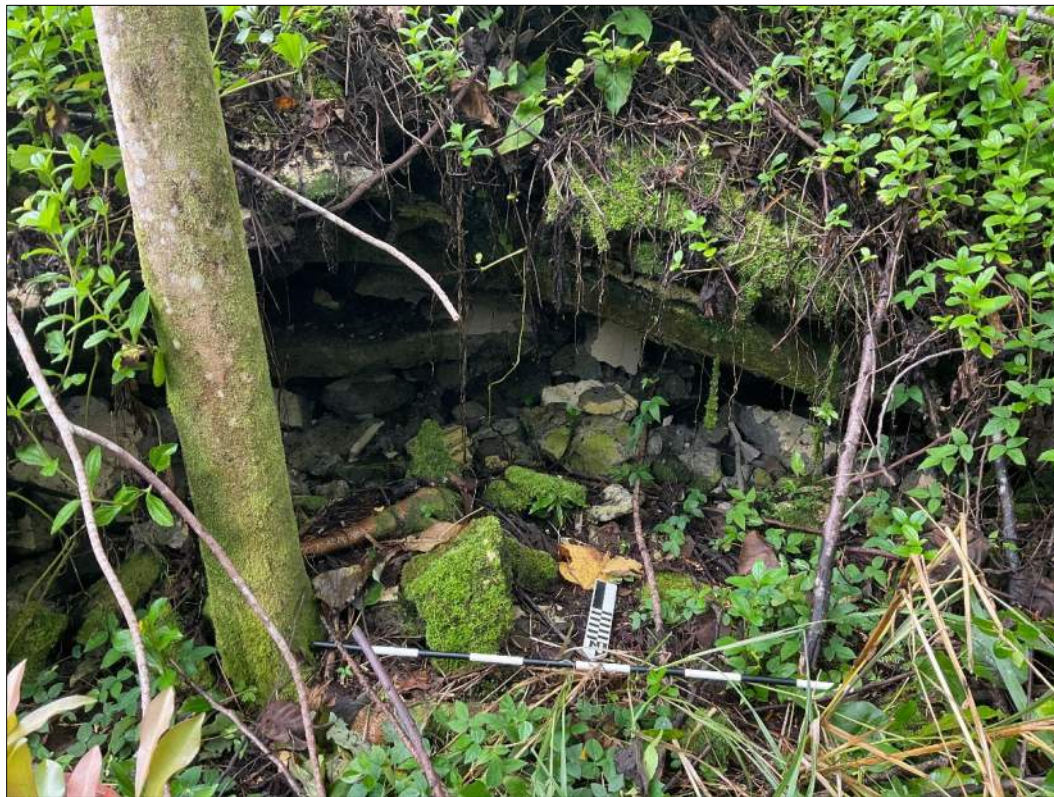
Figure 29. Concrete and rebar pile located along the northern boundary of TMK parcel 082 within the Alternative 3 study area, view to the southwest.
