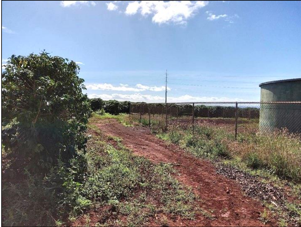
Figure 14. Photograph of the southern boundary of the proposed project area, bordering the Lima Ola Subdivision’s existing water storage tank (view to southeast).
