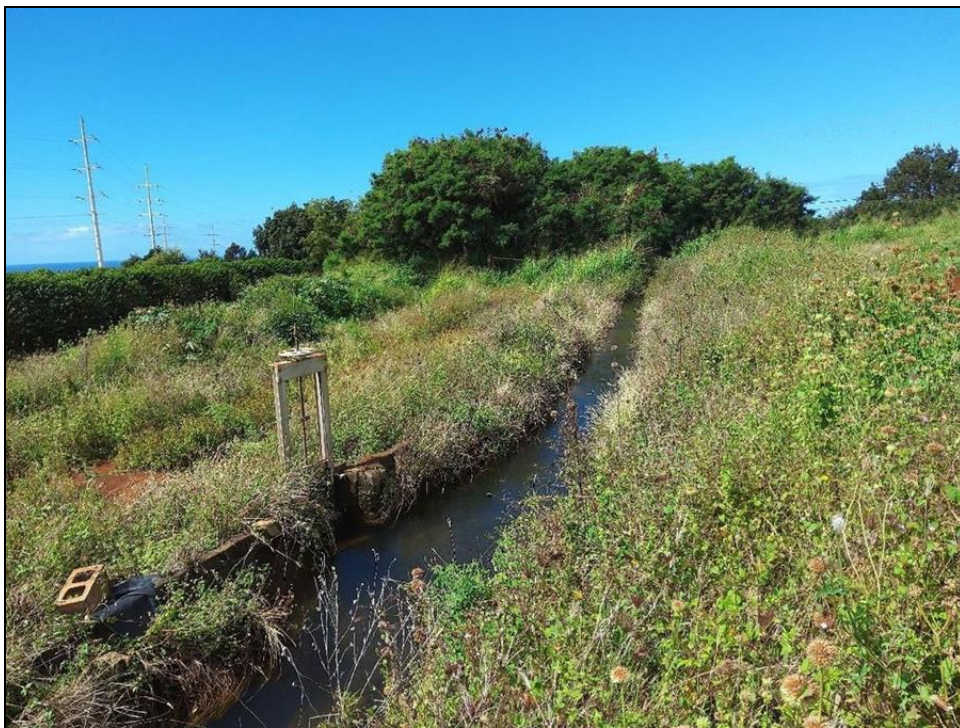
Figure 19. Photograph of a concrete water ditch (SIHP 50-30-09-00689) located on the south side of the current water storage tank, outside of the proposed project area (view to west).
