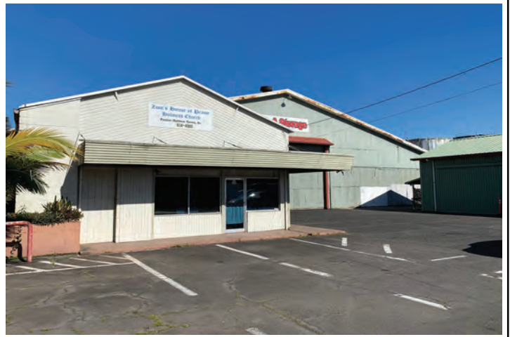
Photo 20. View of Buildings Present at Parcel 2
