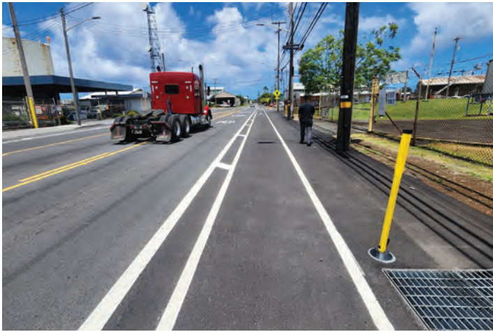
Photo 15. View of Kalaniana'ole Street Eastbound Past Kumau Street (May 2023 Photo)
