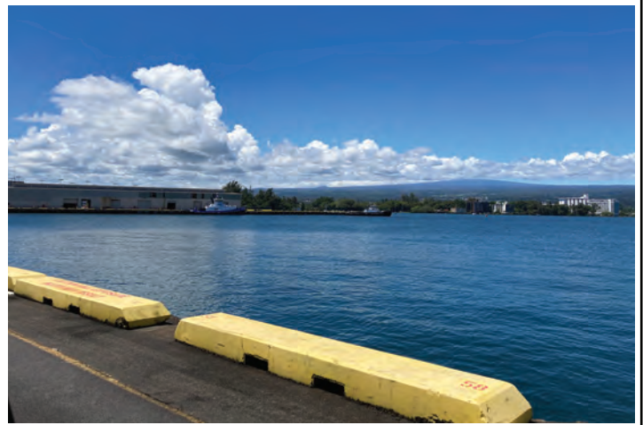
Photo 04. View of Pier 2 and Associated Building
