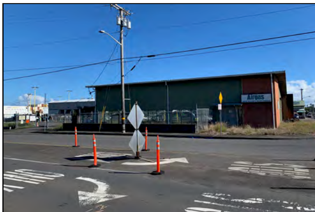
Exhibit 1-10. Photo of AirGas Gaspro, Inc. Site
