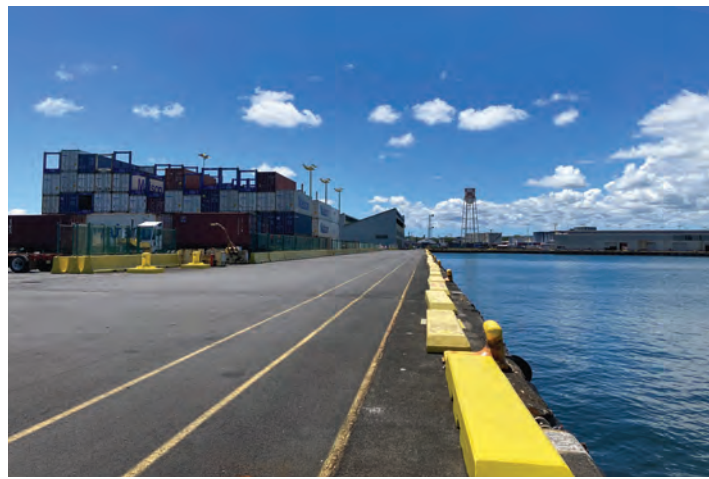
Photo 03. View of Pier 1
