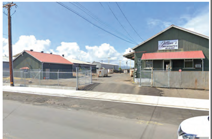
Photo 22. View of Parcel 3 (2-1-7-046) Buildings
