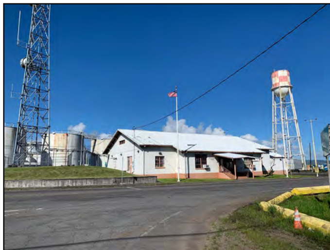
Exhibit 1-16. Water Tower Near U.S. Customs Building
