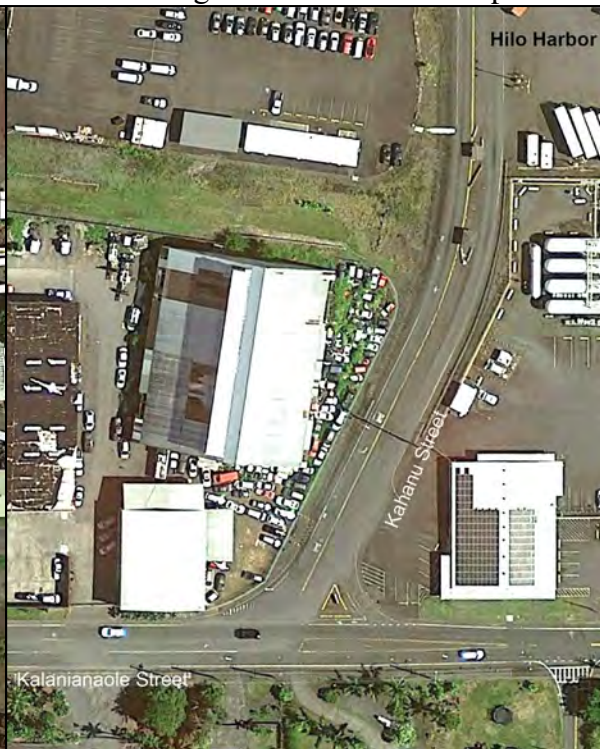
Exhibit 1-8. Aerial View of Kahanu Street
