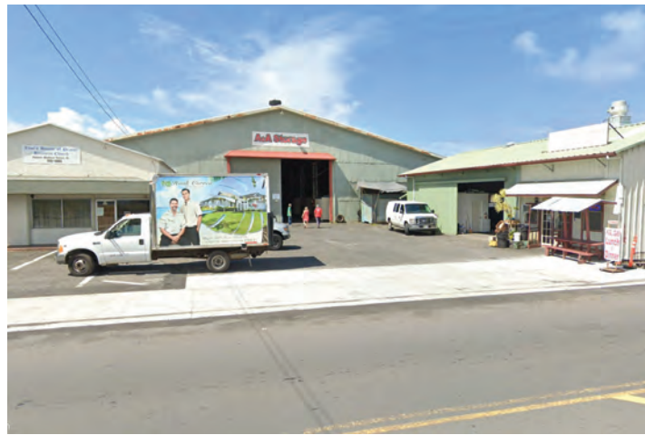
Photo 19. View of Parcel 2 (2-1-7-004) Buildings at Entrance
