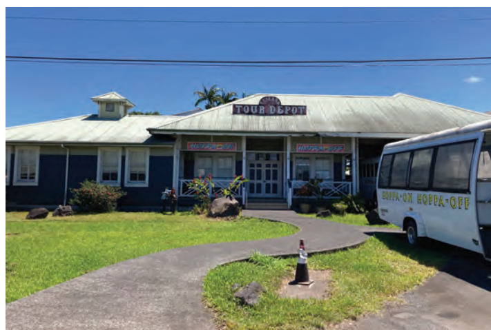
Photo 27. View of Other Buildings on Parcel 4
