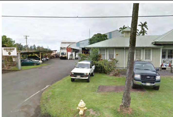
Photo 25. View Parcel 4 Driveway Entrance Along Kuhio Street
