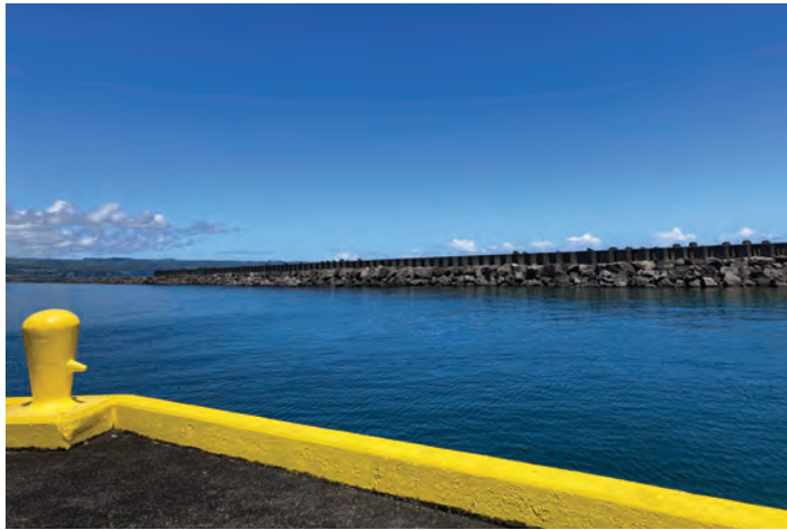
Photo 01. View of Hilo Breakwater
