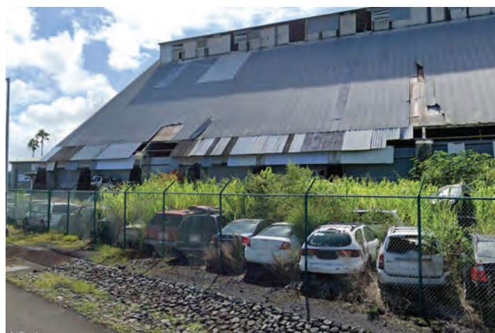
Photo 28. View of Parcel 5 (2-1-9-003) Building Along Kahanu Street
