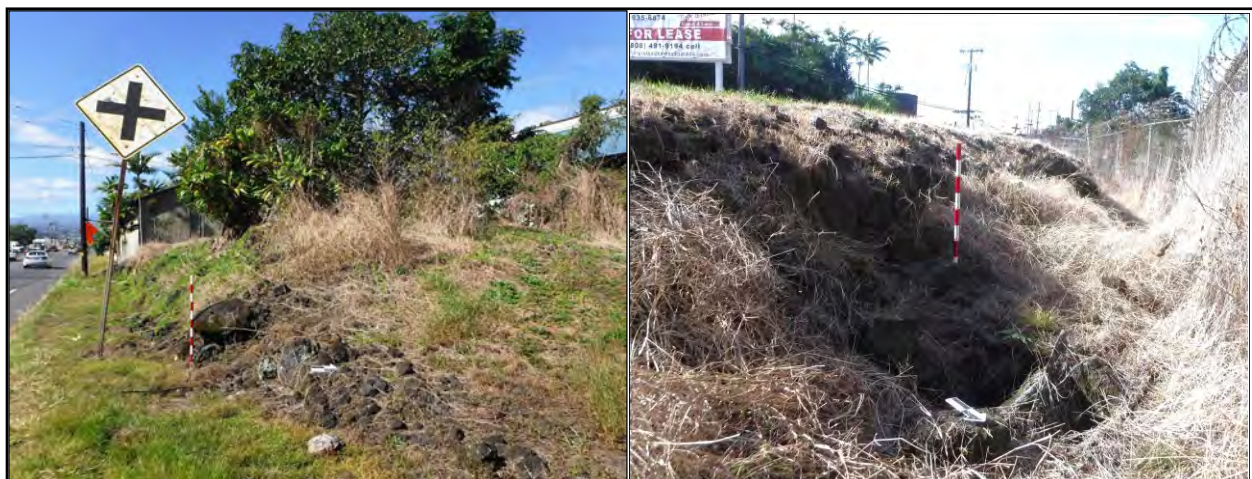
Exhibit 4-2. Photo of First Small Hill on Parcel 4
