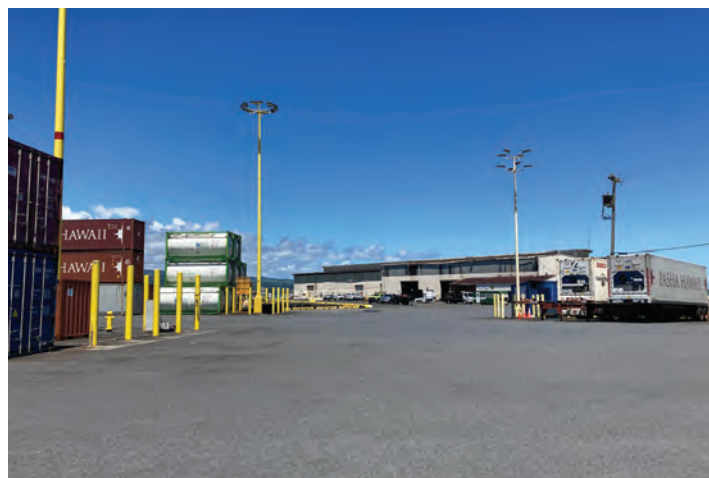
Photo 05. View of Pier 3 Cargo Yard Area
