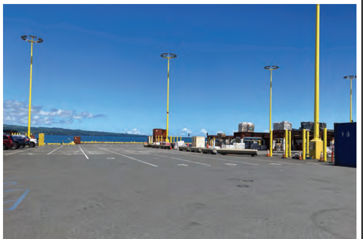
Photo 06. View of Pier 4 Cargo Yard Area
