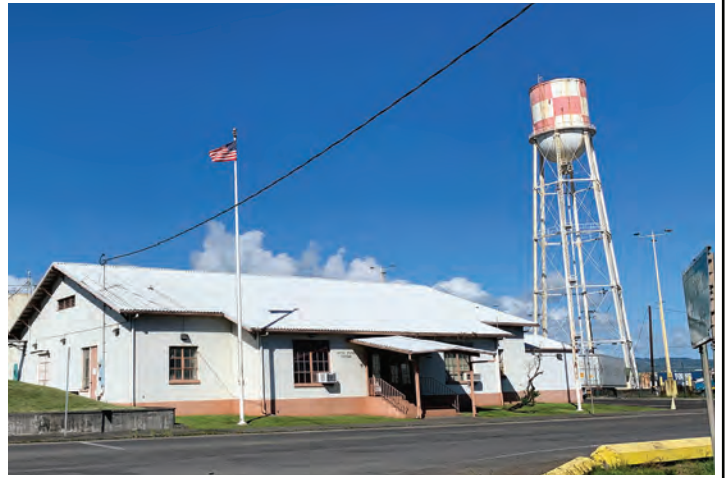
Photo 02. View of Water Tank Near U.S. Customs Building
