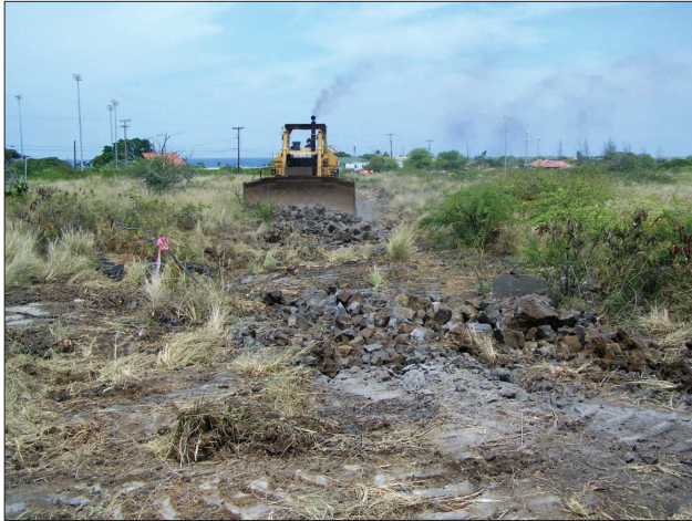
Figure 90. Bulldozer grading access road to drill sites (view north).
