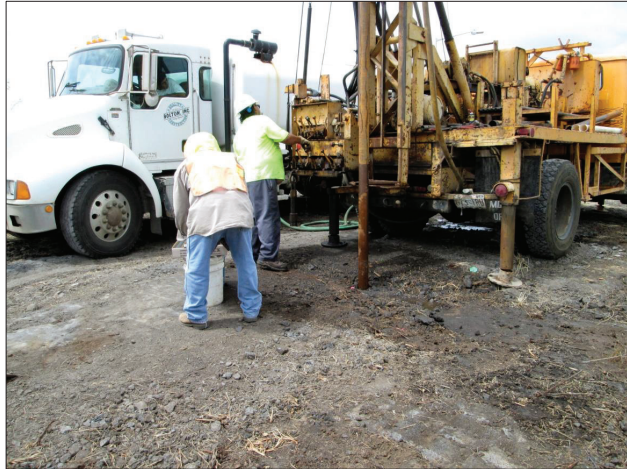
Figure 92. Drilling at bore hole B-2.
