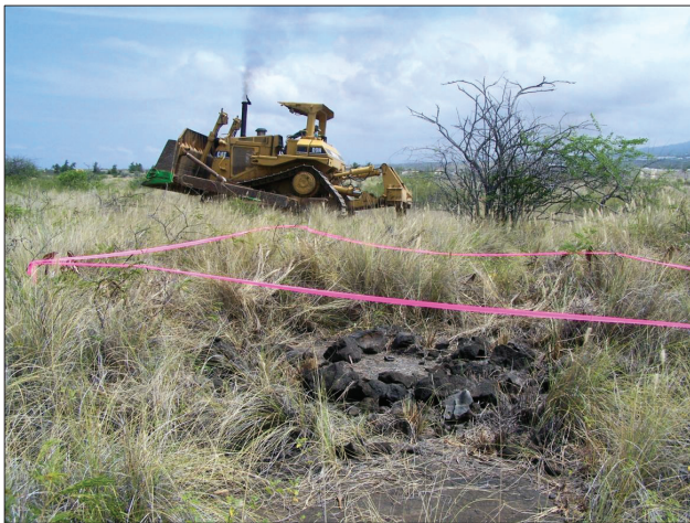
Figure 91. Bulldozer working between Sites 30212 (in foreground) and 30208 (view west).
