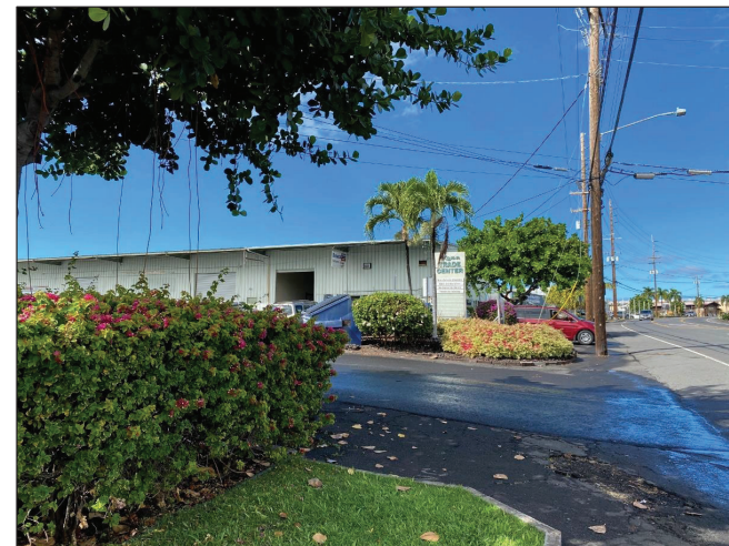
Figure 5. Photo 1: View of eastern perimeter of parcels along Kaiwi St., showing warehouse built on TMK (3) 7-4-010:010 (view to north-northwest).
