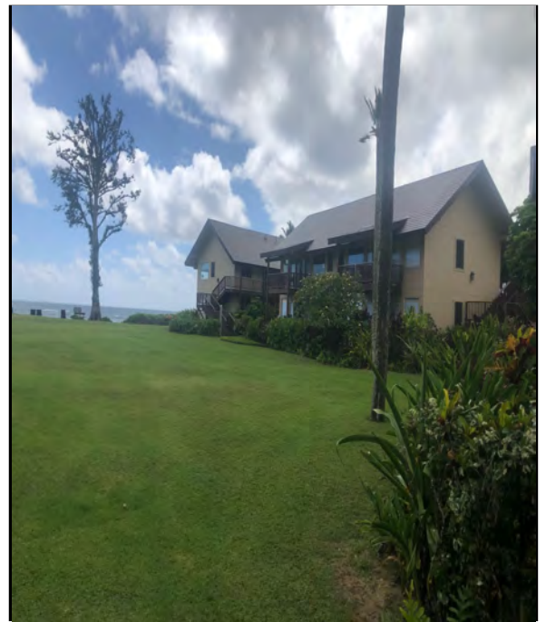
Photo 6: Southeast view of large lot A1, buildings E and F can be seen
