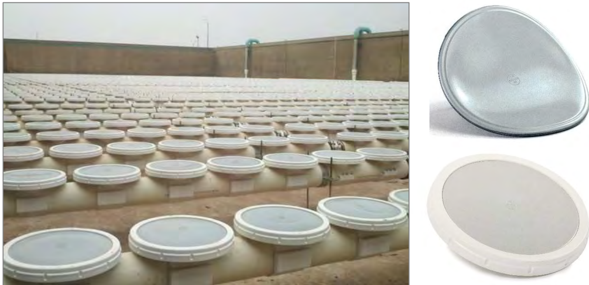
Figure 6: Example ECD Diffusers with PTFE Membranes
