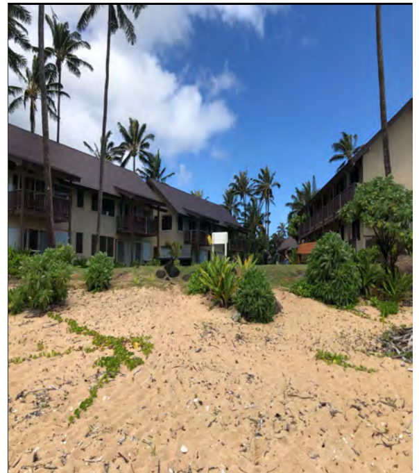
Photo 16: West facing view of smaller lot A2 showing buildings I, J, and K
