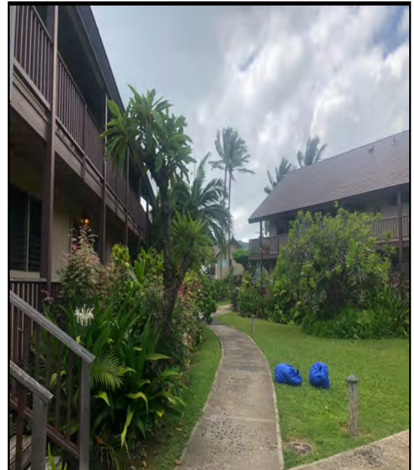
Photo 4: East view of walkway between buildings D and L
