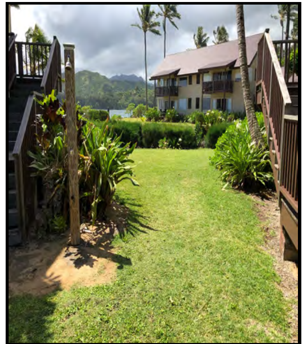
Photo 20: Southeast view of building I from between buildings G and H
