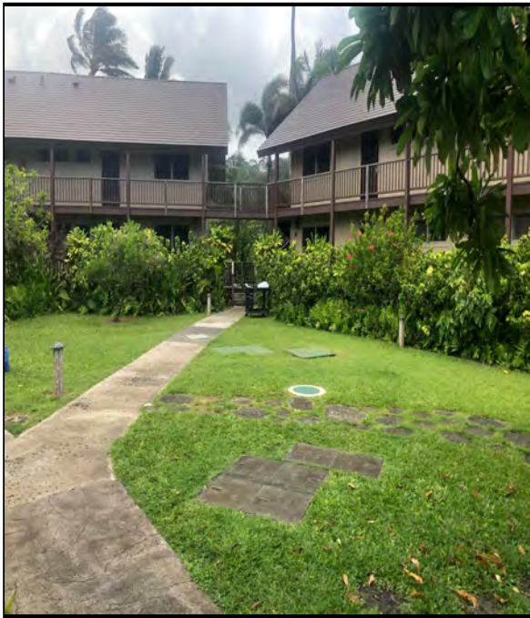
Photo 3: Southeast view of buildings M and L
