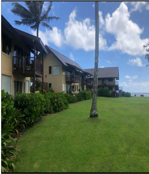
Photo 5: Northeast view of large lot A1, buildings C, B, and A can be seen
