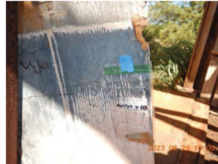
Photo 19 - 4011PKA-W-01A (Close-up) [BB\DSCN9838.JPG]
