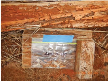
Photo 47 - 4011PKA-P-03 (Close-up) [BB\DSCN9802.JPG]
