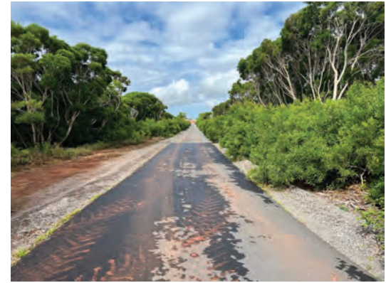
Picture 6. New access road at Site #4
