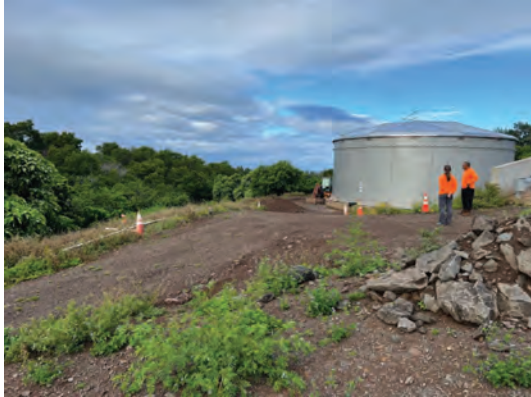
Picture 3. Site #1 water tanks and retaining wall to the right of tank.
