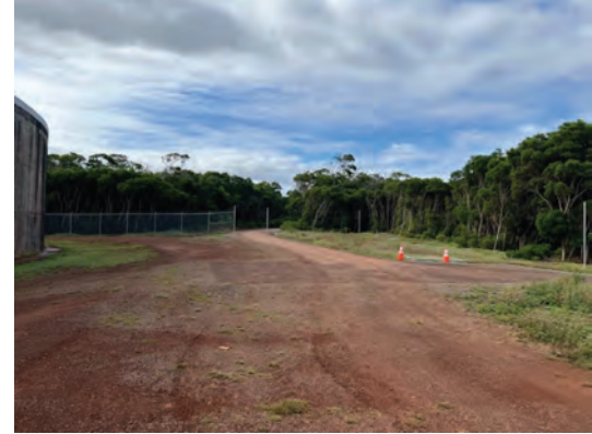
Picture 5. New 8-foot fenceline installation at Site #4
