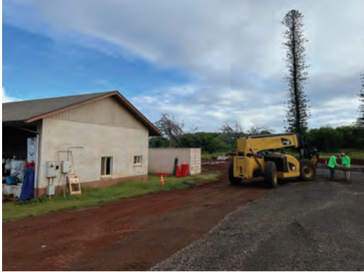
Picture 7. Maintenance Yard Site #7 with new gravel pad installed.
