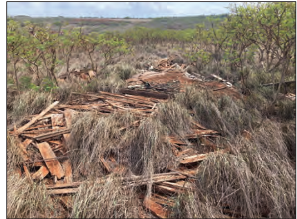
Figure 32. Photo F: View of collapsed structure in the 31.7-acre TMK: [2] 5-2-005:031 parcel, view to northeast
