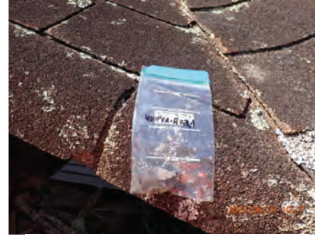
Photo 37 - 4011PKA-R-02A (Close-up) [JA\JA003578.JPG]
