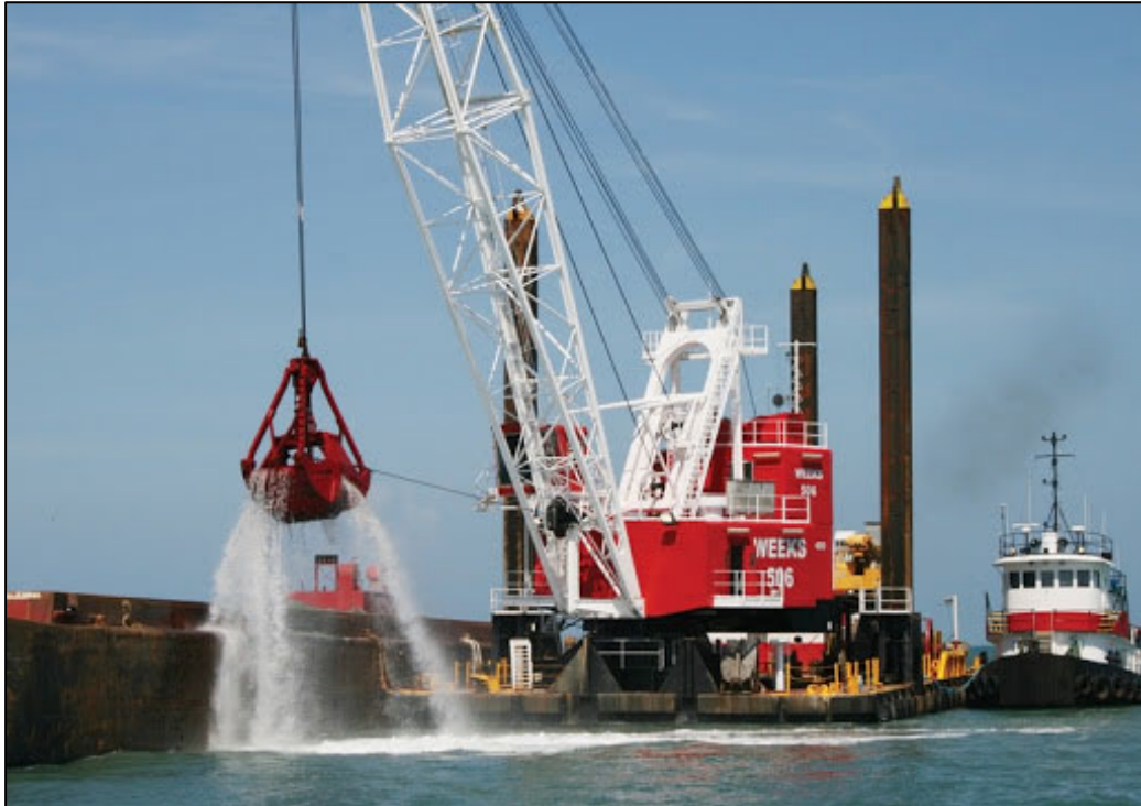
Figure 3-9 Example of clamshell dredging (IP Subsea)
