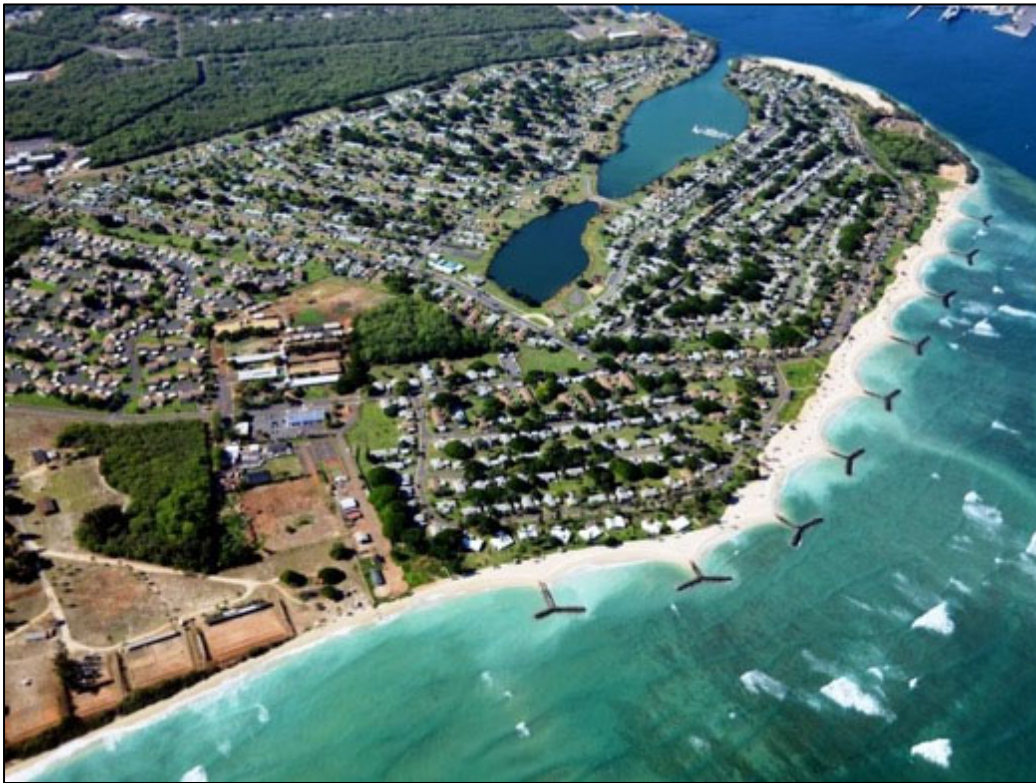
Figure 3-4 Beach nourishment with T-head groins at Iroquois Point, O'ahu
