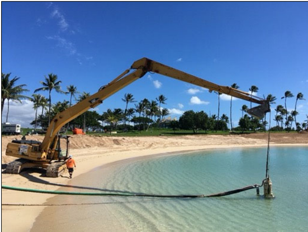
Figure 3-2 Sand pumping at Ko‘olina, O‘ahu (2017)
