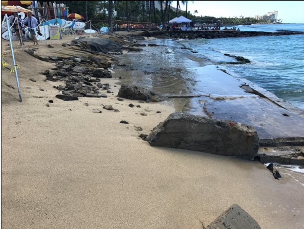
Figure 2-7 Conditions before construction of Kūhiō Sandbag Groin (Nov 2017)
