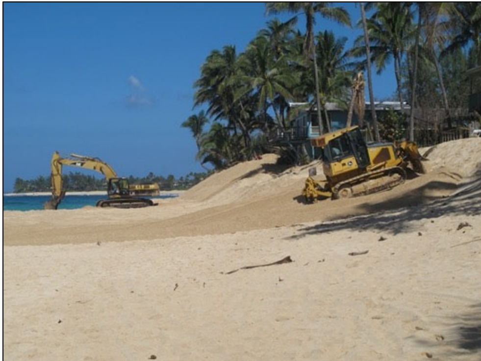
Figure 3-1 Sand pushing at Sunset Beach, O‘ahu (2014)
