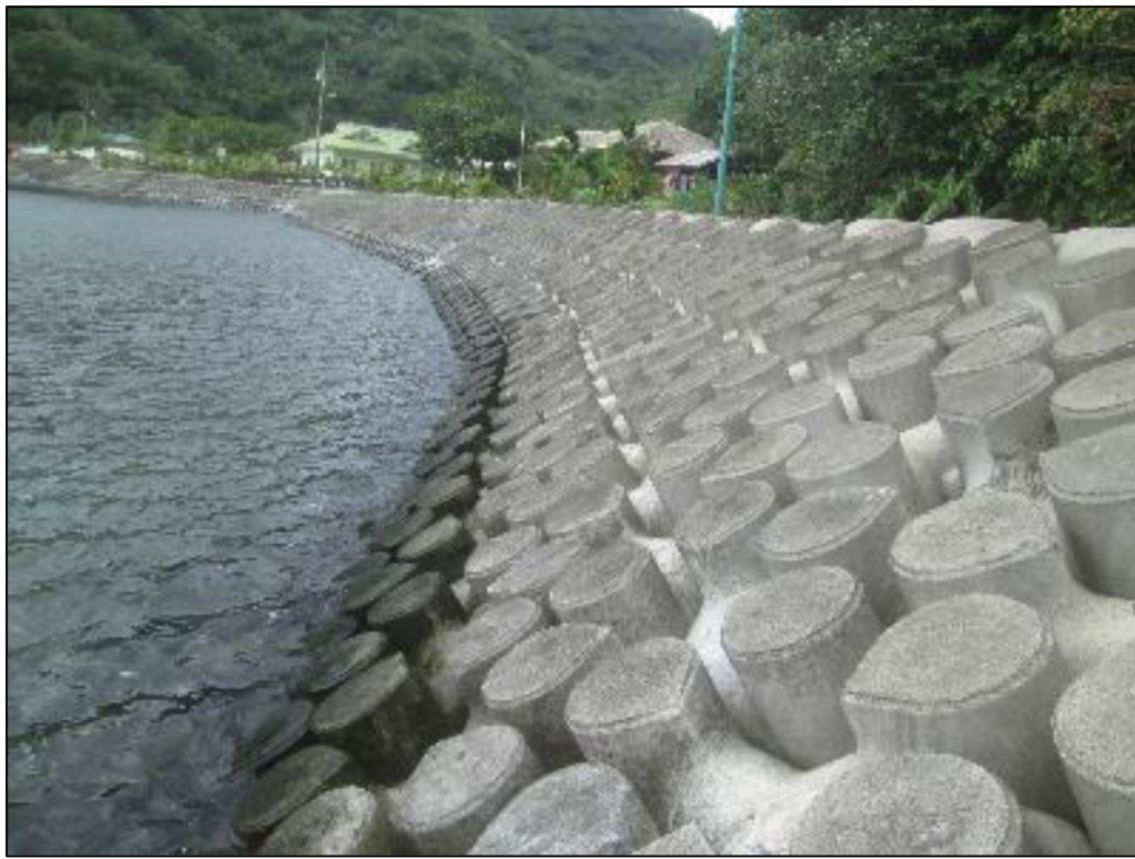
Figure 3-14 Tribar concrete armor units in American Samoa
