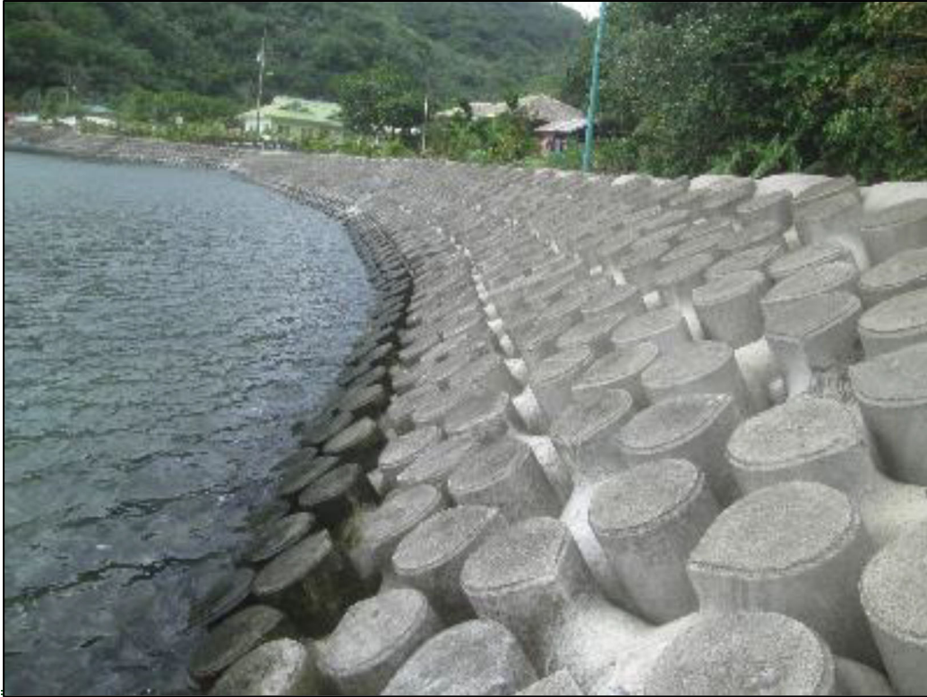
Figure 5-14 Tribar concrete armor units in American Samoa
