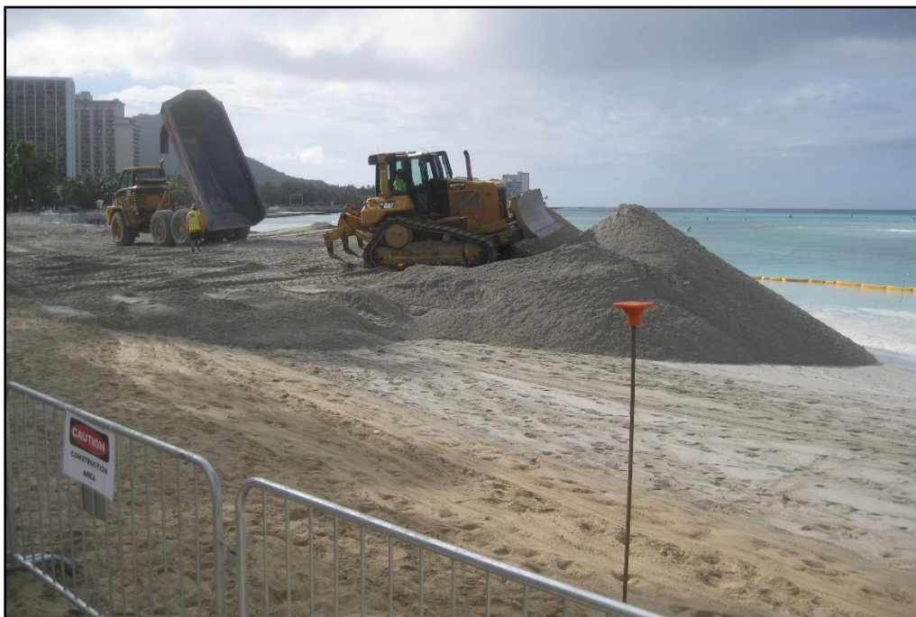
Figure 5-16 Sand placement, 2012 Waikiki Beach Maintenance Project.
