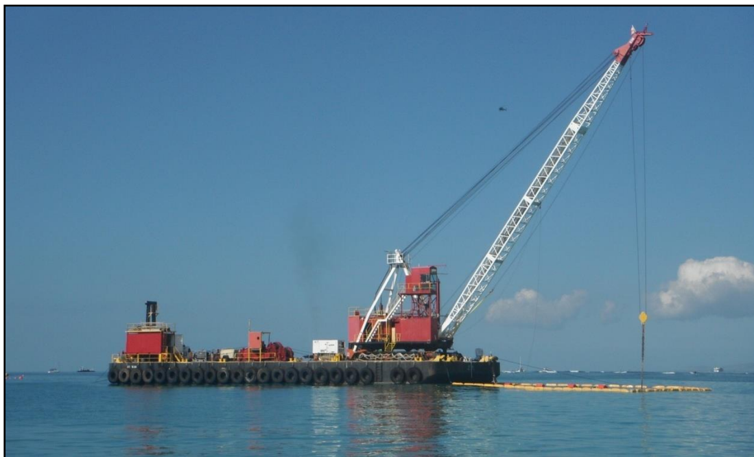
Figure 5-7 Healy Tibbitts Crane Barge used in the 2012 Waikiki Beach Maintenance Project
