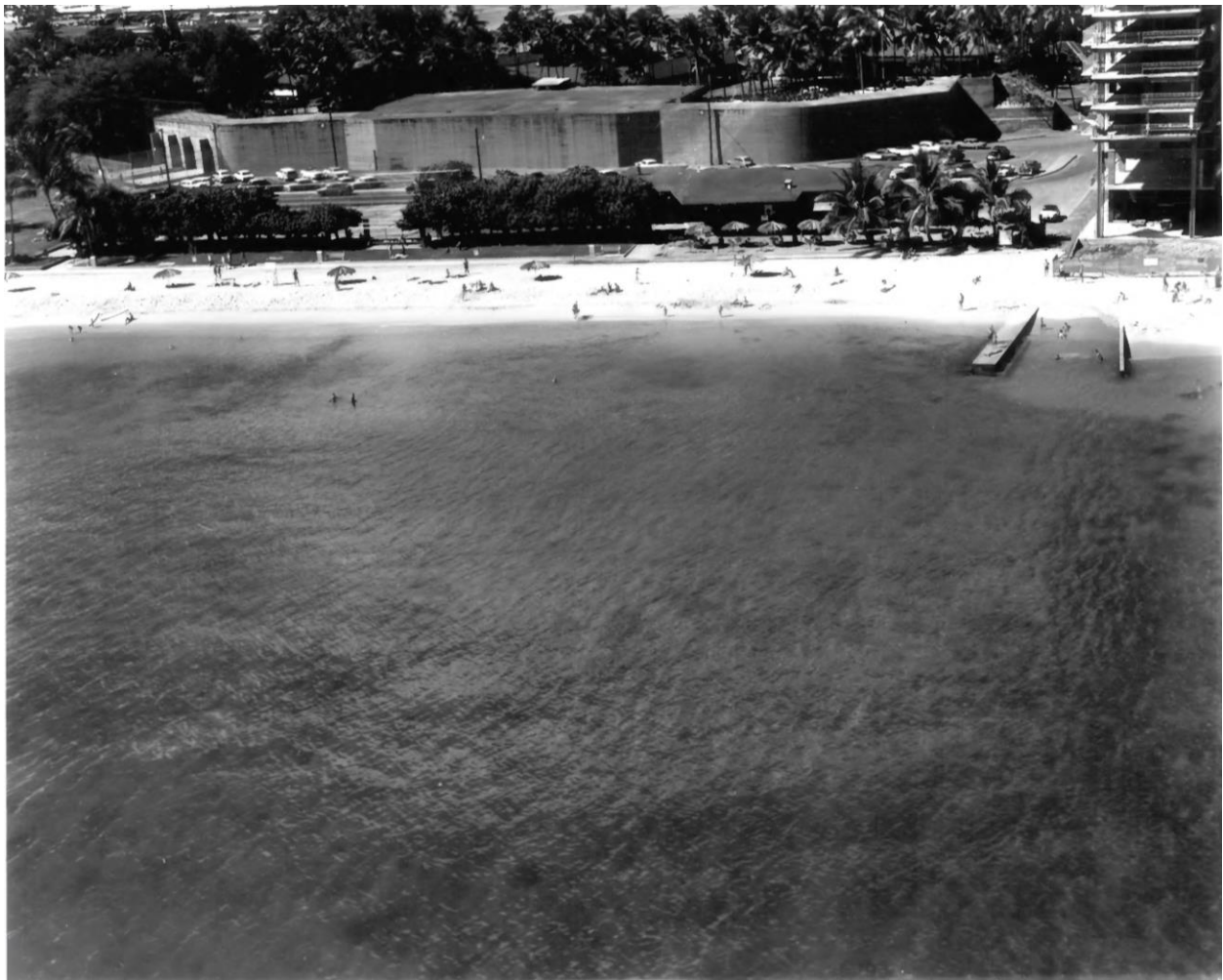
Photo 11. Battery Randolph from the ocean, 1961. U.S. Army Engineer District, Honolulu. Reproduced from the Artillery District of Honolulu (Site 1382) NRHP nomination (Char 1983).
