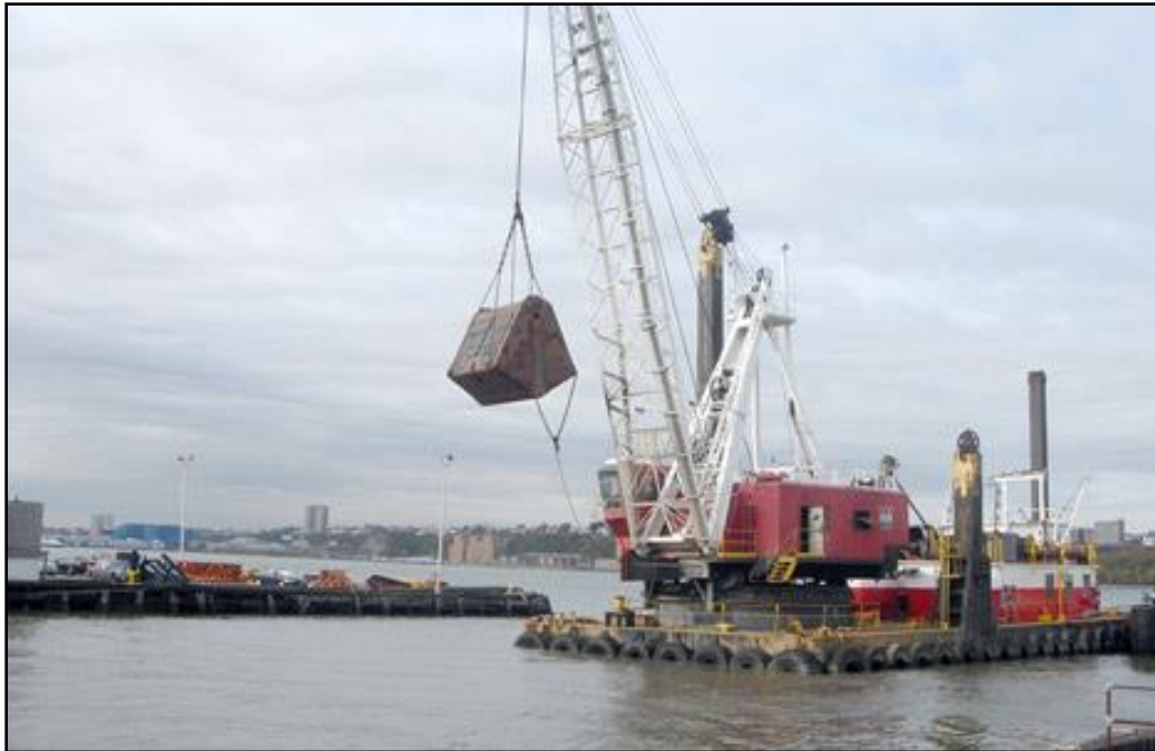
Figure 5-2 Example: Clamshell Dredge with Environmental Bucket ( http://www.conedison.com/ehs/2009annualreport/environmental_stewardship )
