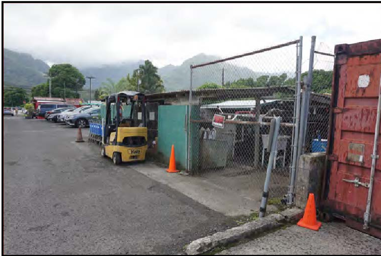
Photo 1: View of existing WWTP enclosure. Facing South. Property line ends at short concrete wall in lower right.
