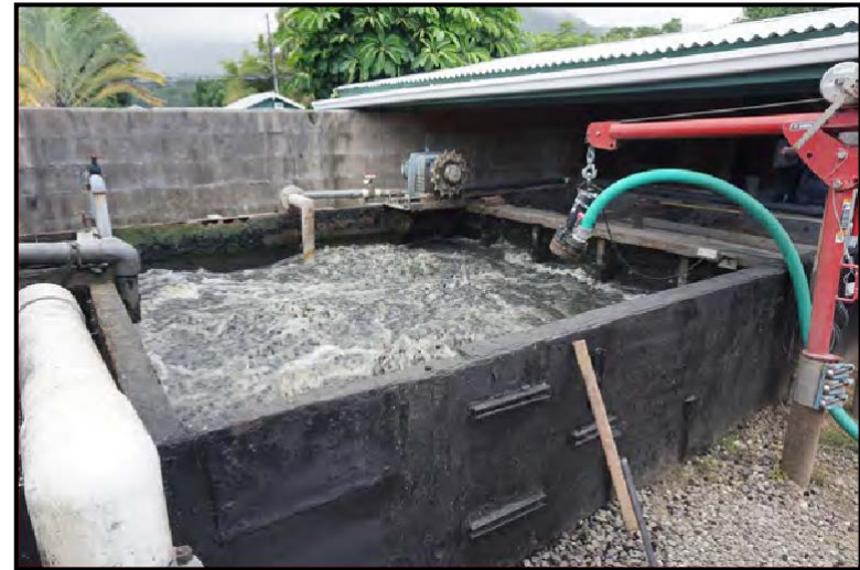
Photo10: Existing aeration tank within WWTP enclosure. Facing southeast.
