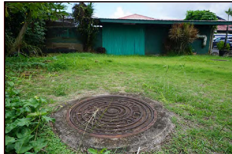
Photo 4: View of existing backup injection wells and existing WWTP enclosure. Facing east
