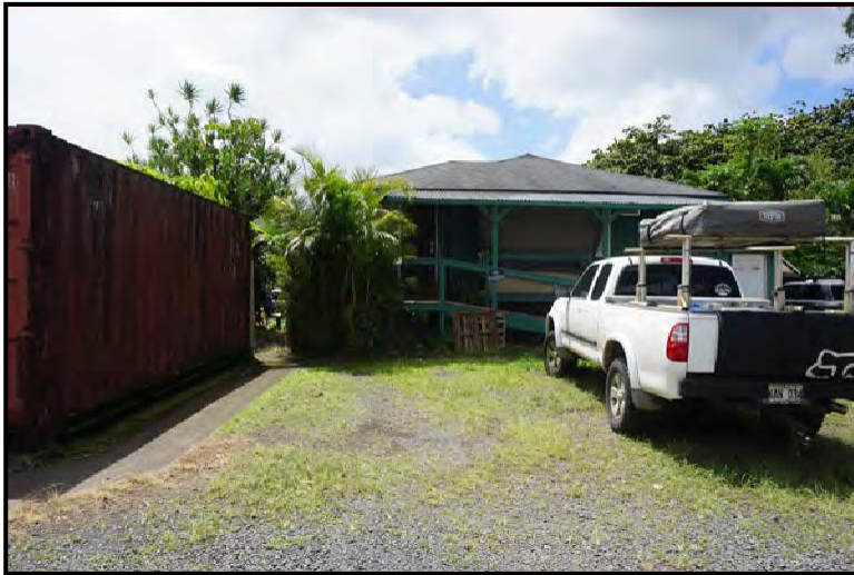
Photo 19: Building located on north side of existing WWTP. Facing west.
