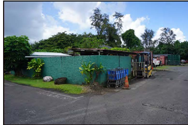
Photo 2: View of existing WWTP enclosure. Facing northwest.
