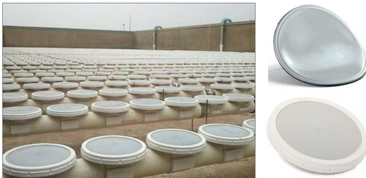
Figure 4: Example ECD Diffusers with PTFE Membranes
