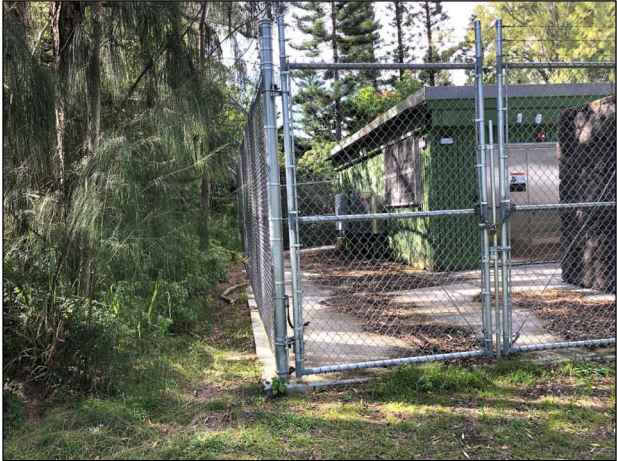
Figure 16. Southwest corner of Radio facility, looking NNW.
