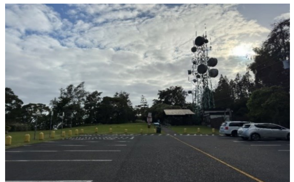
View of existing tower from parking lot facing makai
