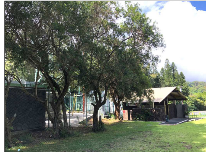
Figure 15. Looking NNE. Foreground is 1 st radio tower, second is behind the stone building which is the restrooms; the parking lot is visible beyond.
