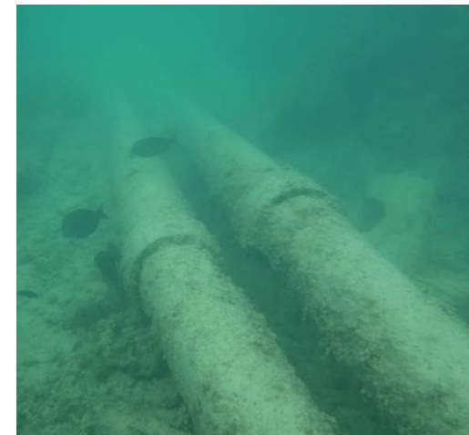
Photo 3. Typical view over the pipe intake channel, where pipe is exposed
