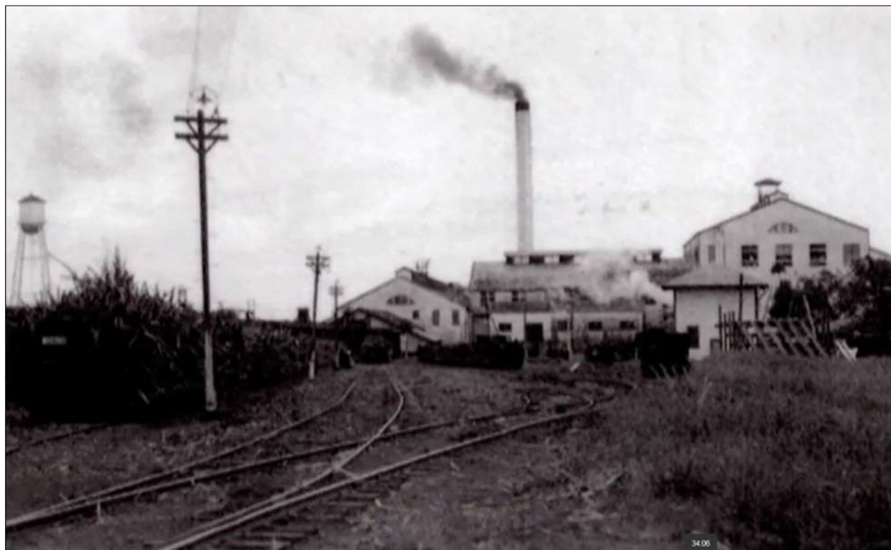
Figure 29. Hawai'i Consolidated Railway alignments at ‘Ōla‘a Sugar Mill.
