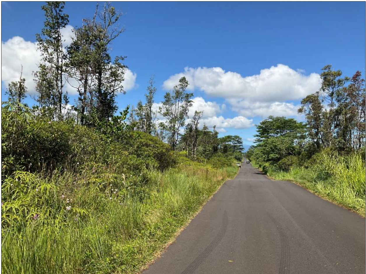
Figure 4. Makai (northeastern) boundary of project area (on right) along 25 th (‘Okika Avenue), view to the west-northwest.
