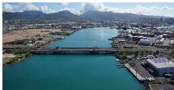
Sand Island Parkway provides the sole connection to mainland Oahu.
