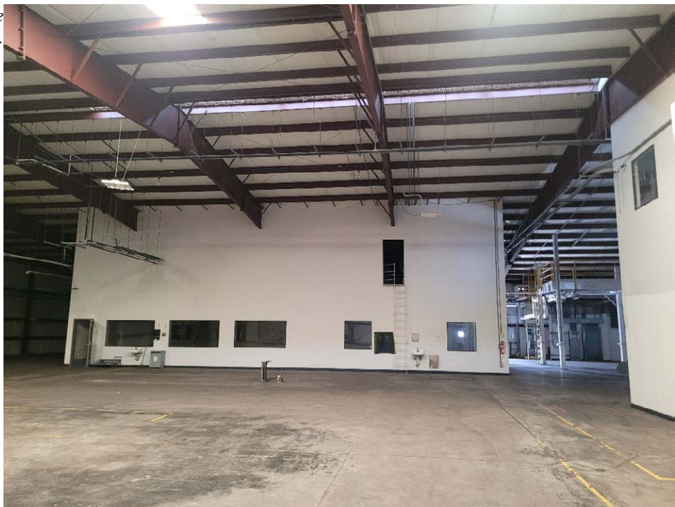
b. View of warehouse interior.
