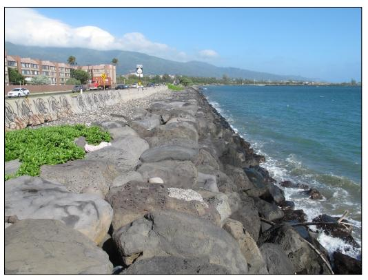
Figure 5-21 Rock rubblemound revetment at Kahului, Maui (2011)
