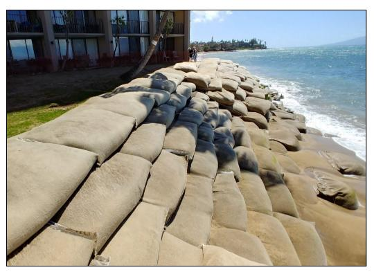
Figure 5-12 Geotextile sandbag revetment at Kahana, Maui (2018)
