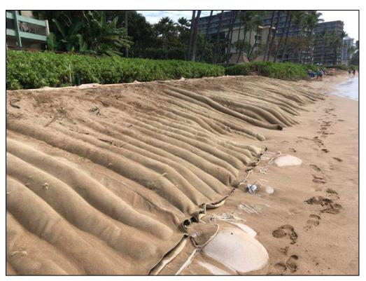
Figure 5-11 Geotextile sand filled mattress at Kaanapali, Maui (2018)
