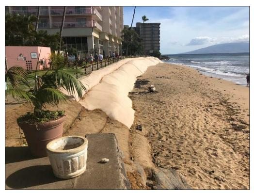
Figure 5-10 Geotextile erosion protection skirt at Honokowai, Maui (2018)
