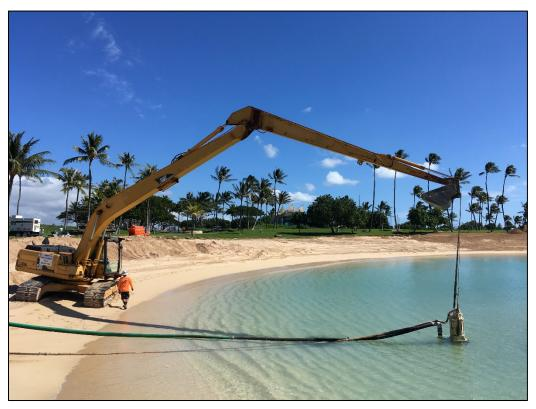
Figure 5-2 Sand pumping at Ko'olina, Oahu (2017)
