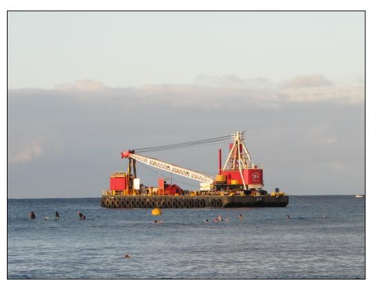
Figure 5-9 Offshore sand recovery at Waikiki Beach, Oahu (2012)
