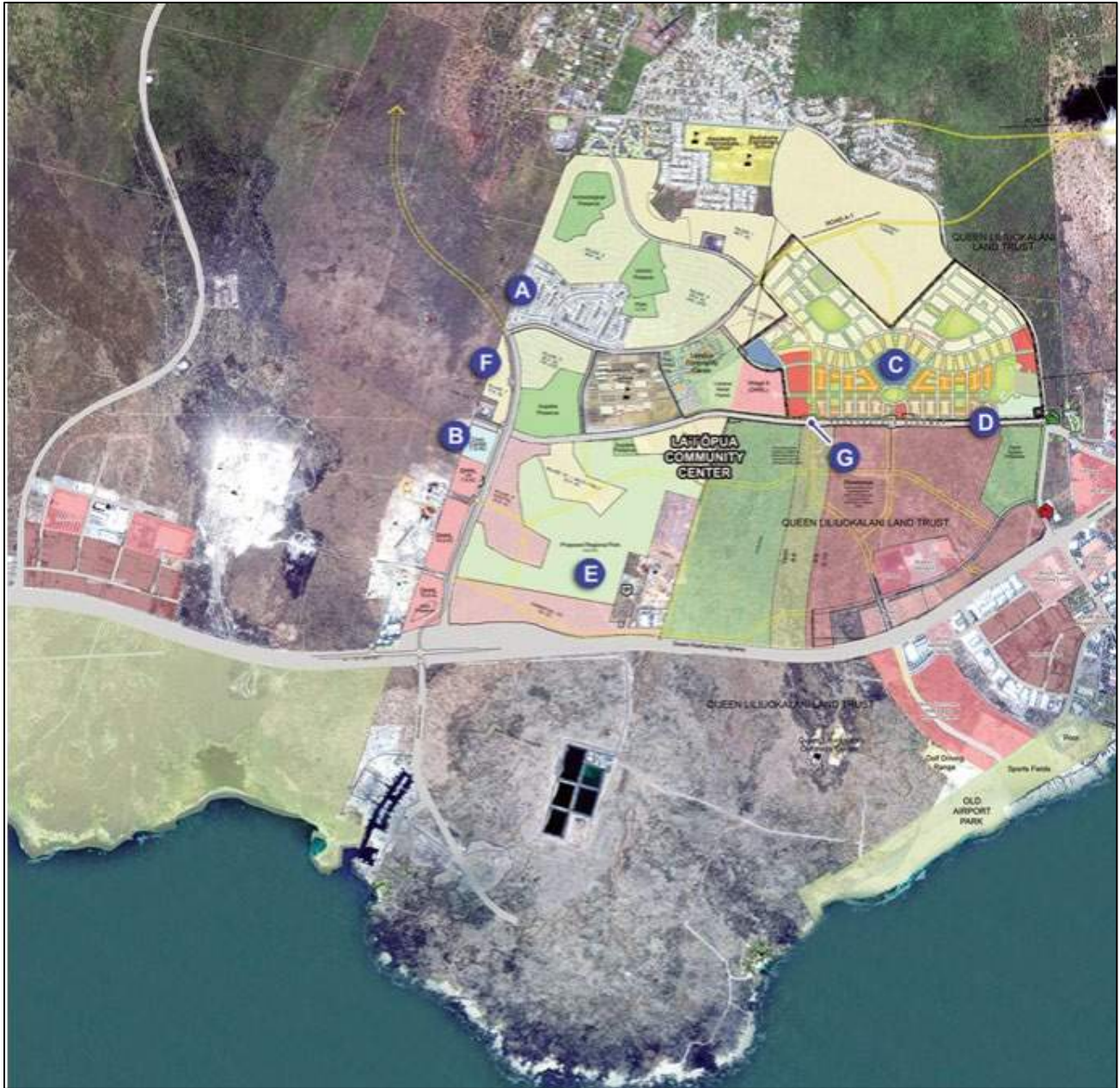
Figure 14. Overall view of the Villages of La'i 'Ōpua (La'i 'Ōpua n.d.)
