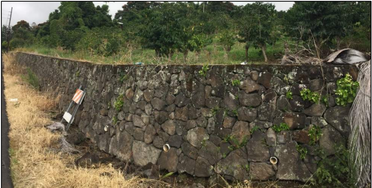
Figure 23. Photo showing the northern portion of the modern stone wall fronting the project area along Māmalahoa Highway; note PVC drainpipes along the base of the wall; view to north
