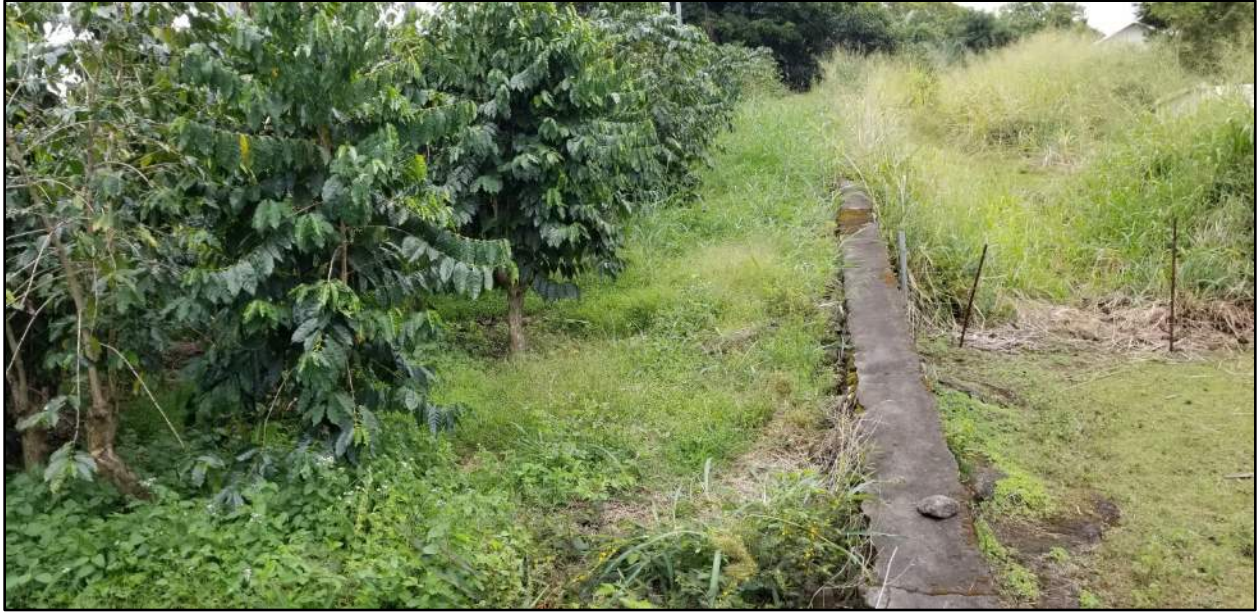
Figure 26. Photo looking mauka along the low, modern stone wall extension bounding the property to the south; view to east
