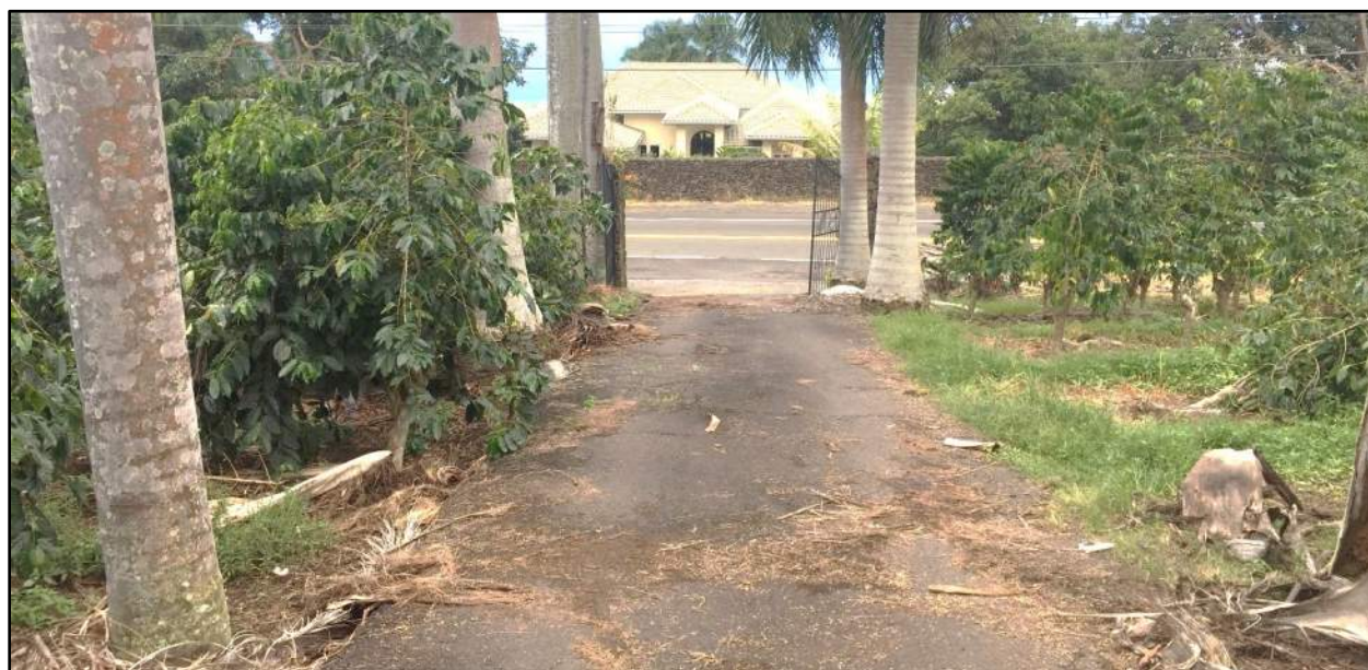
Figure 21. Photo looking down the modern asphalt driveway in the project area to its entry gate at Māmalahoa Highway; view to west
