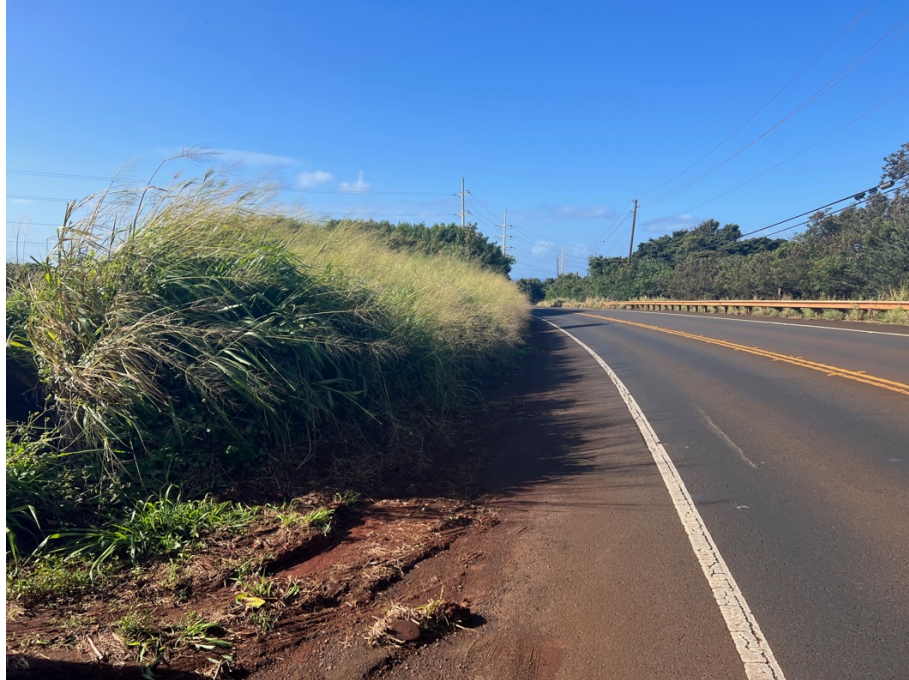
Figure 2. Kaumuali'i Highway on the right with Guinea grass hedgeline and access road opening to the PA.
