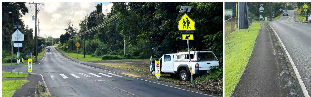
School Crosswalk (Left) and Sidewalk Cross-Section Adjacent to School Property (Right)
