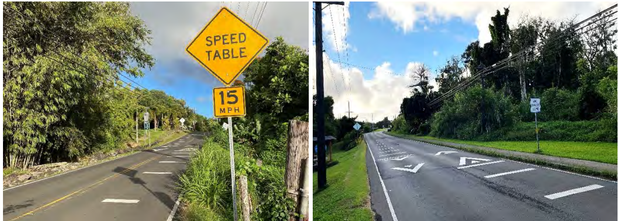
North Driveway Speed Table (Left) and South Driveway Speed Table (Right)
