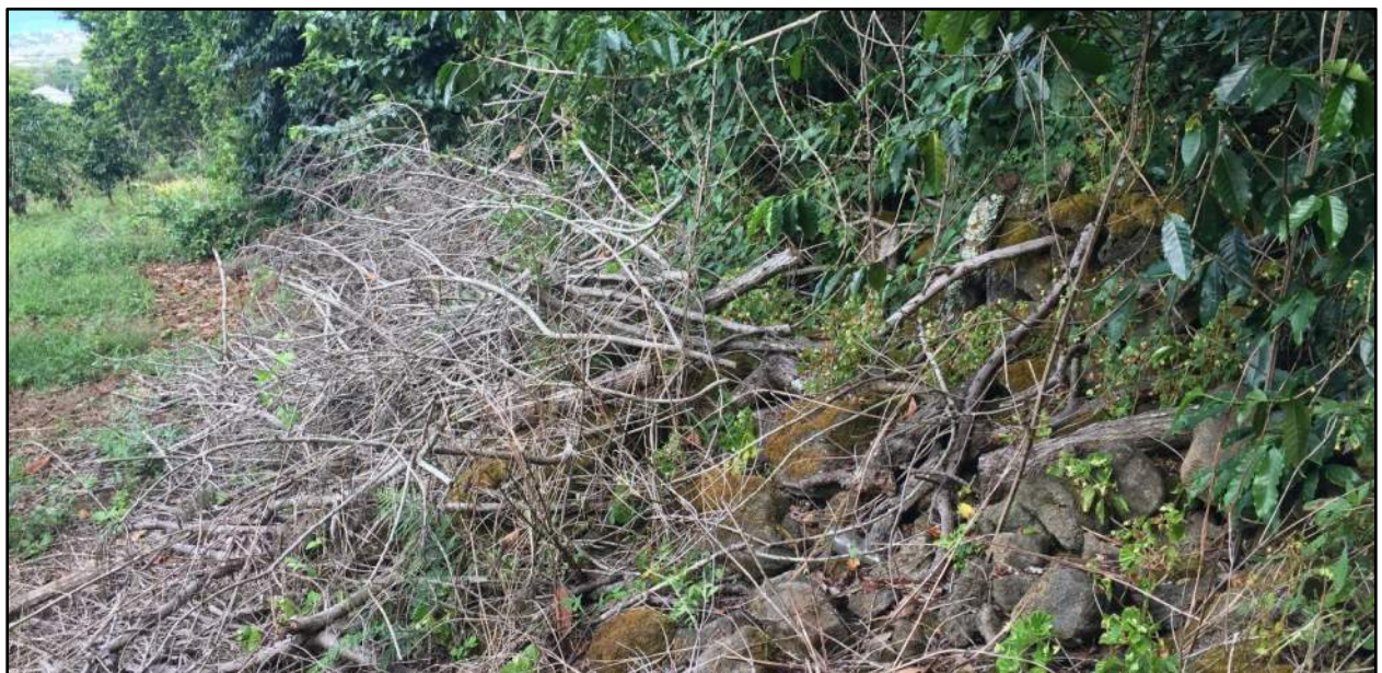
Figure 24. Photo showing rock material and debris pushed up against the wall located just outside the project area to the north; view to west
