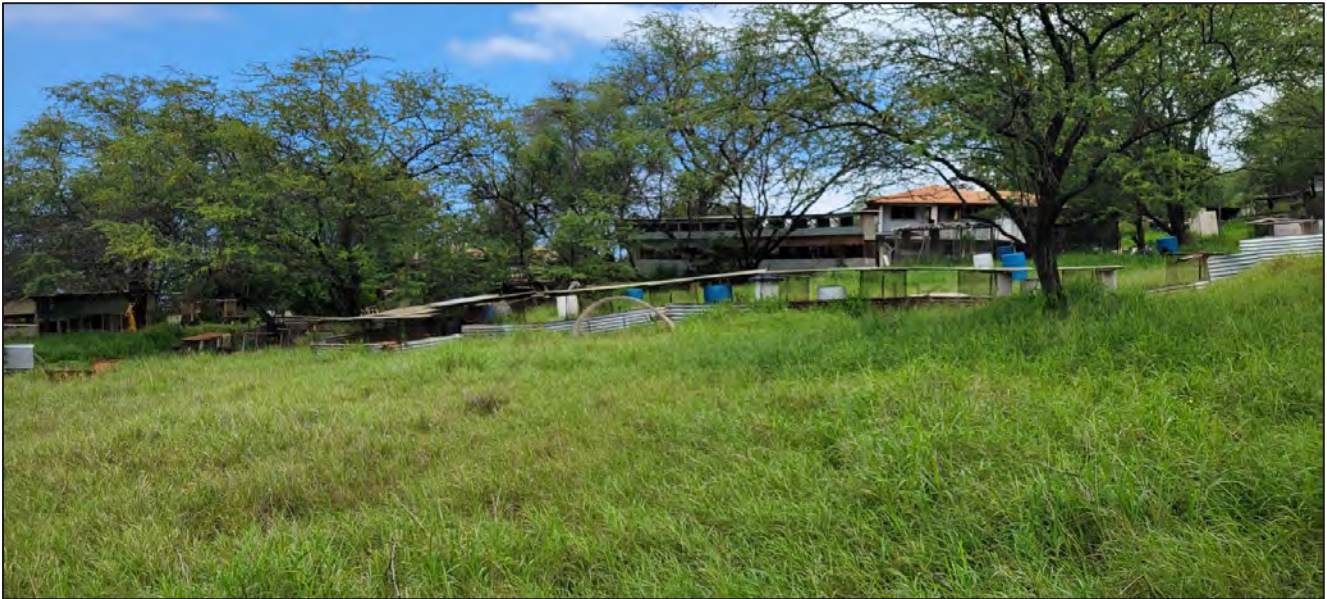
FIGURE 8. OVERVIEW OF ENCROACHMENT IN THE DIRECT APE, FACING WEST.
