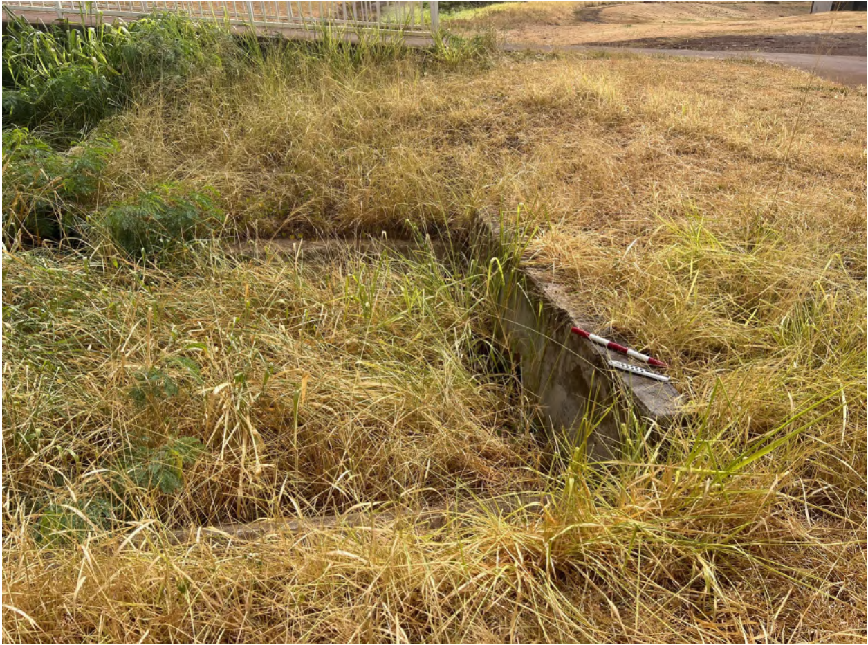
Photo 4 – Concrete culvert head wall facing northeast
