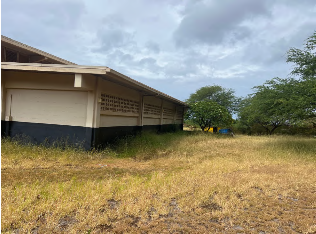
Photo 13 – Kitchen building facing south
