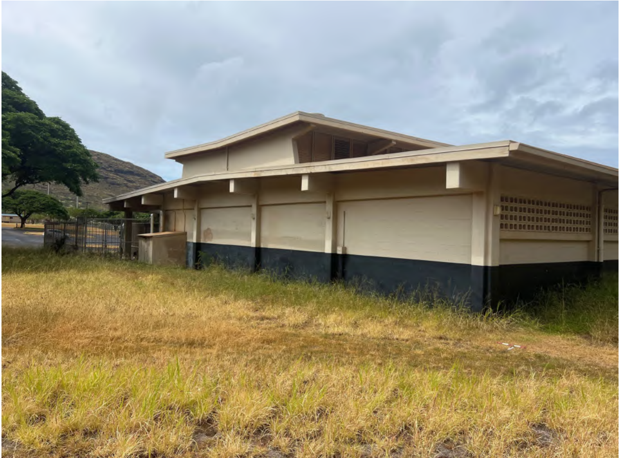
Photo 12 – Kitchen building facing southwest
