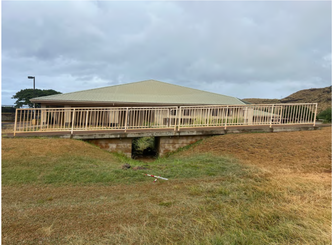
Photo 2 – Culvert and foot bridge facing northwest
