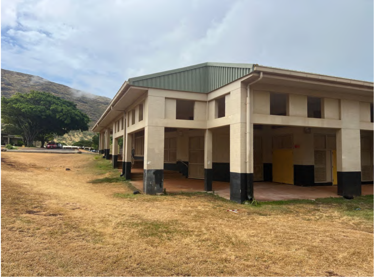
Photo 7 – Performance arts building facing south
