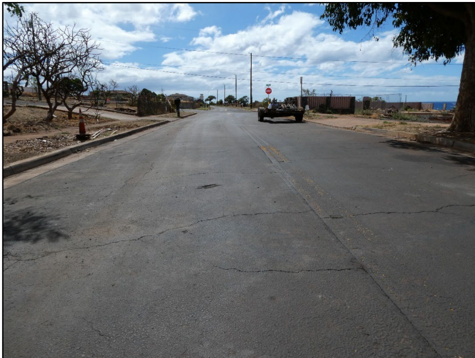
Figure B-2. View south along Aa Street from northern APE boundary.
