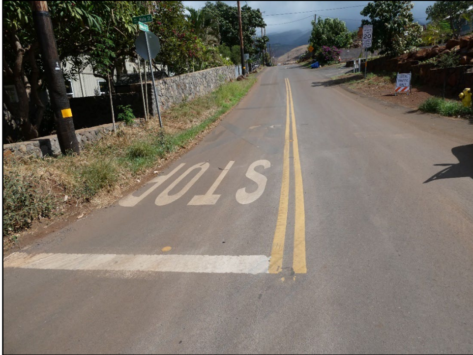
Figure B-13. View east along Wahikuli Road from Malo Street at western APE boundary.
