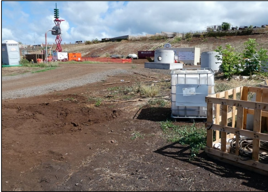
Figure 24. Equipment and materials storage behind the Lahaina 3 Pump Station building, view to the northeast.
