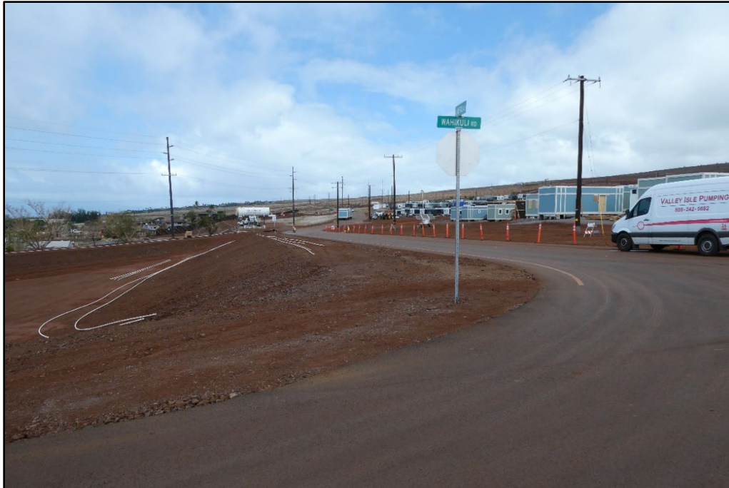
Figure 22. Newly identified segment of SIHP Site 50-50-03-08886 (railroad), adjacent to the APE (lined with delineators), photographed from the eastern APE boundary at Wahikuli Road, view to the northeast.
