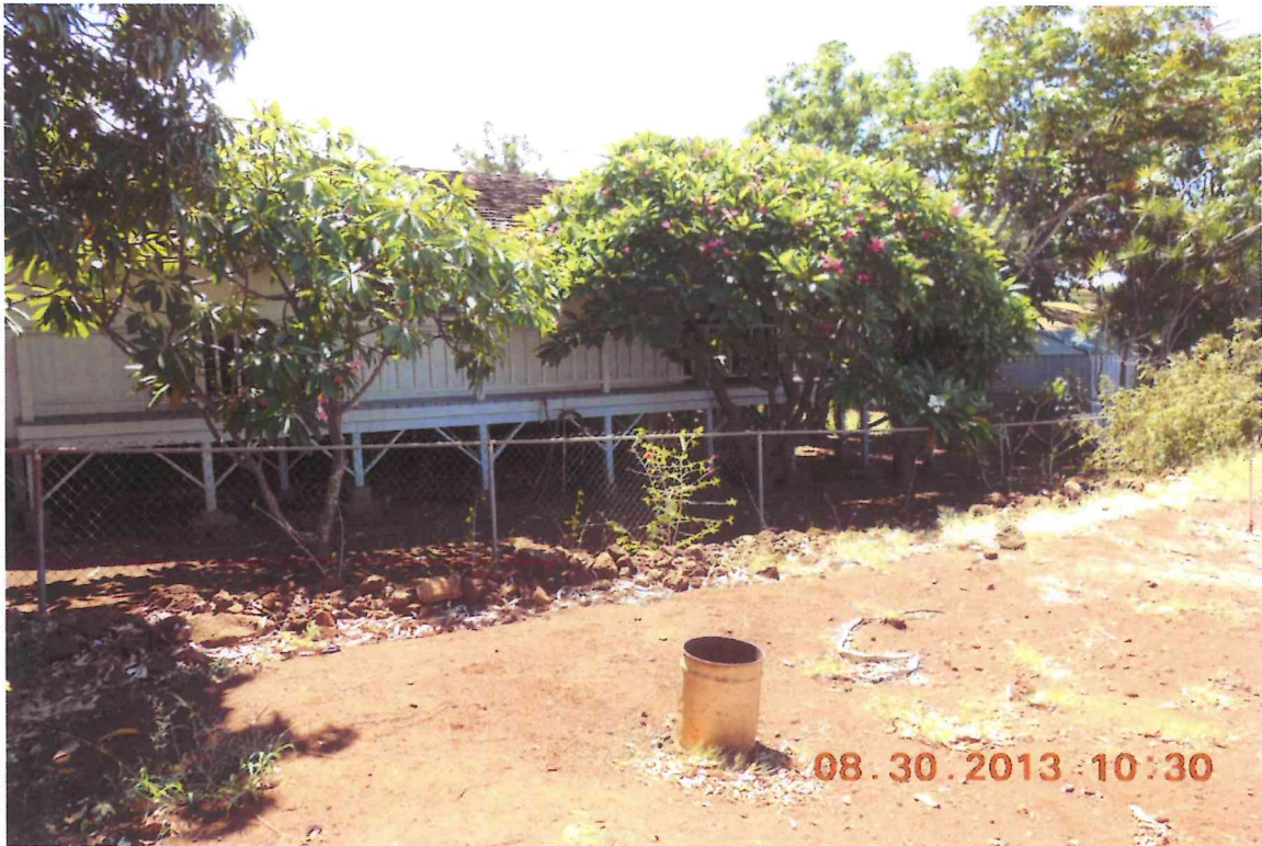
Photo No. 57 Facing east between TMK 4-5-27:38 and 24
