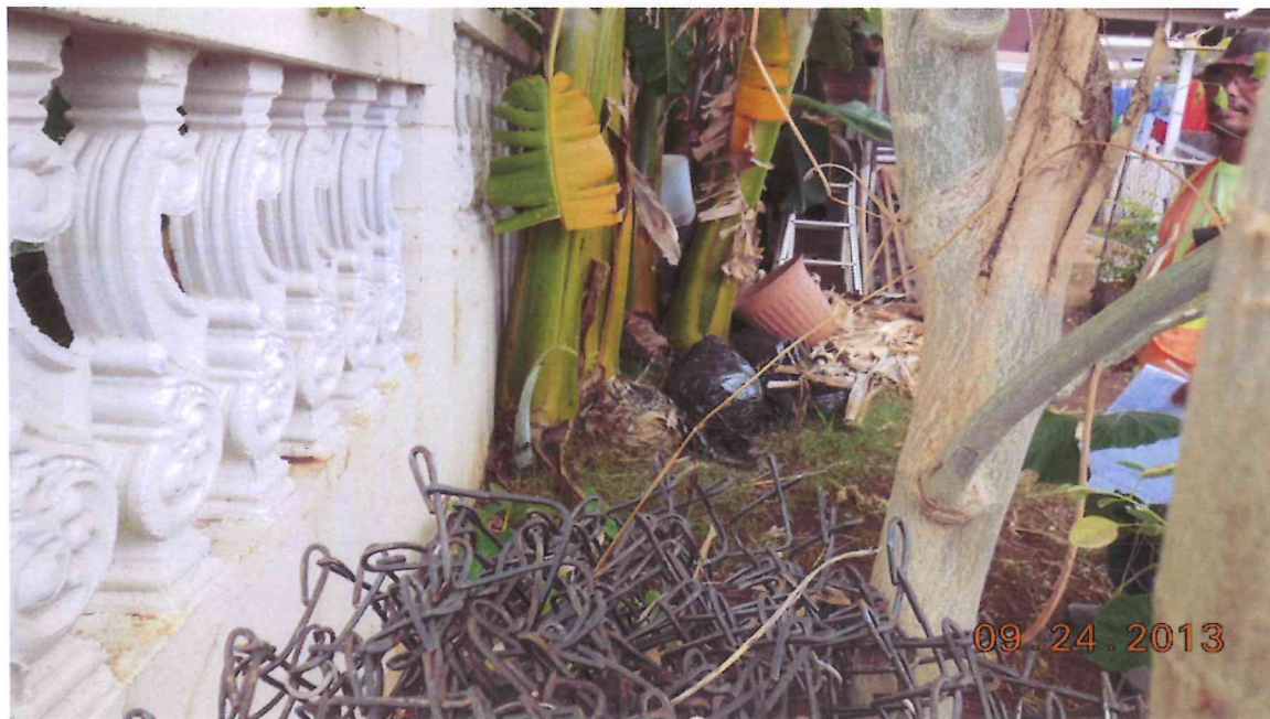
Photo No. 24 Facing east between TMK 4-5-28:61 and 60
