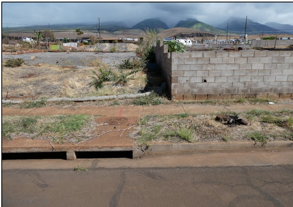
Figure B-20. Proposed sewer line easement trending east from Aa Street (in foreground) between Kaniau Road and Malanai Street, view to the east.
