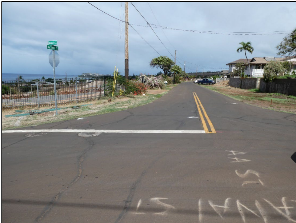
Figure B-8. View north along Aa Street from Malanai Street within the APE.
