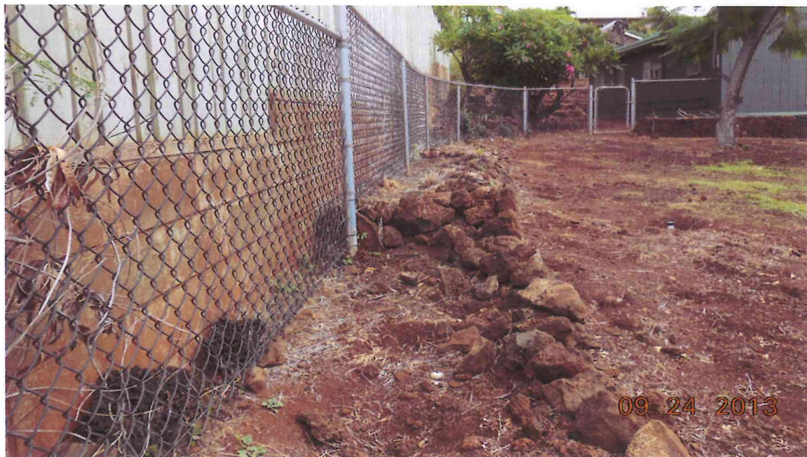
Photo No. 48 Facing east between TMK 4-5-28:5 and 6
