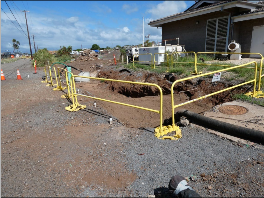
Figure 26. Open exposure near the Lahaina 3 Pump Station, view to the north.
