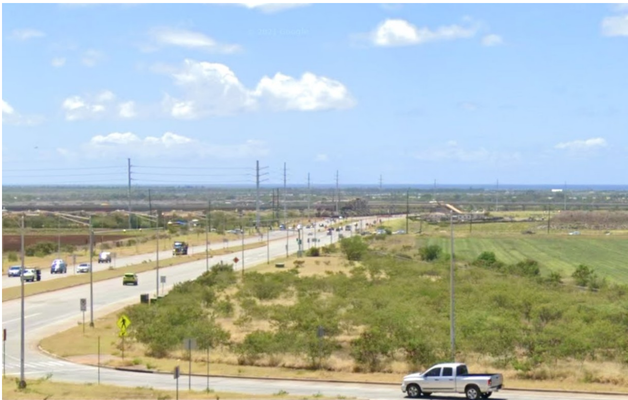
Figure 3-3: View toward the Project Site from H-1 near Kualakai Parkway
