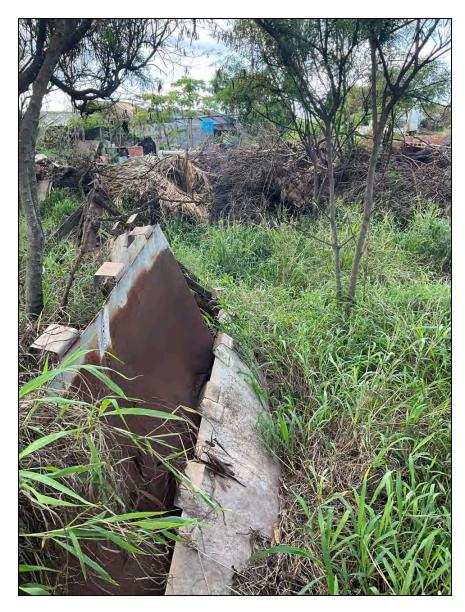
**Photo 16.** Flume in disrepair at NHD-identified Ditch 1 location showing where the ditch previously crossed the western branch of Kalo'i Gulch. Date: 02/04/2025.
